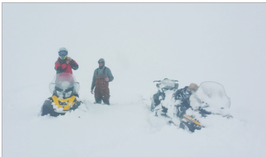
Figure 4. The technician team pauses to discuss travel to the next site during generator servicing in light snow on 15 December 2016. (WMI photograph by Michael Paul.)
