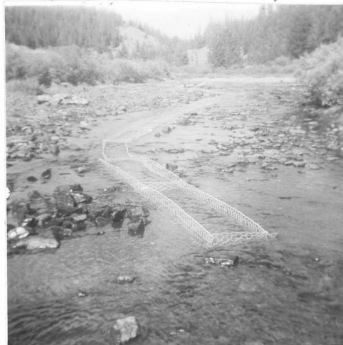
Barrier during construction, 5 cfs
