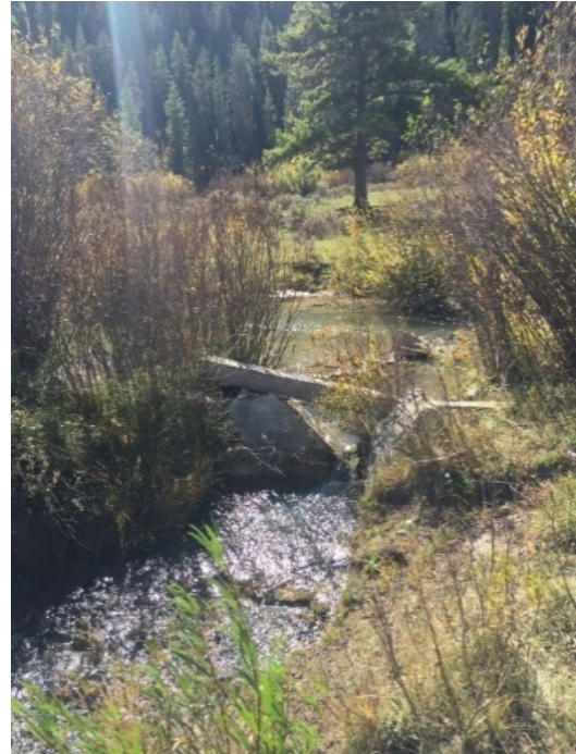
Photo 27 Fall Creek Diversion Structure
