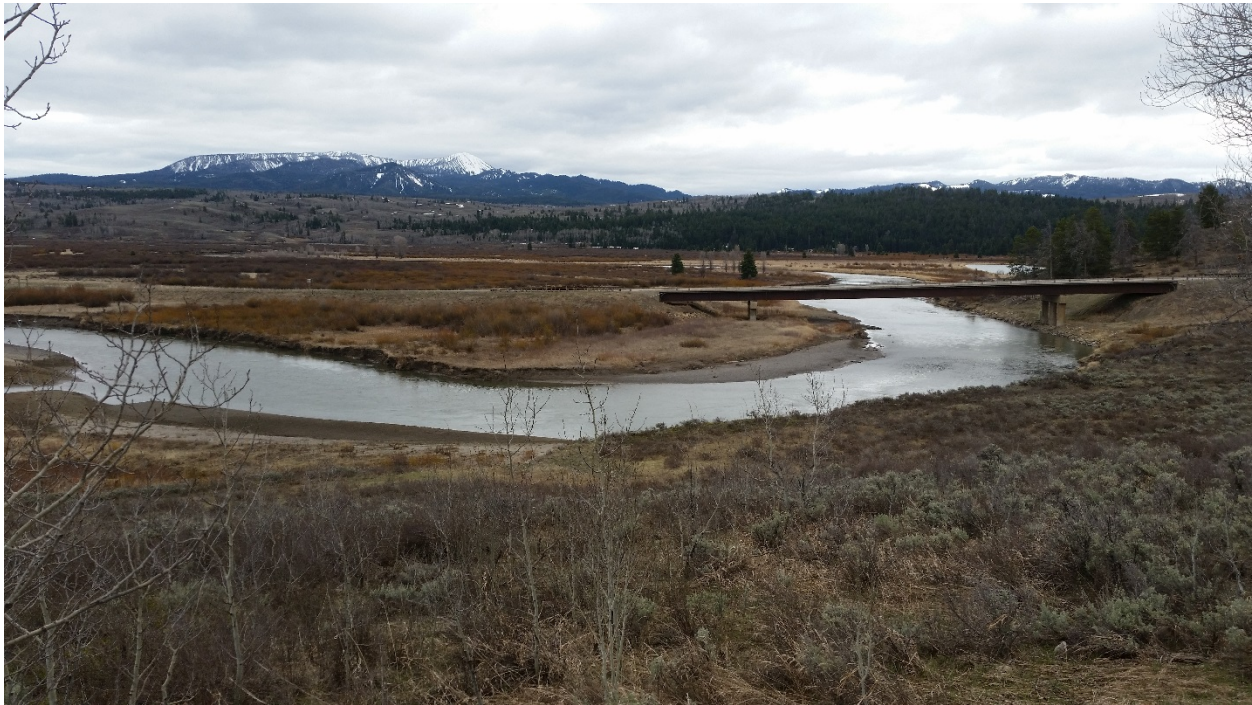
Photo 10 Buffalo Fork Looking Downstream at the Highway 191 Bridge
