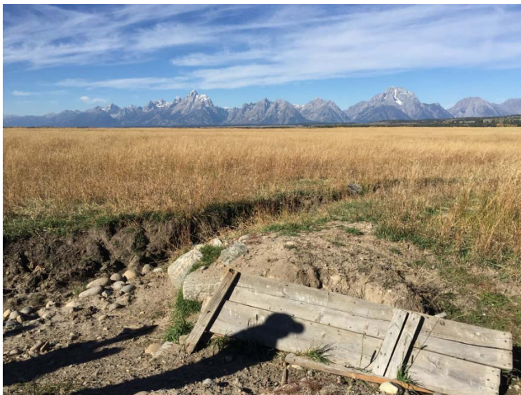
Photo 17 Elk Ranch Flood Irrigation Ditch and Diversions
