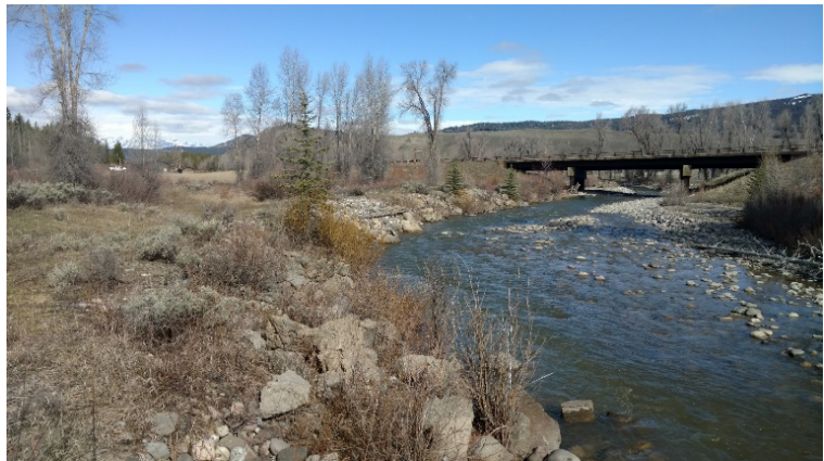
Photo 16 Blackrock Creek and Levee
