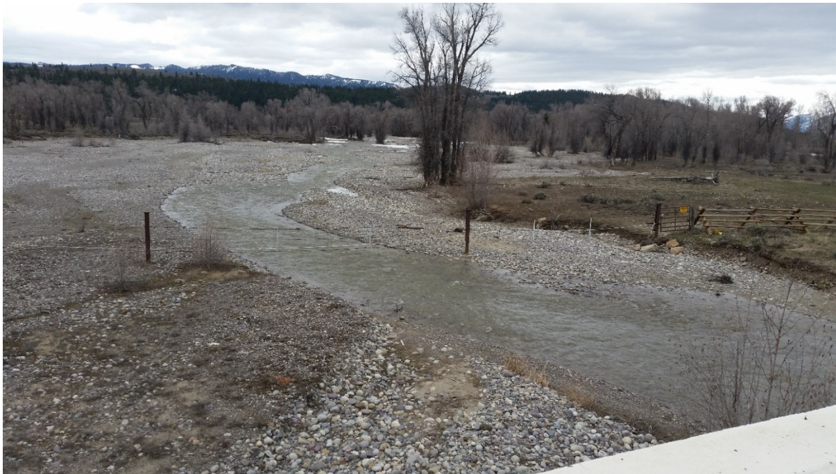
Photo 9 Lava Creek Looking Downstream from the Bridge on Highway 191
