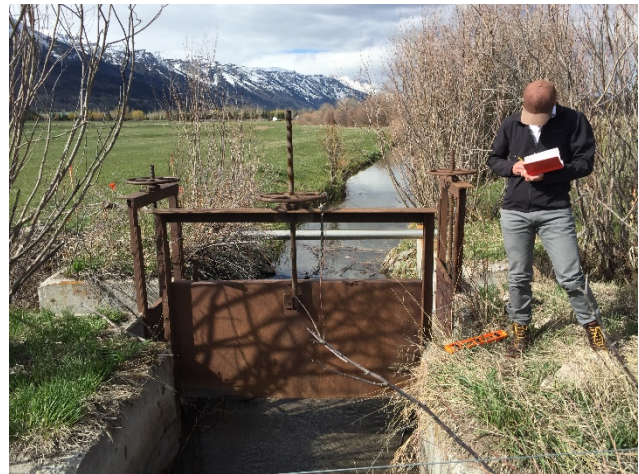
Photo 24 Three-way Headgate, Prosperity Ditch at Highway 22
