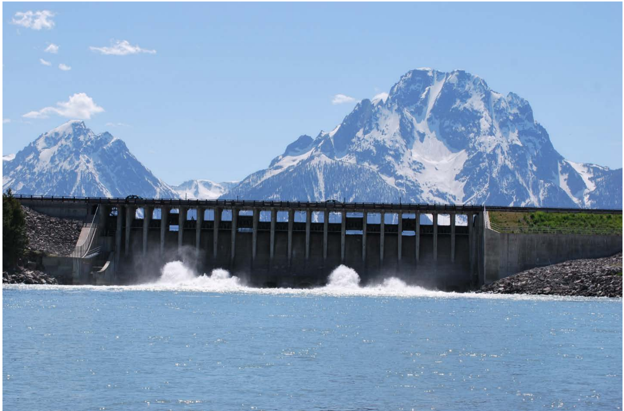
Photo 3 Jackson Lake Dam at Grand Teton National Park
