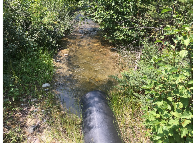
Photo 19 Terminus of Pipeline for Antler Ditch
