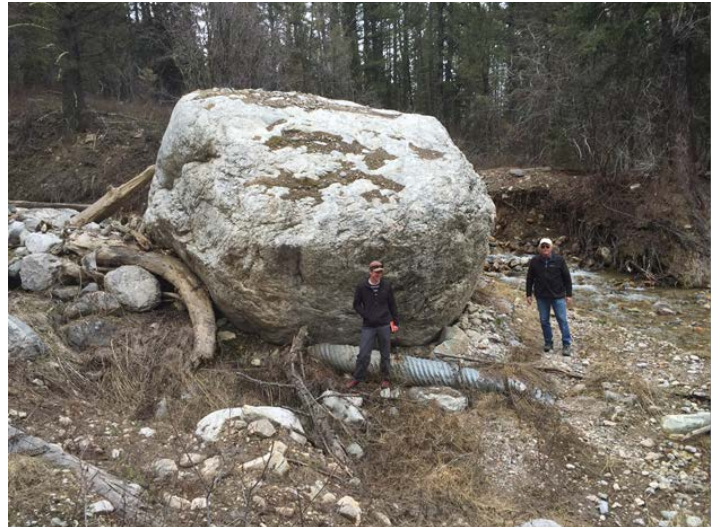
Photo 23 Jensen Creek Diversion Structure Crushed by a Boulder During a Debris Flow.
