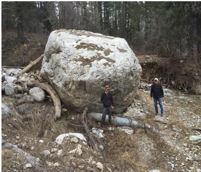
Example of an irrigation system improvement needs in the Upper Snake River Watershed where a Jensen Creek diversion structure was crushed by a boulder during a debris flow. The replacement structure is proposed as Project Number #ISI-10.
