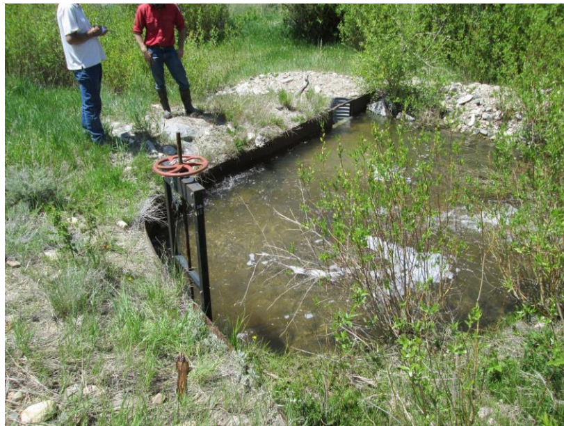
Figure 4.4-15 Example of a Cost-Effective Irrigation Diversion Structure.
