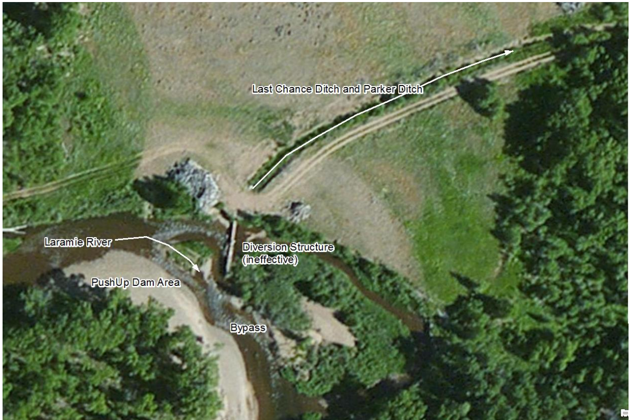
Figure 4.4-8 Combined Last Chance Ditch and Parker Ditch Diversion Facility.
