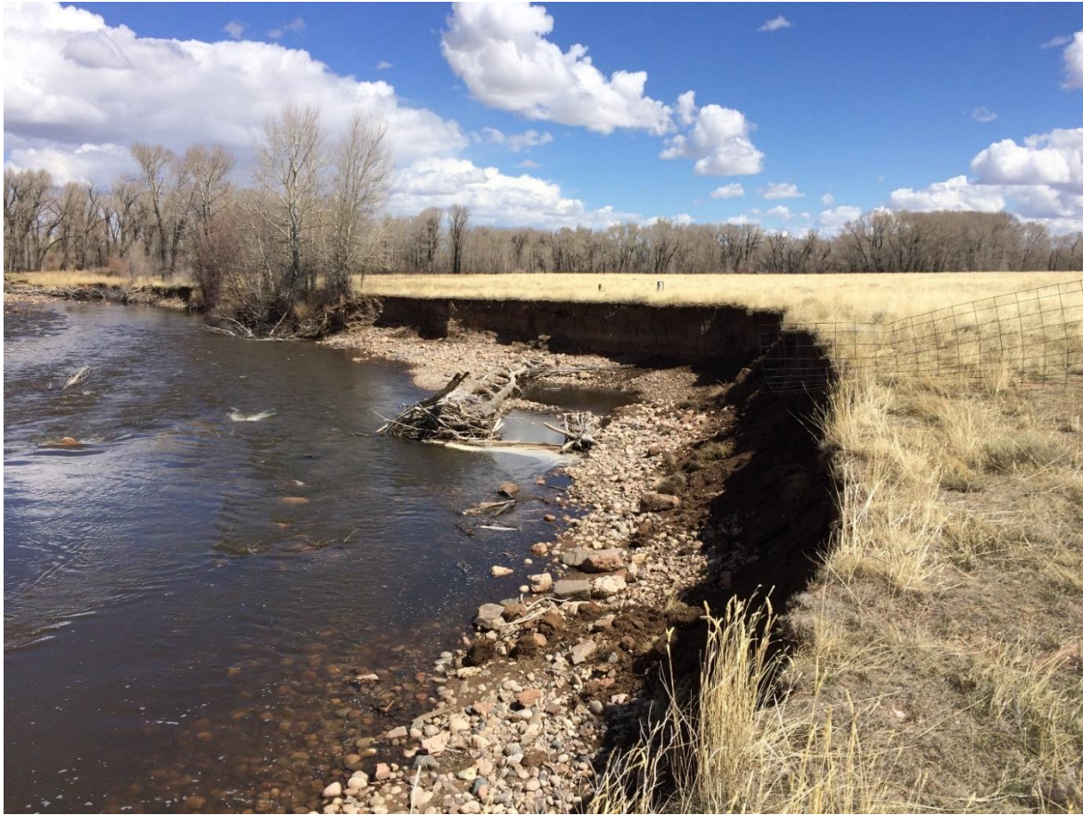
Figure 3.6-10 Bank Erosion on the Laramie River Downstream of Woods Landing.
