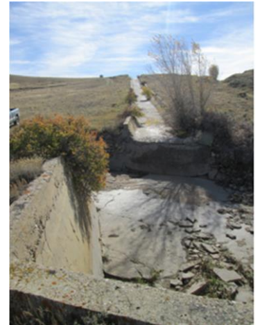
Figure 4.4-5. Bellamy Ditch Drop Chute Structure Looking Upstream from Outlet.
