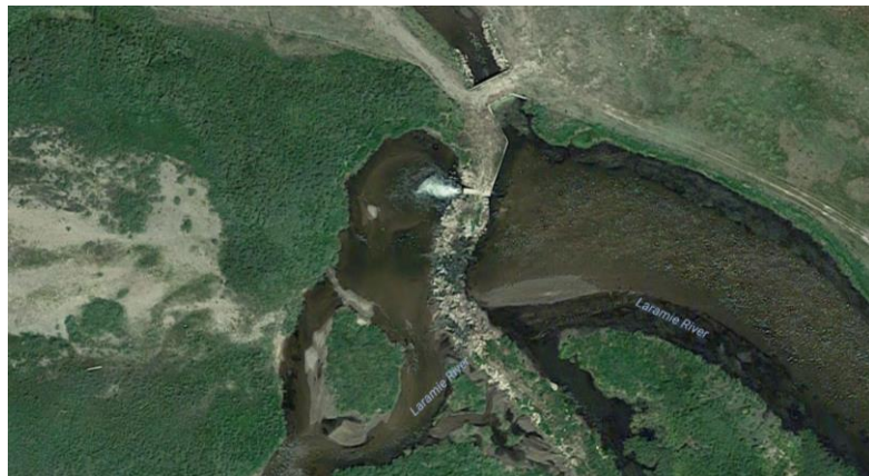
Figure 4.4-17. Oasis Ditch Diversion and Headgate Overview.
