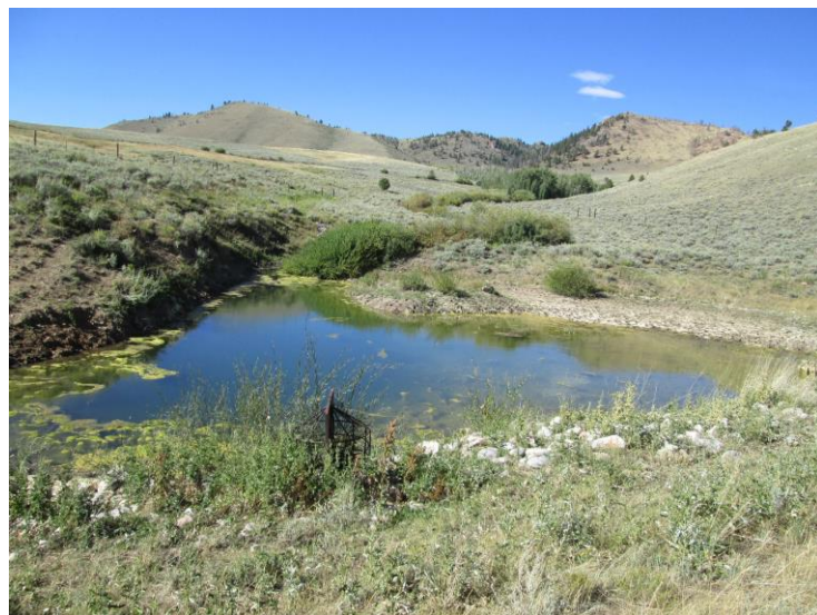
Figure 4.4-38 Existing Stock Reservoir in need of Rehabilitation.
