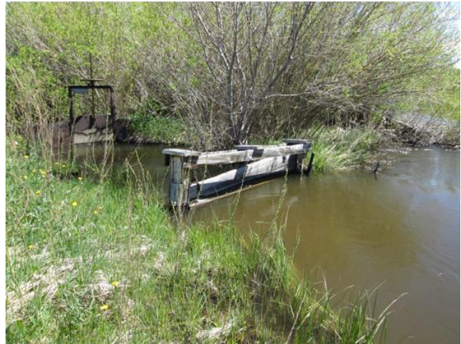
Figure 4.4-24. Hatton No. 1 Ditch Headgate.
