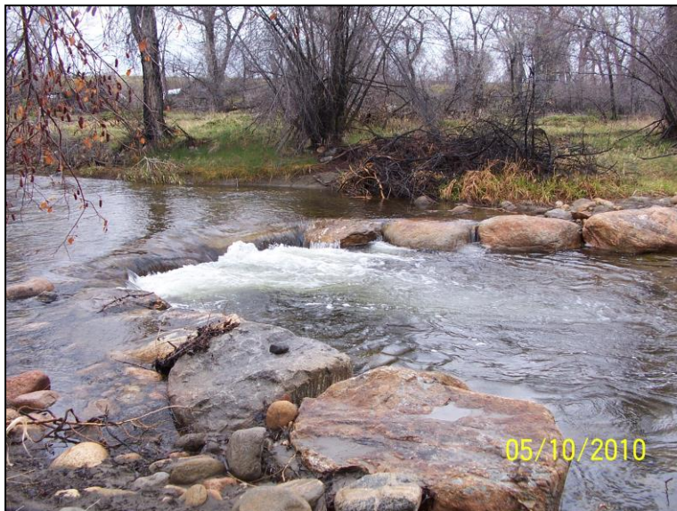
Figure 4.4-52 Stream Stabilization Structure: Rock Vortex Weir.
