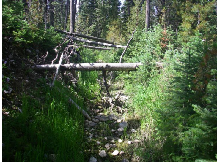
Figure 4.4-27 Typical Ditch Originating on Forest Lands Displaying Significant Deadfall.
