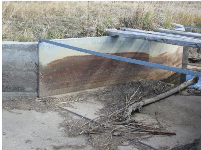
Figure 4.4-20. Existing Parshall Flume on the Oasis Ditch.
