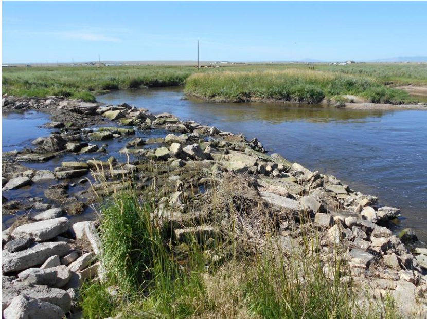
Figure 4.4-16 Oasis Ditch Diversion Structure on the Laramie River.
