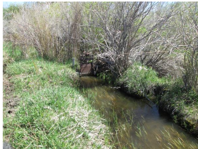
Figure 4.4-22 Hatton No. 2 Ditch Headgate. There is currently no diversion structure on the Hatton Ditch (Hatton Ditch is visible through vegetation on right side of photo).
