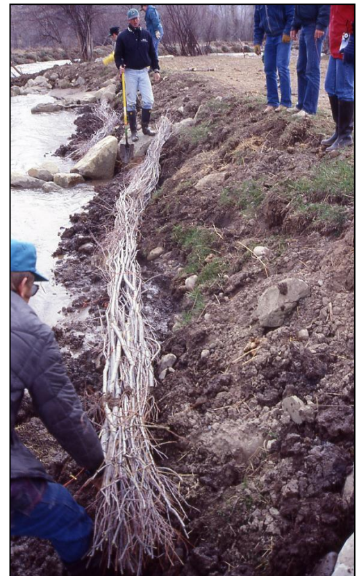
Figure 4.4-54 Stream Stabilization Measure: Willow Fascine Installation.
