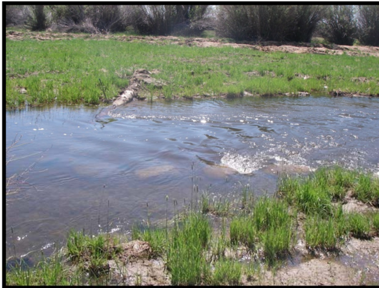
Instream treatment example: hybrid rock/log vane.
