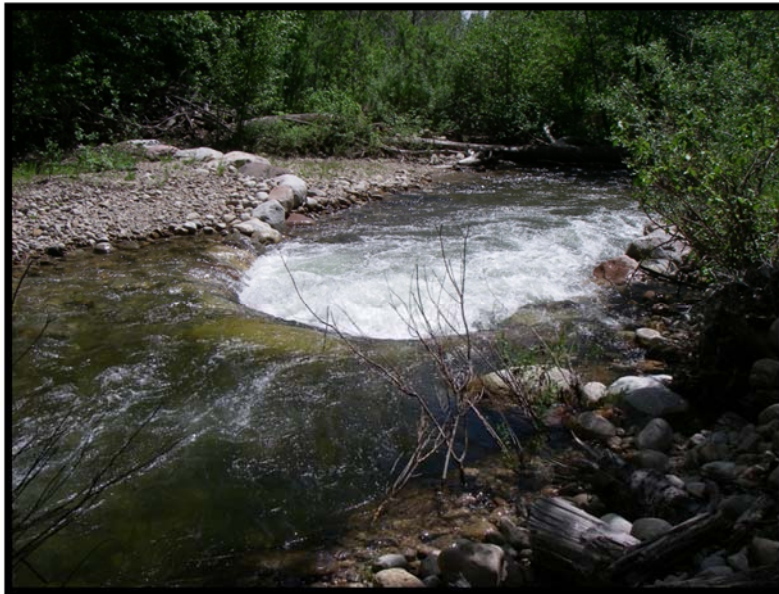
Instream treatment example: rock cross vane.
