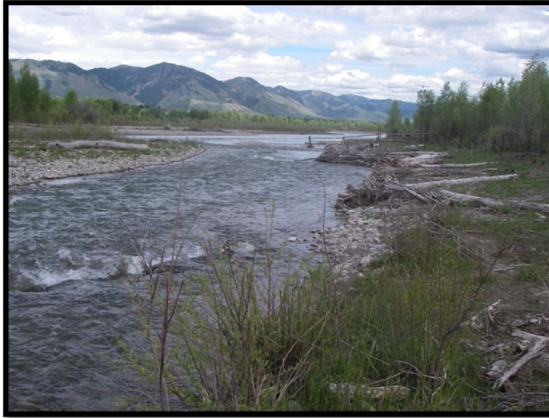
Instream treatment example: root wad revetment and rock barb.
