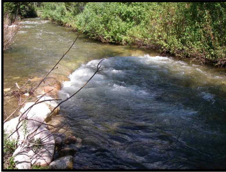
Instream treatment example: rock J-hook vane.
