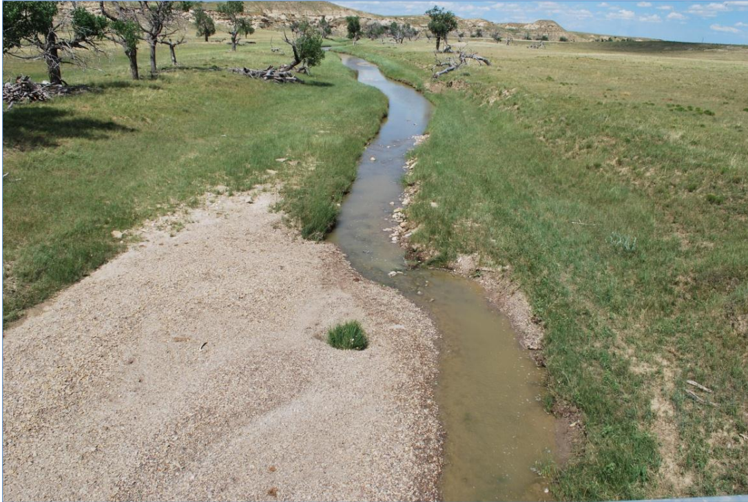
Photo 3 - Lightning Creek from bridge after significant runoff event. Sediment deposit on bank.
