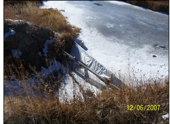
Figure 2.33 J.M. Brown Ditch (East) Diversion on Lower Long Creek.
