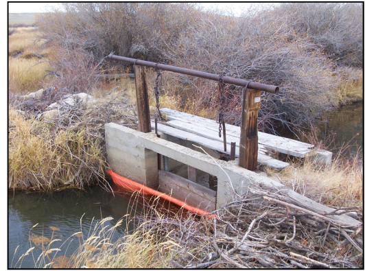
Figure 2.34 Russell Ditch Headgate.
