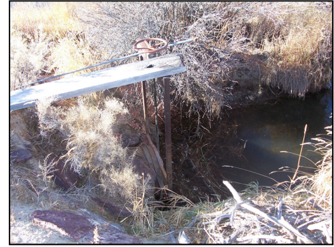
Figure 2.38 Koehler Ditch Headgate.
