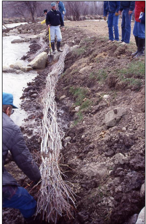
Figure 3.3 Stream Stabilization Measure: Willow Fascine Installation.
