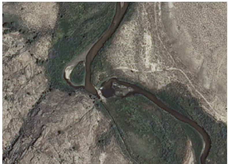
Figure 2.34 Overview of the McIntosh Ditch Diversion Structure.
