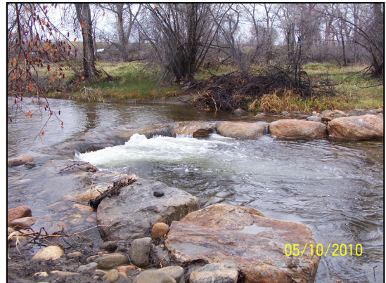
Figure 3.2 Stream Stabilization Structure: Rock Vortex Weir.
