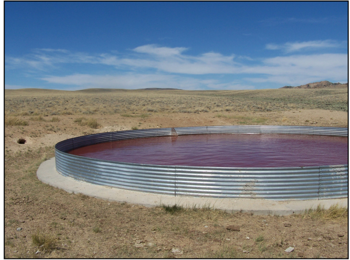
Figure 2.30 30-Foot Diameter Concrete Bottomless Stock Tank.
