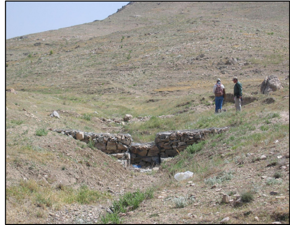
Figure 3.5 Stream Stabilization Structure: Rock Filled Gabion.
