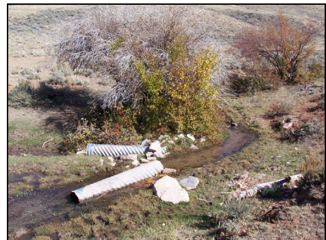
Figure 2.30 Hays Ditch Diversion on Whiskey Creek.
