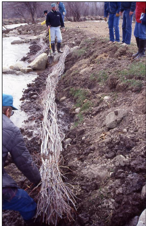
Figure 3.6 Stream Stabilization Measure: Willow Fascine Installation.
