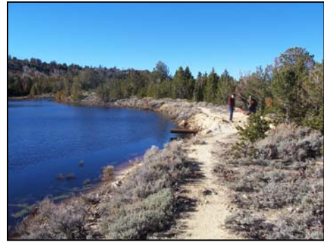
Figure 3.11 Woods Gulch Pond Reservoir Embankment and Outlet.
