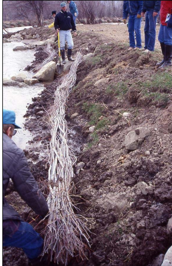
Figure 3.3 Stream Stabilization Measure: Willow Fascine Installation.
