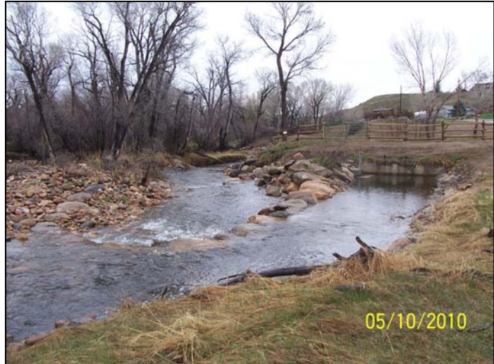
Figure 3.5 Rock Vortex Weir Installed to Facilitate Diversion of Irrigation Water.
