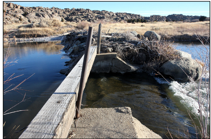
Figure 2.33 Point of Rocks / Emigrant Road Diversion Structure on the Sweetwater River.
