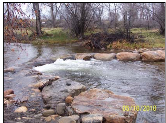
Figure 3.2 Stream Stabilization Structure: Rock Vortex Weir.
