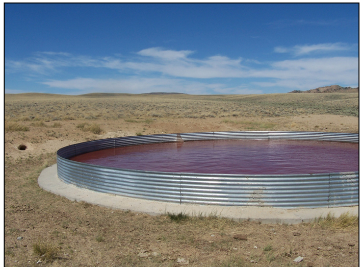
Figure 2.29 30-Foot Diameter Concrete Bottomless Stock Tank.
