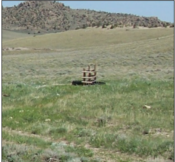
Figure 2.30 Undersized Livestock / Wildlife Watering Tank.
