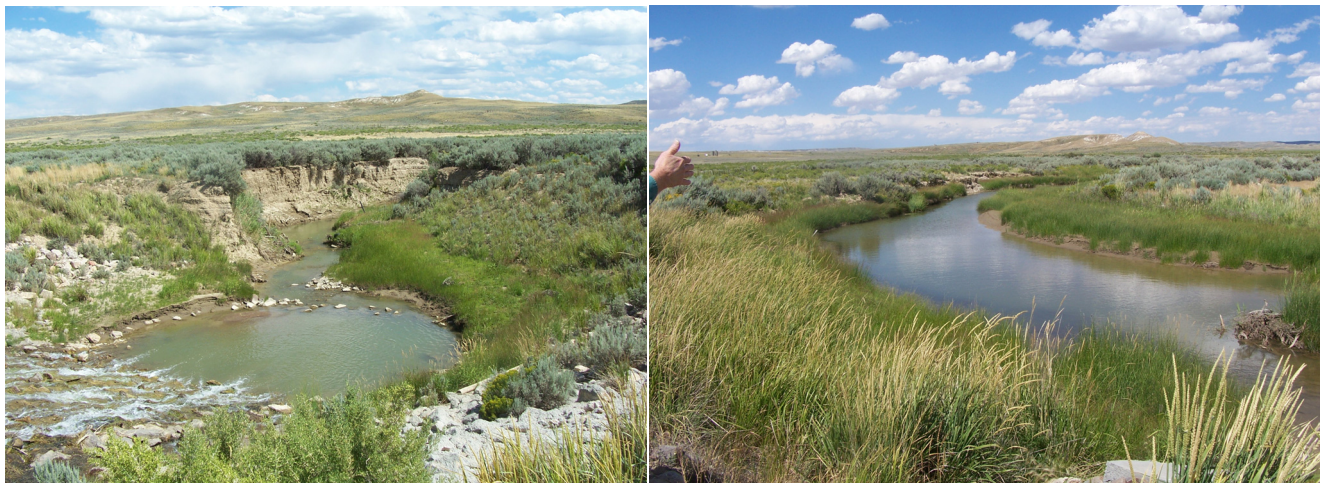
Figure 4.7 Channel Gradient Restoration Feature on Muddy Creek near Baggs, WY. Photo on left is viewed downstream from the dam at incised channel. Photo on the right is viewed upstream at restored gradient.
