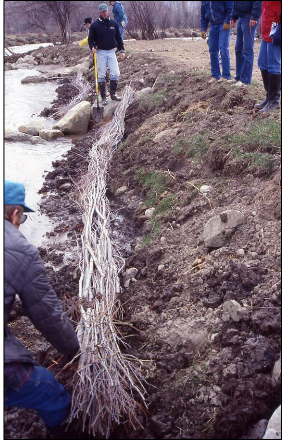
Figure 4.8 Stream Stabilization Measure: Willow Fascine Installation.
