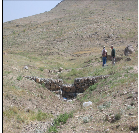
Figure 4.6 Stream Stabilization Structure.
