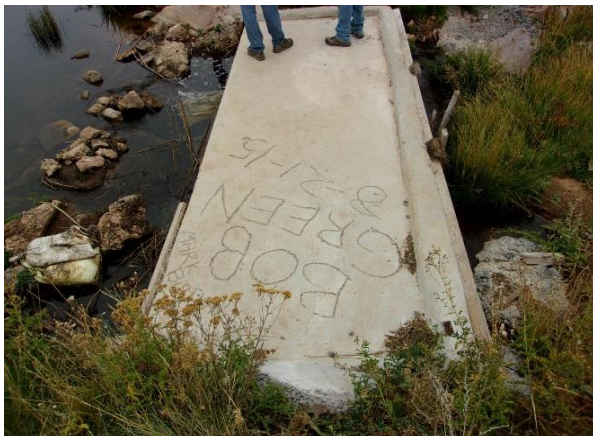
Concrete crest at emergency spillway
