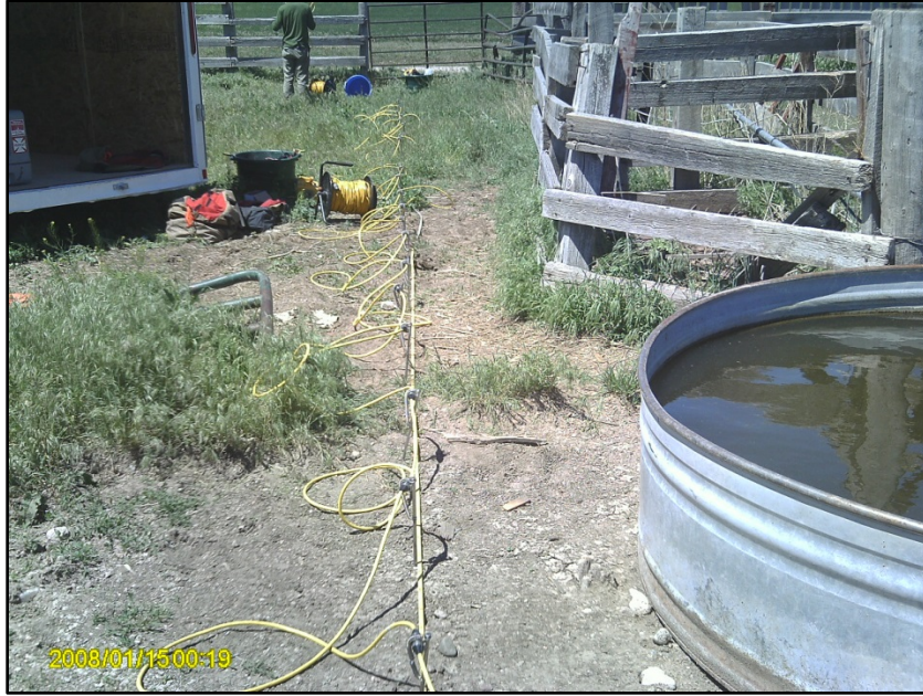
Photo shows the electrodes installed for the resistivity survey.
