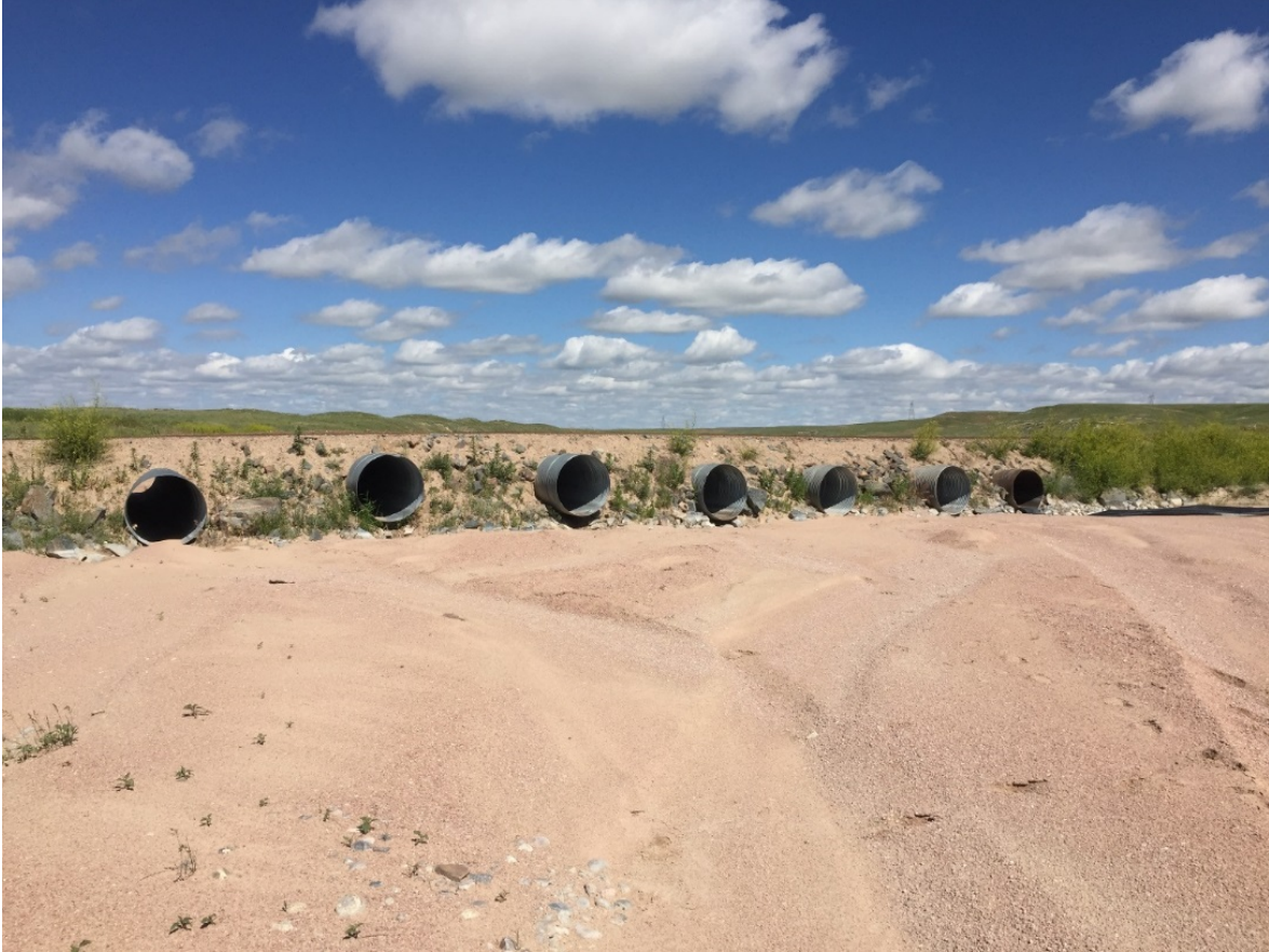
Oil and Gas Roadway Crossing on Lodgepole Creek
