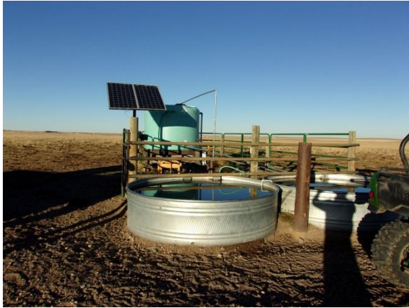
Existing Birdie No. 1 Well and Tanks
