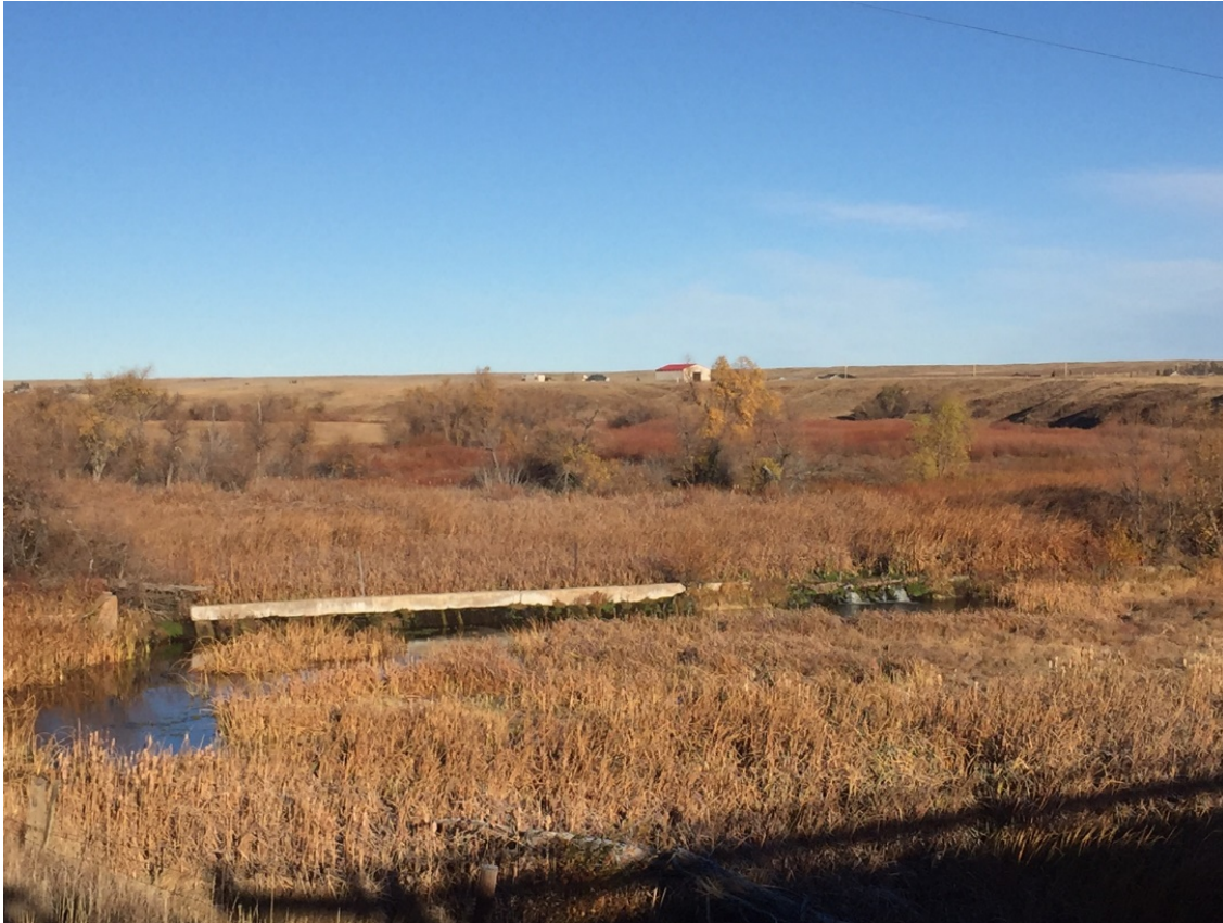
One Mile Ditch Diversion Dam on Lodgepole Creek
