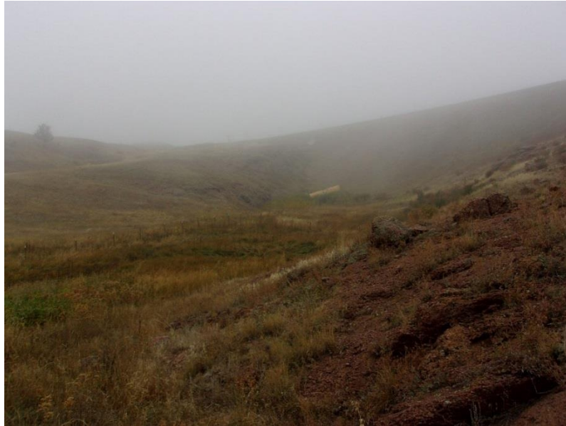
Proposed dam site looking upstream (generally west). The UPRR embankment is visible in the background.
