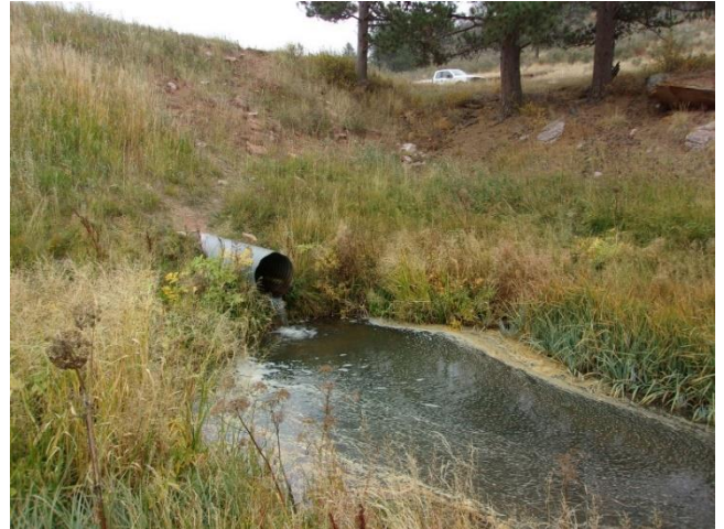
Downstream end of the 24" Outlet pipe
