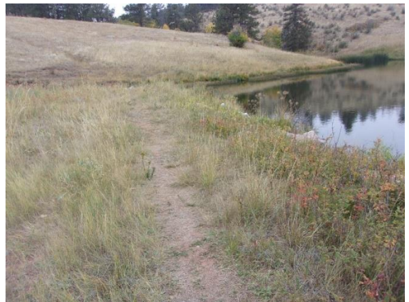
Top of Dam
