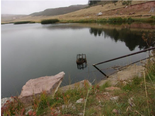
Drop Inlet of Principal Spillway
