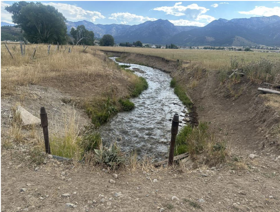
Figure D-45. Photo of the existing Stewart Creek channel west of HWY 89 looking east.
