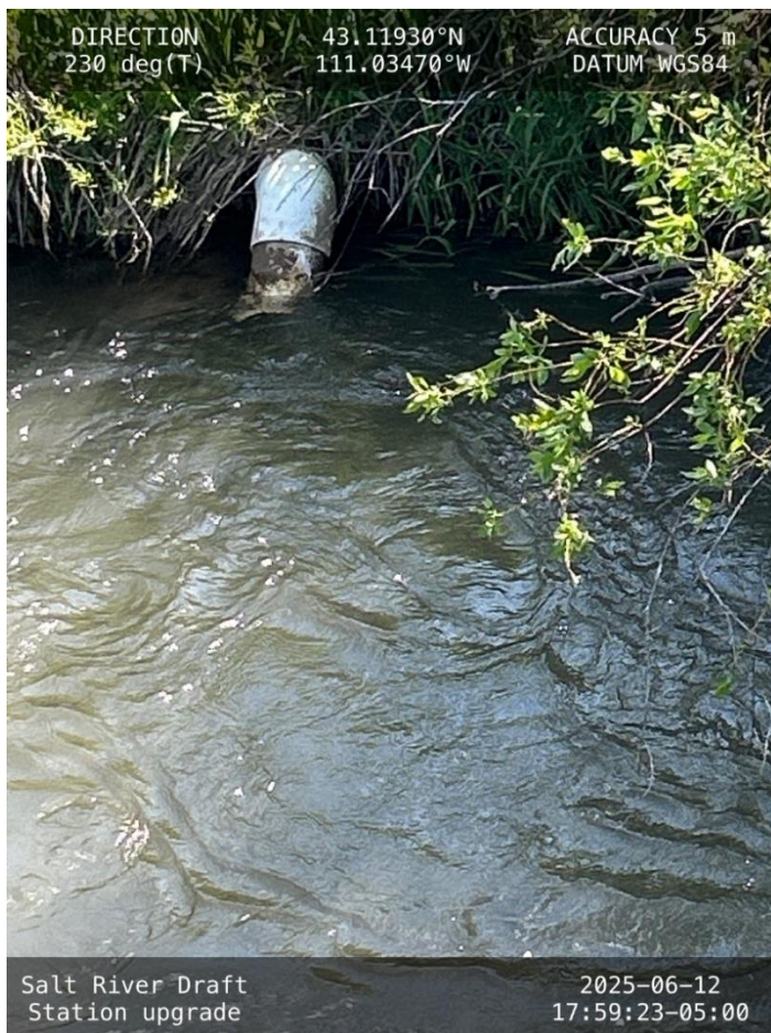
Figure D-35. Existing draft station on Salt River.
