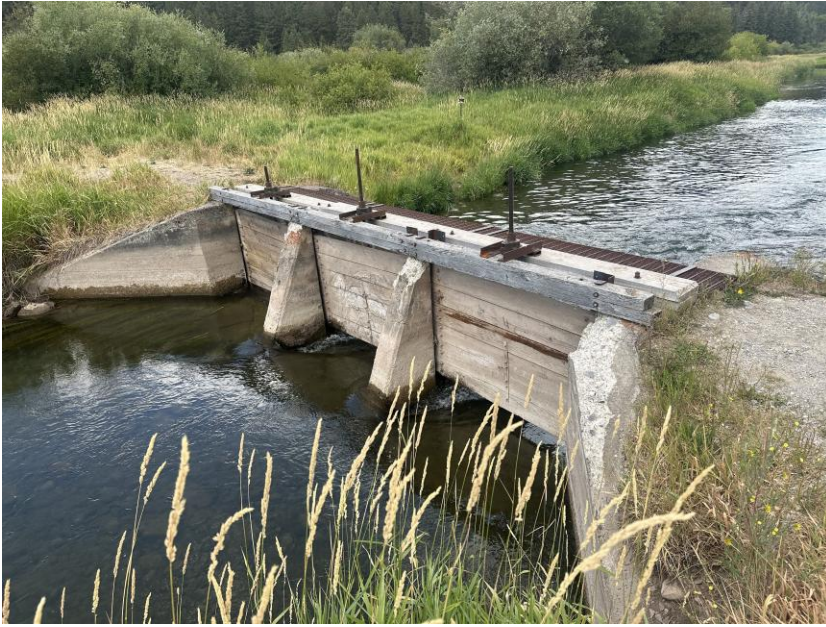
Figure D-1. Photo of existing East Side Canal diversion.
