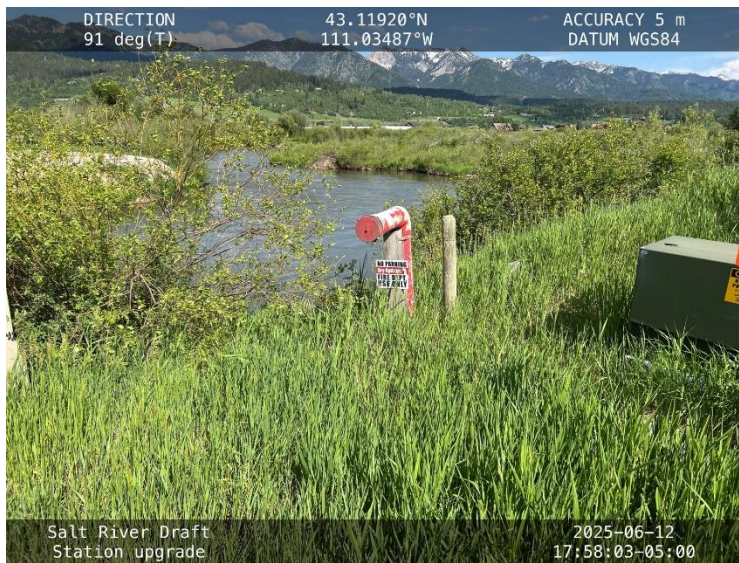
Figure D-34. Existing draft station on Salt River.
