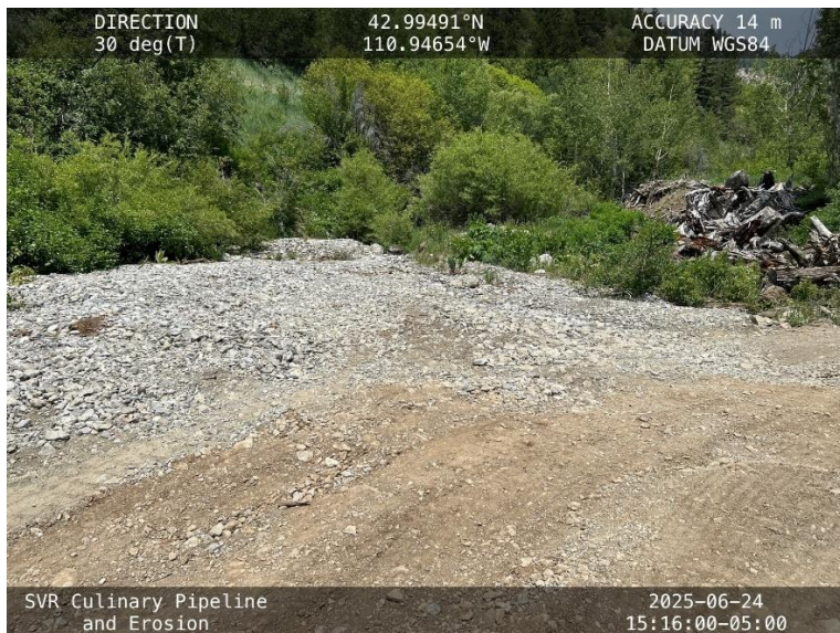
Figure D-48. Existing conditions on Prater Canyon Road.
