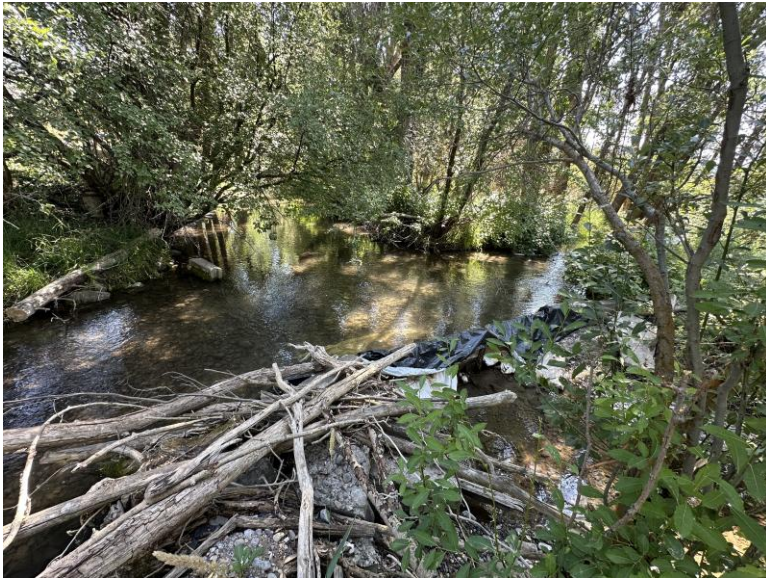
Figure D-7. Photo of existing A Frame Diversion.
