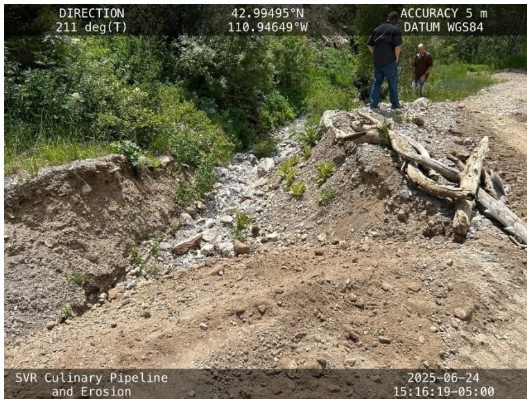
Figure D-50. Existing conditions on Prater Canyon Road.
