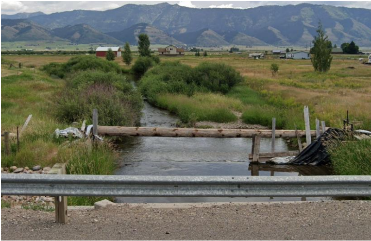
Figure D-10. Existing diversion structure on Stump Creek.
