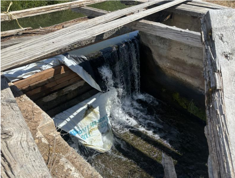
Figure D-4. Photo of existing diversion structure on Willow Creek.
