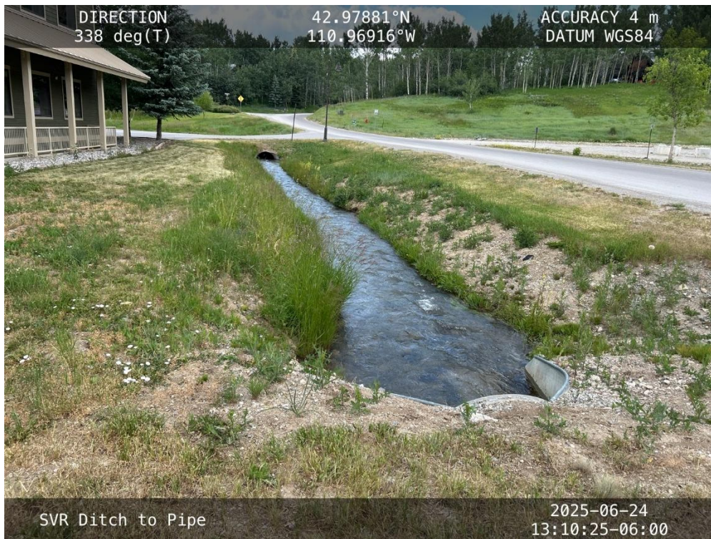
Figure D-21. Existing conditions of Star Valley Ranch area for ditch to pipeline project.
