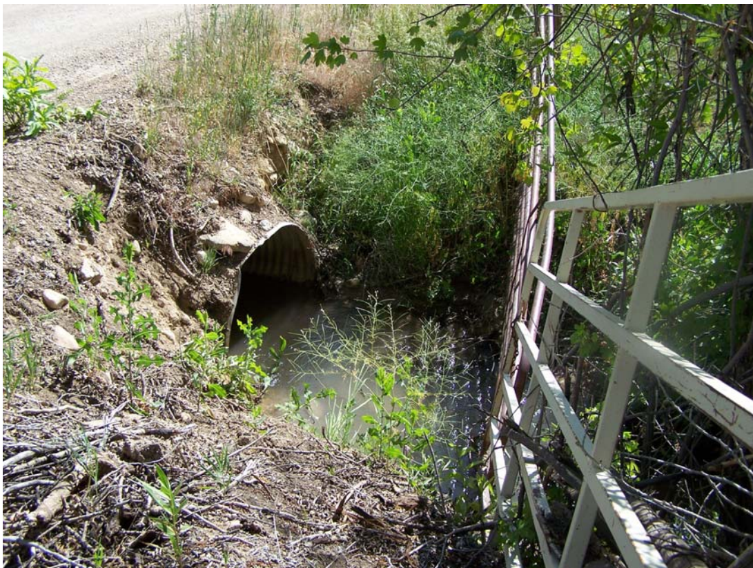
HC-I: Horse Creek at culvert along County Rd 31 (July 10, 2007)
