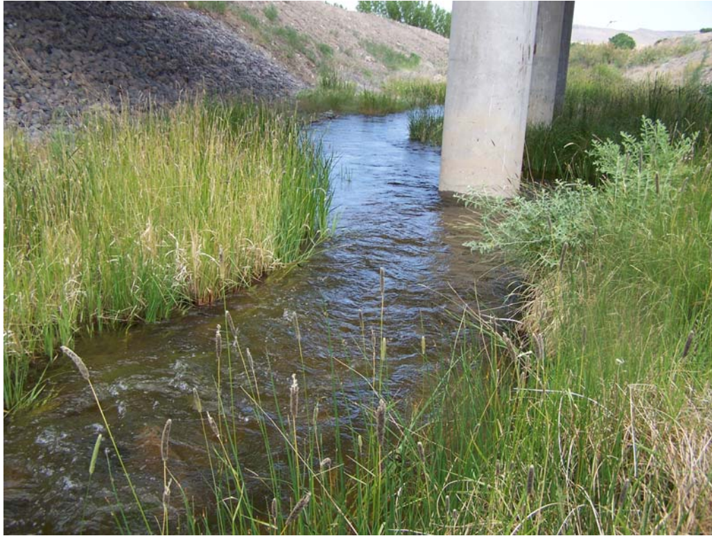
SHG-I: Sheldon Gulch at Hwy 14 crossing (July 10, 2007)
