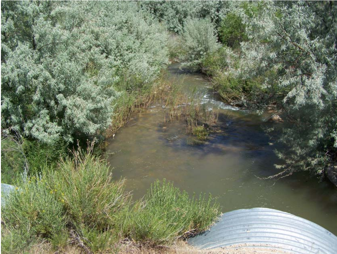
BC-1: Beaver Creek at culvert near Leavitt Reservoir (July 10, 2007)
