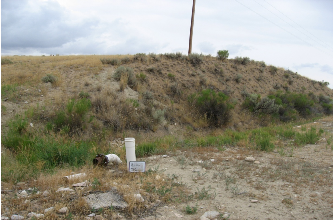
Photo 27: High Line Reservoir Expansion - West Abutment
