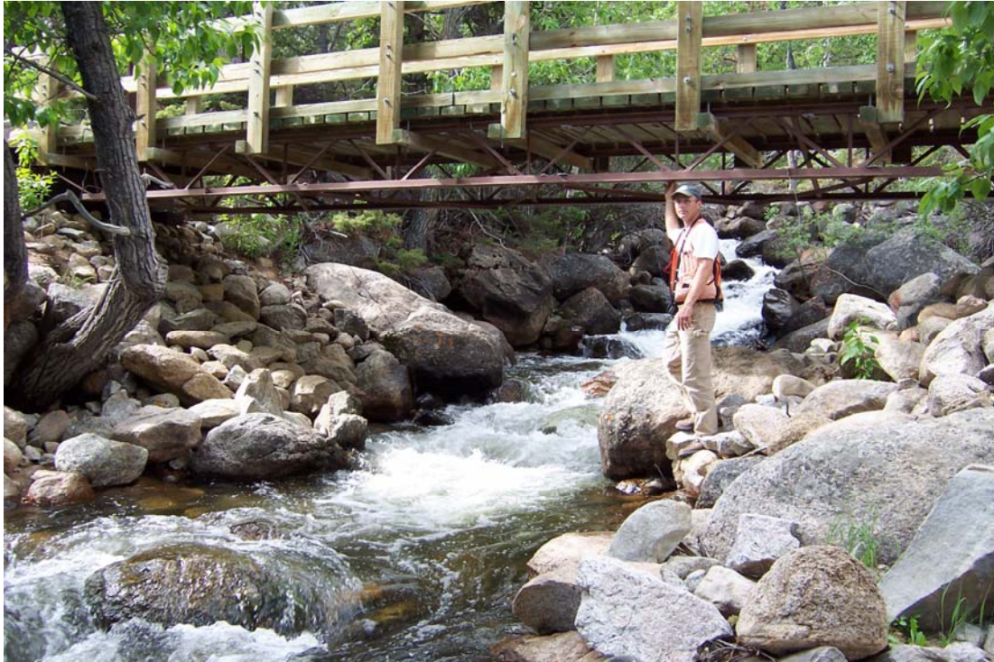
WC-I: Willett Creek at trail bridge (6-22-06)
