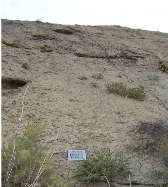
Photo 37: Red Canyon - West Abutment
