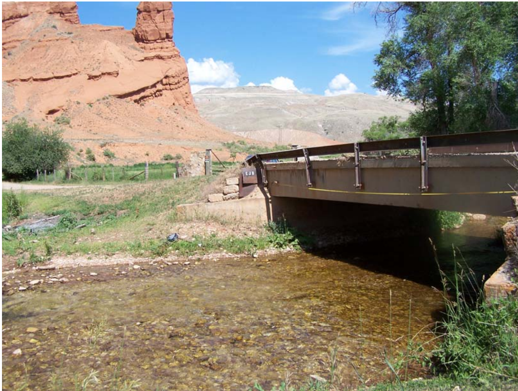
TC-I: Trapper Creek at bridge (July 10, 2007)
