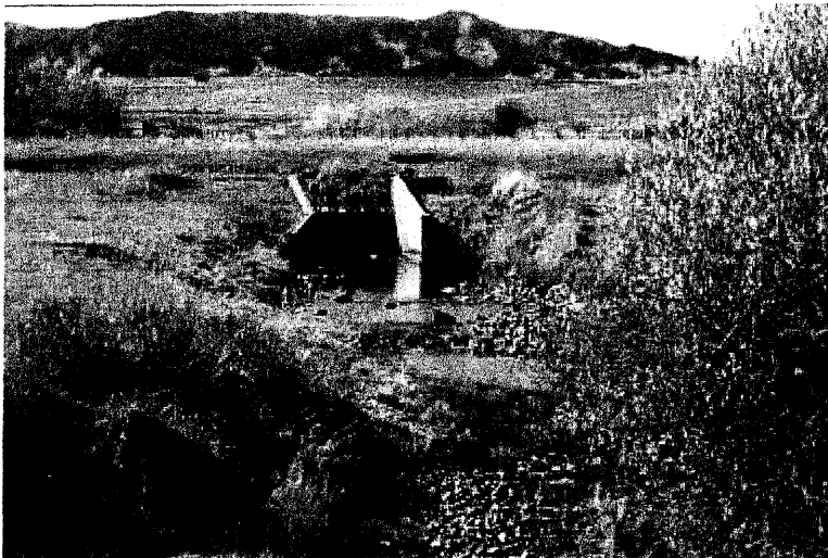
View of diversion
