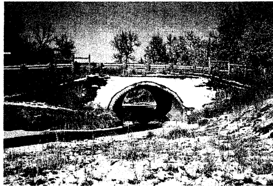
View of culvert
