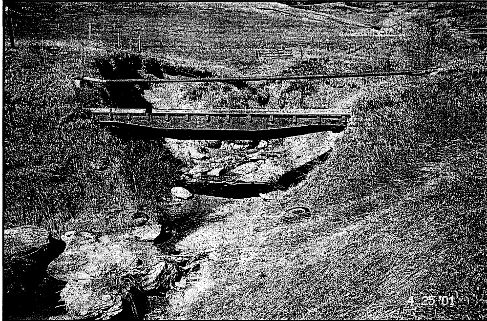
Photo 6, Jenks Creek: widening channel (039)
