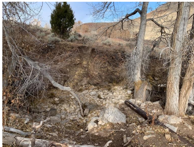
Photo 12. Enterprise Ditch – Cascade Reach Ditch Section.
