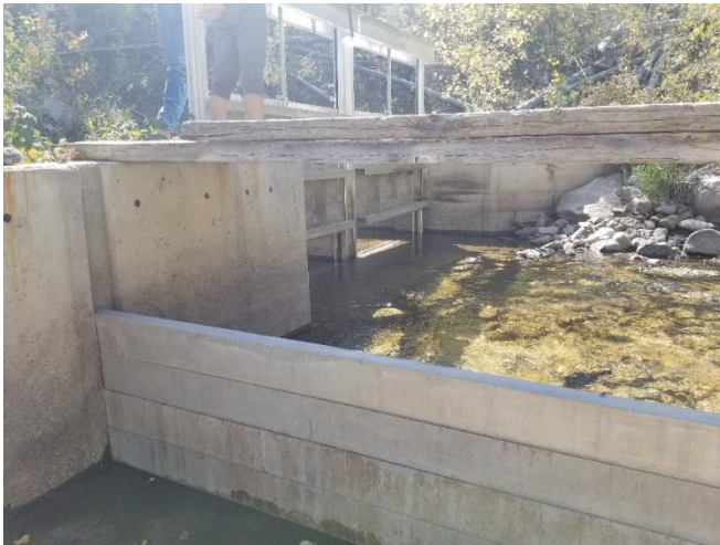
Photo 10. Enterprise Ditch – Sawmill Creek Diversion.
