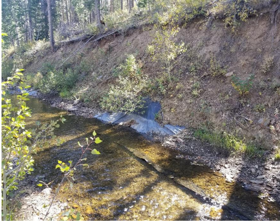
Photo 13. Enterprise Ditch – Sawmill Creek Reach Channel Lining.
