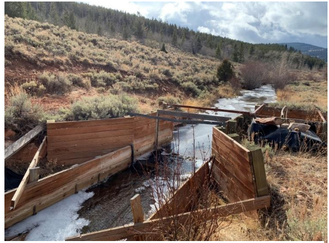
Photo 11. Enterprise Ditch – Crooked Creek Diversion.
