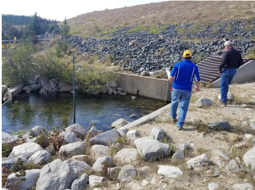
Photo 15. Outlet structure at Worthen Meadows Reservoir.
