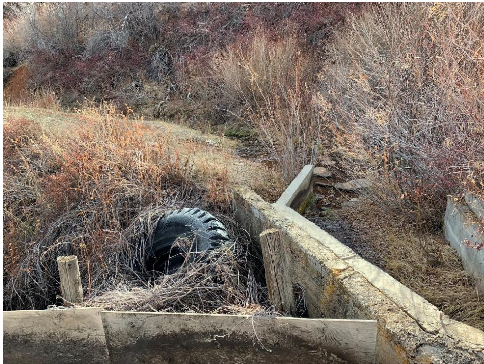
Photo 14. Enterprise Ditch Thompson Lateral Headgate and Drop Structure
