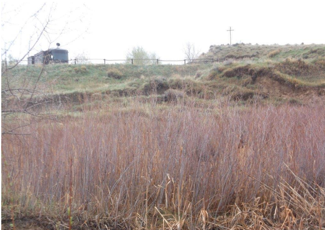
Photo 8. Hillslope Instability Below Dutch Flat / Taylor Ditch near Highway 287.
