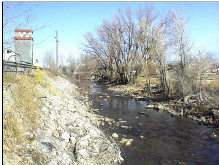
Figure 4.17 Bank Stabilization and Channelization of Middle Popo Agie River (Site MPA-4: Type-B3c Channel).
