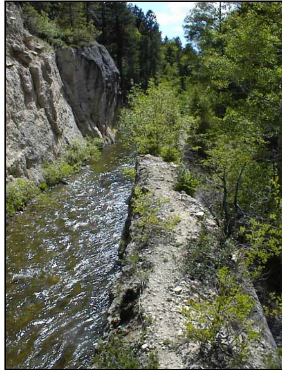
Figure 5.11 Rock Cut Segment of the Enterprise Ditch between Sawmill Creek and Crooked Creek.
