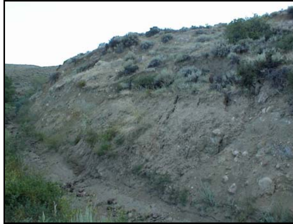
Figure 5-24 Example of Erosive Reach on Nicol-Table Mountain Ditch.
