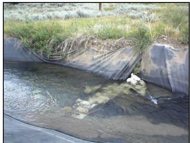
Figure 5.10 Installation of Geomembrane on the Dutch Flat/Taylor Ditch.
