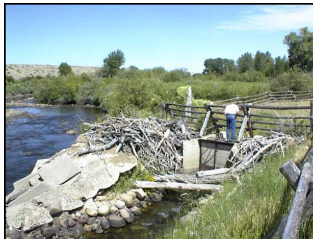
Figure 5.26 North Fork Ditch Headgate and Diversion Structure.
