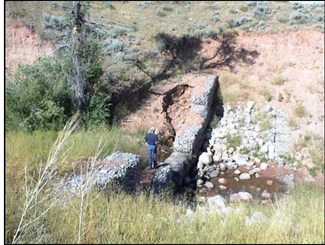
Figure 5. 13 One of Five Rock Gabion Drop Structures Located on Beason Creek.
