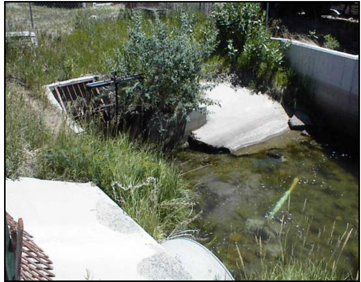
Figure 5.9 Taylor / Dutch Flat Ditch Siphon Inlet.
