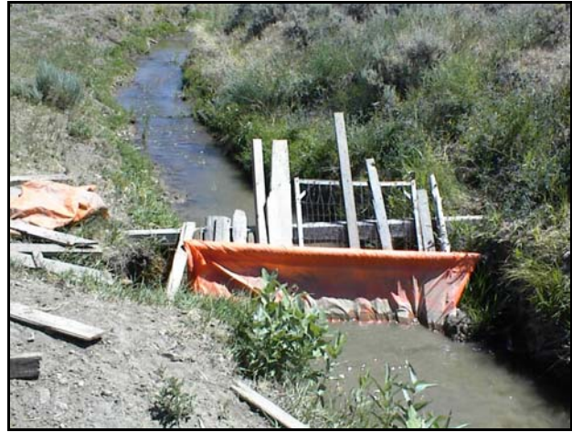
Figure 5.27 Turnout Structure on North Fork Ditch.
