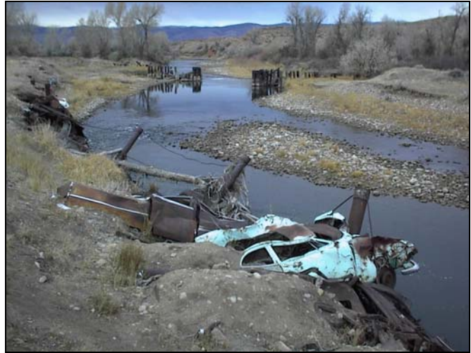
Figure 4.22 Bank Stabilization Efforts on the Popo Agie River (Site PA-3: Type-C3 Channel).
