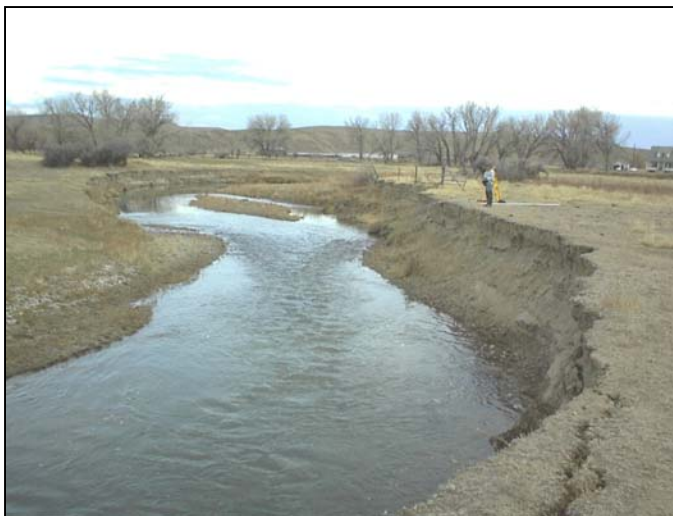
Figure 1.6 Stream Bank Erosion on Little Popo Agie River.
