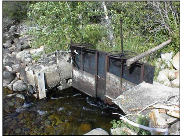
Figure 5.22 Nicol-Table Mountain Ditch Diversion Structure.
