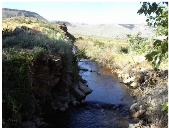
Figure 5.23 Sandstone Bedrock Reach of the Nicol-Table Mountain Ditch with Reduced Conveyance Capacity.
