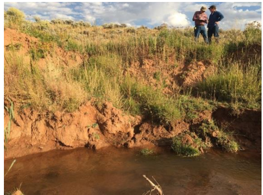
SCS-003 Same location showing erosion on Red Creek
