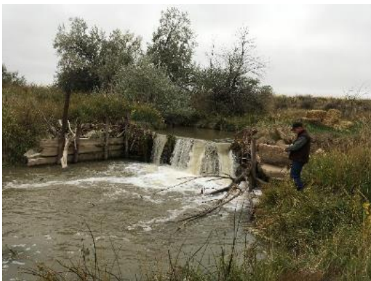
SCS-004: Check structure on Owl Creek
