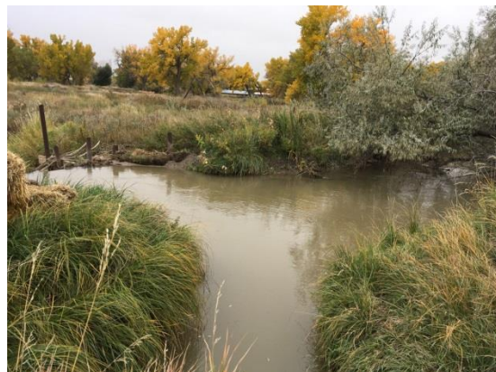
SCS-004: Check structure and diversion
