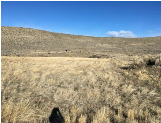
Silted reservoir pool level with spillway looking NW 50' upstream of top of cut.
