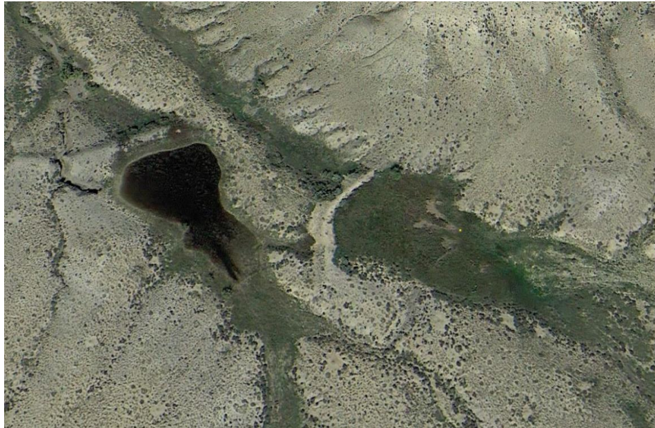
Figure 3.9.3-2b. Example of a Non-Functional reservoir. Old reservoir (on the right) breached leaving it non-functional. (Source: NAIP Imagery 2015)
