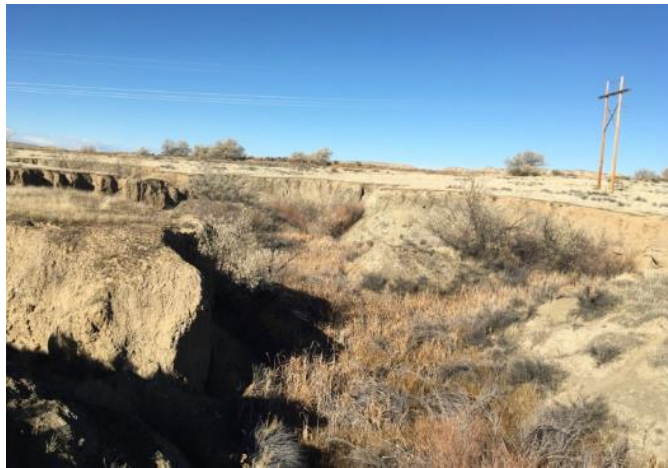
OWI-005: Drainage Channel and Historic Embankment
