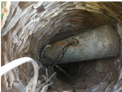
URI-002: Existing Well, Highpoint looking at Reservoir
