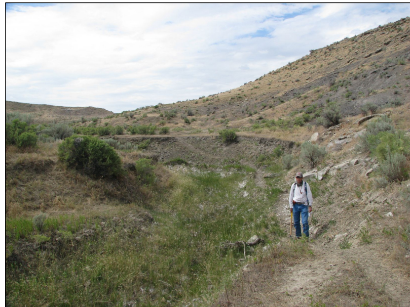
C DRAINAGE BOTTOM UPSTREAM OF EMBANKMENT LOCATION
