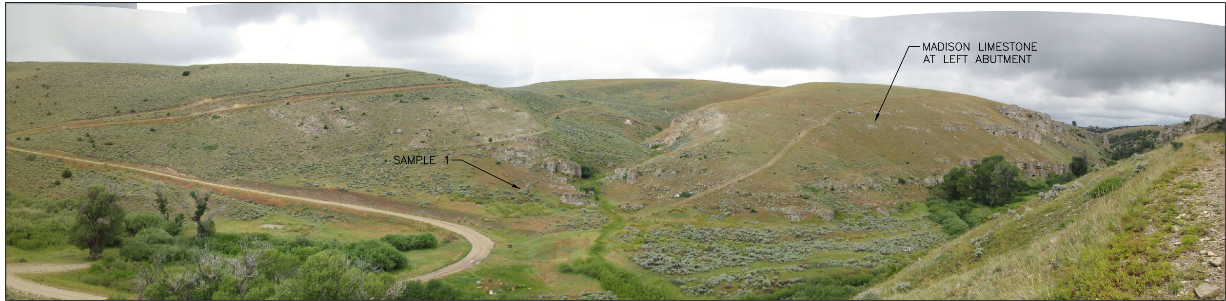
A VIEW OF LEFT ABUTMENT
