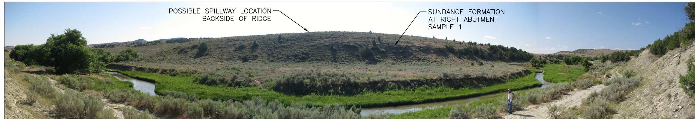
B VIEW OF RIGHT ABUTMENT
