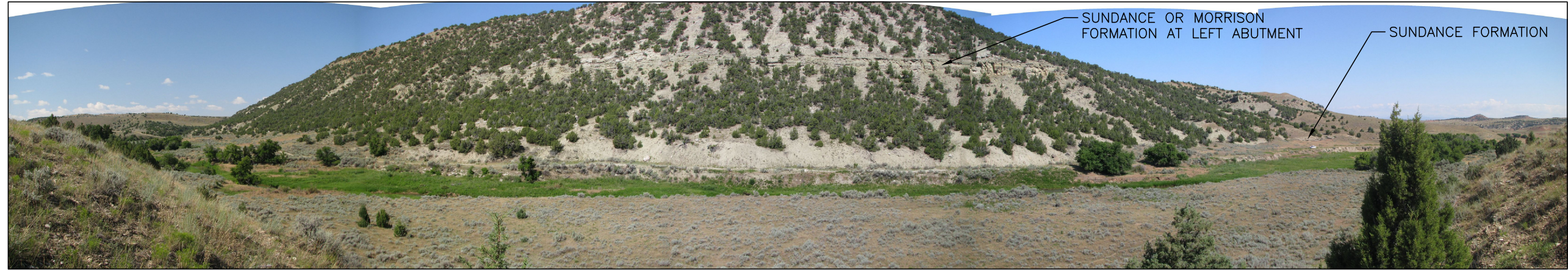
A VIEW OF LEFT ABUTMENT
