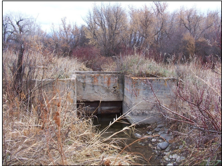
Figure 3.69 Headgate Structure on Victoria Ditch
