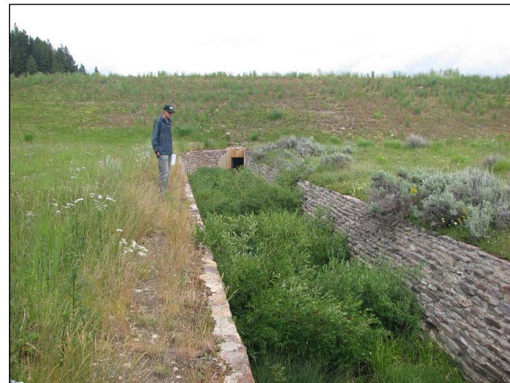
B PRIMARY OUTLET CHANNEL
