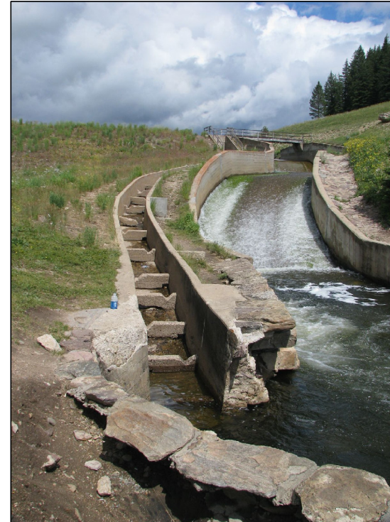
C SPILLWAY AND FISH LADDER
