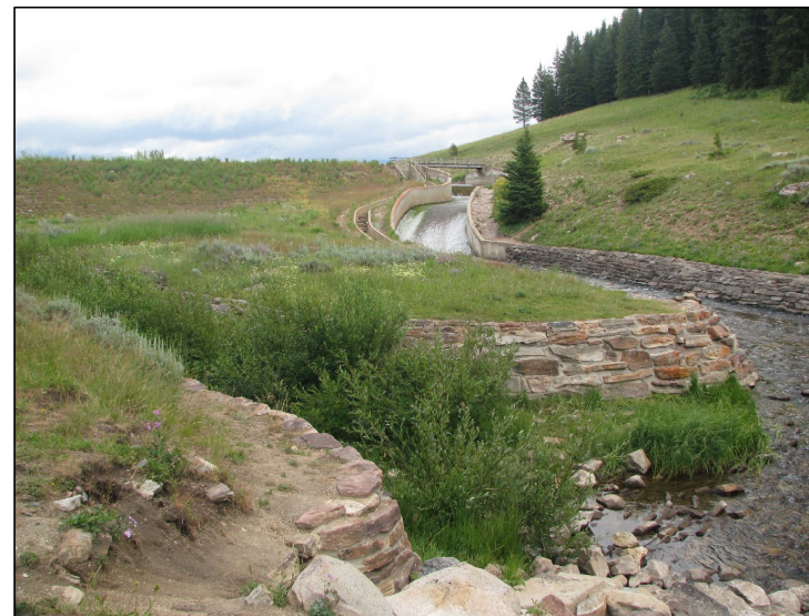
D DOWNSTREAM END OF PRIMARY OUTLET CHANNEL
