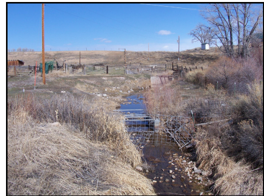
Figure 1.4 Typical Irrigation Ditch in Nowood River Watershed: Anita Ditch
