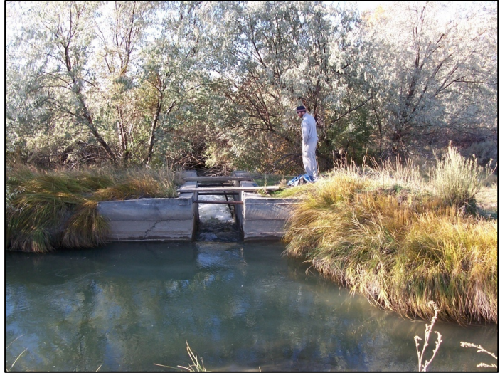
Figure 3.67 Wasteway Structure on the Shafer Ditch
