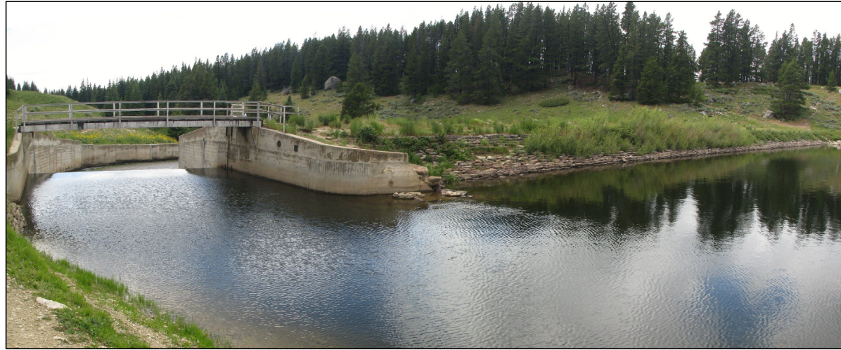
A UPSTREAM FACE OF EMBANKMENT
