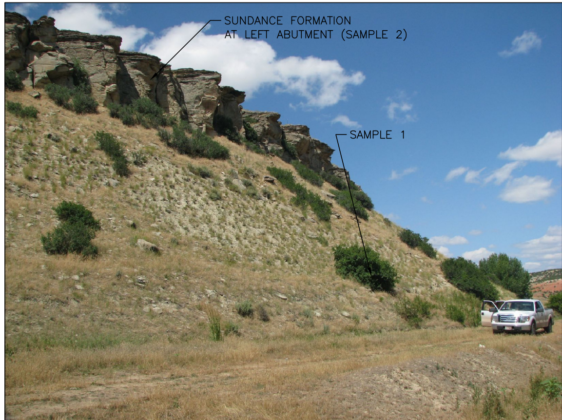
B VIEW OF LEFT ABUTMENT SHOWING SANDSTONE CAP OVER GYPSUM
