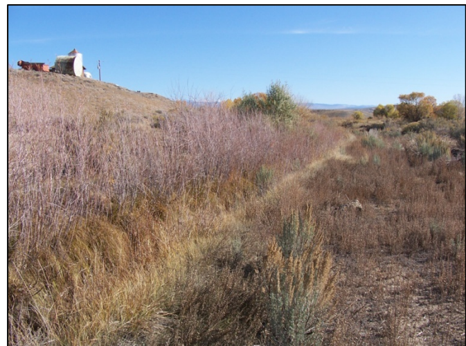
Figure 3.68 Reach of Shafer Ditch with Excessive Vegetation on Banks and Bed
