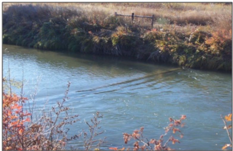
Figure 3.70 Exposed Siphon Crossing on the Nowood River
