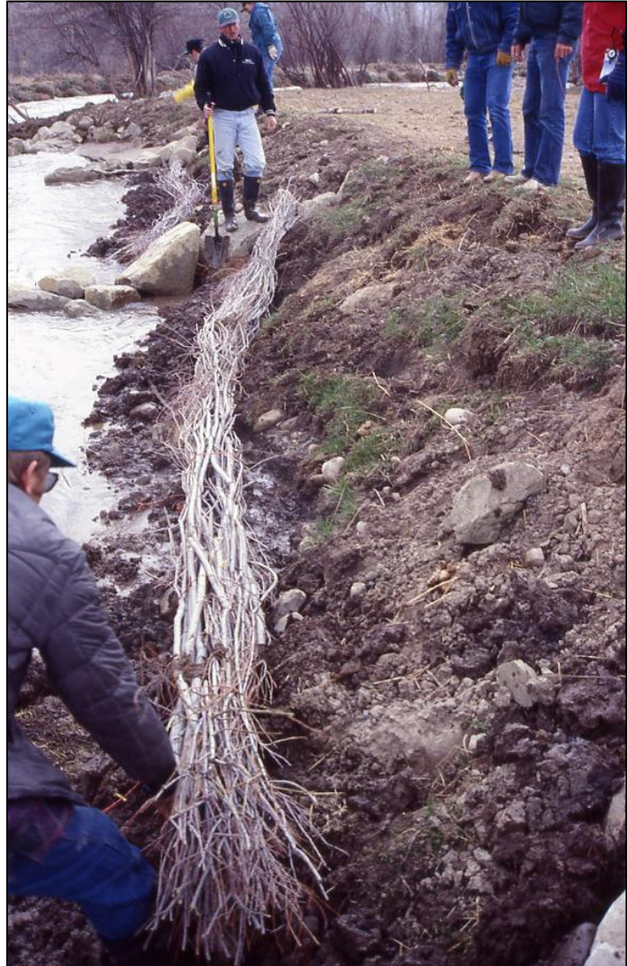
Figure 4.56 Stream Stabilization Measure: Willow Fascine Installation
