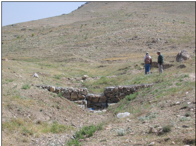
Figure 4.55 Stream Stabilization Structure: Rock Filled Gabion
