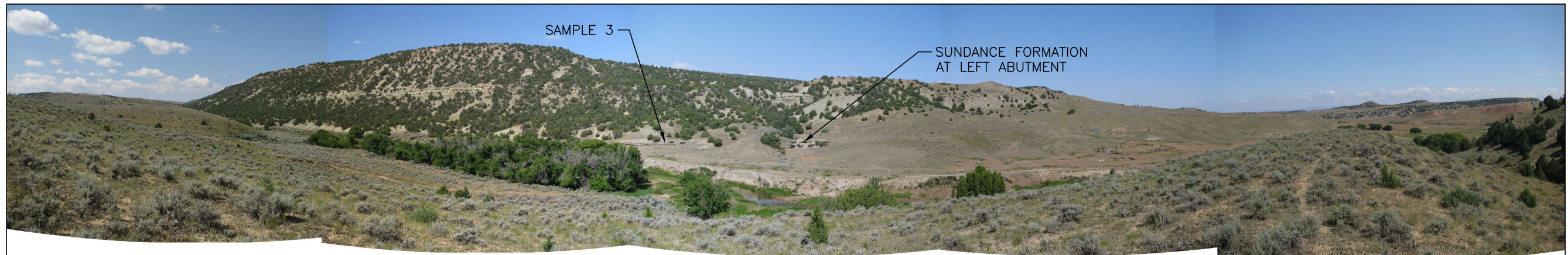
A VIEW OF LEFT ABUTMENT
