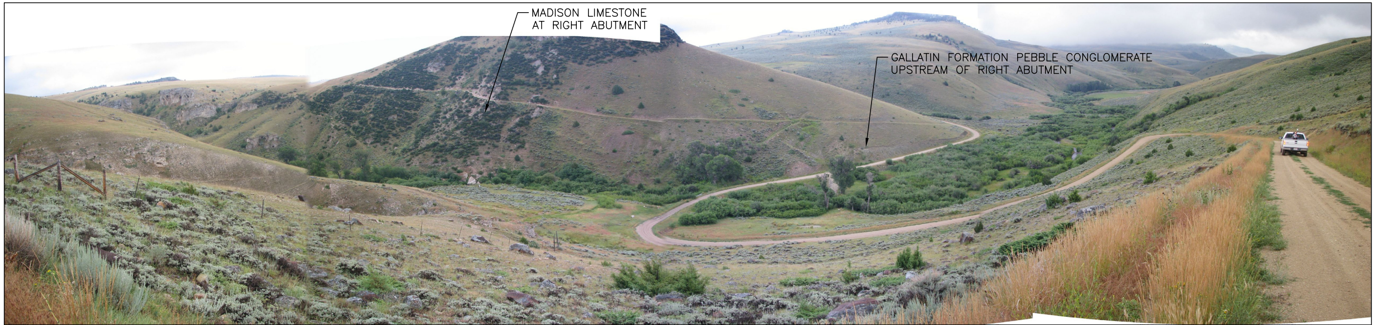
B VIEW OF RIGHT ABUTMENT
