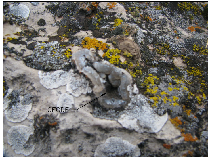
B SOLUTION FEATURE IN OUTCROP NEAR LEFT ABUTMENT
