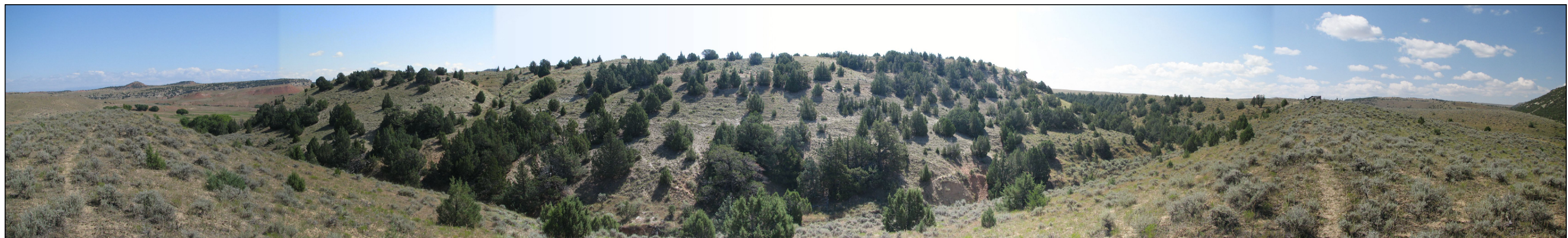
C VIEW OF POSSIBLE SPILLWAY CHANNEL BEHIND RIDGE AT RIGHT ABUTMENT
