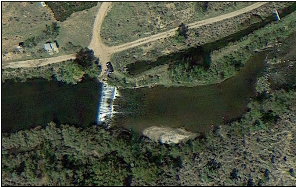
Figure 4.3-6 Encampment Platte Valley Ditch Diversion Structure.
