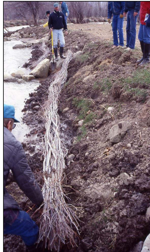
Figure 4.7-8 Stream Stabilization Measure: Willow Fascine Installation.
