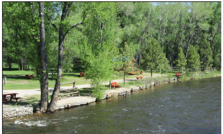
Figure 4.7-3 Encampment River Bank Stabilization Downstream of Highway 230.
