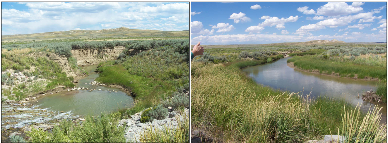
Figure 4.7-7 Channel Gradient Restoration Feature on Muddy Creek near Baggs, WY. Photo on left is viewed downstream from the dam at incised channel. Photo on the right is viewed upstream at restored gradient.
