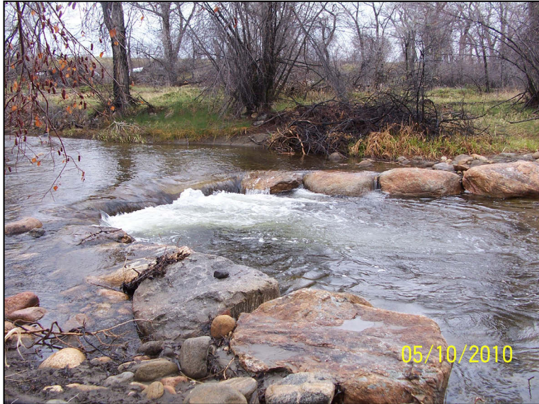
Figure 4.7-6 Stream Stabilization Structure: Rock Vortex Weir.
