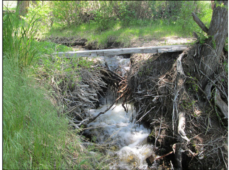
Figure 4.7-2 Headcut on Cumberland Gulch at Pennock Ranch.
