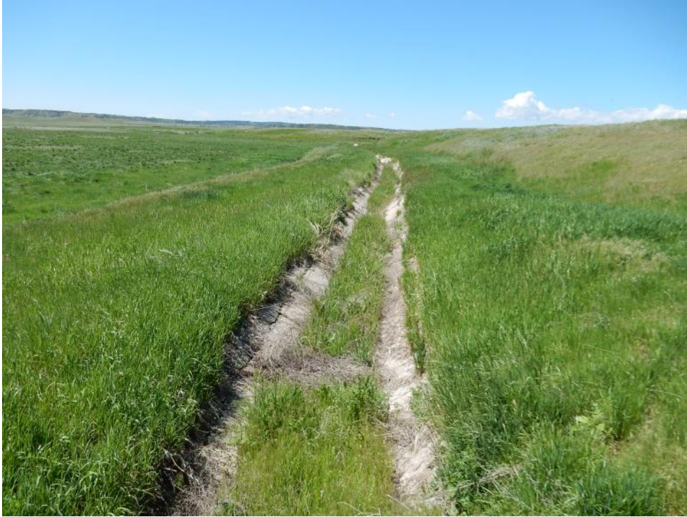
Figure 3.54. Johnson Pump Lift ACT Cassa Ditch With Accumulated Sediment and Vegetation Growth.
