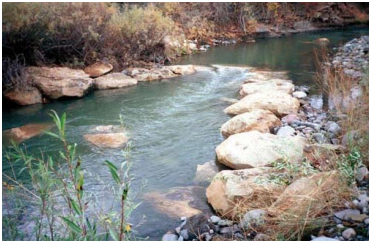
Figure 4.33. Cross Vane Installed on the Blanco River in Colorado (Adapted From NRCS [2007]).
