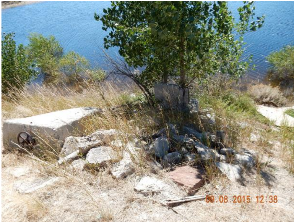
Figure 3.38. Existing Outlet Works for the East Side No. 3 Reservoir.
