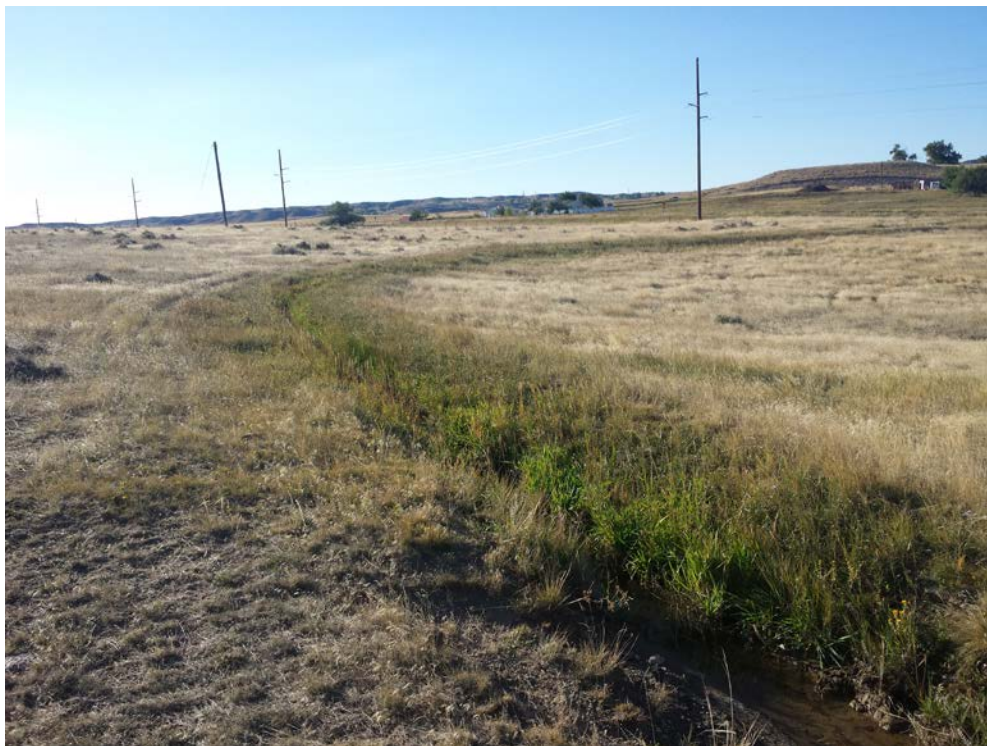
Figure 3.48. Downstream View of Lateral No. 4 Sublateral From the Headgate on Lateral No. 4.
