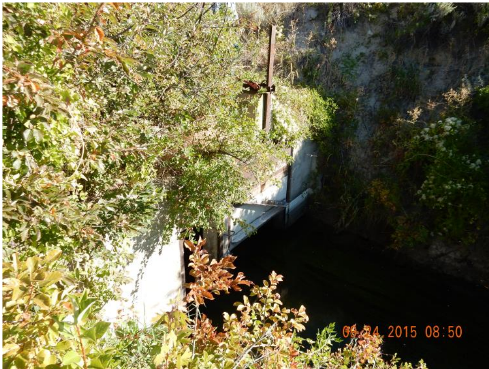
Figure 3.44. LaPrele Westside Canal Slide Gate and Entrance Into Tunnel No. 1.
