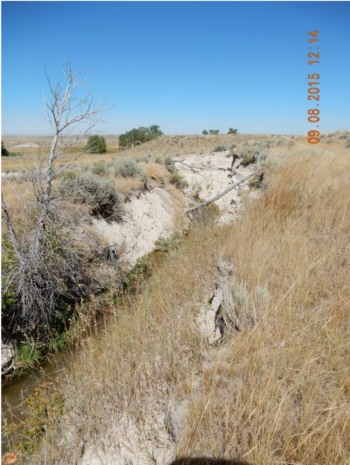
Figure 3.35. Eroding Section of the LaPrele Lateral No. 1.
