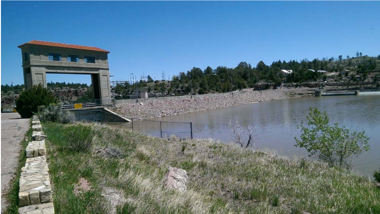
Figure 3.111. Downstream View of Guernsey Reservoir Dam and Existing Outlet Works.
