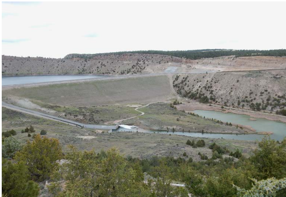
Figure 3.109. Existing Outlet Works for the Glendo Reservoir.
