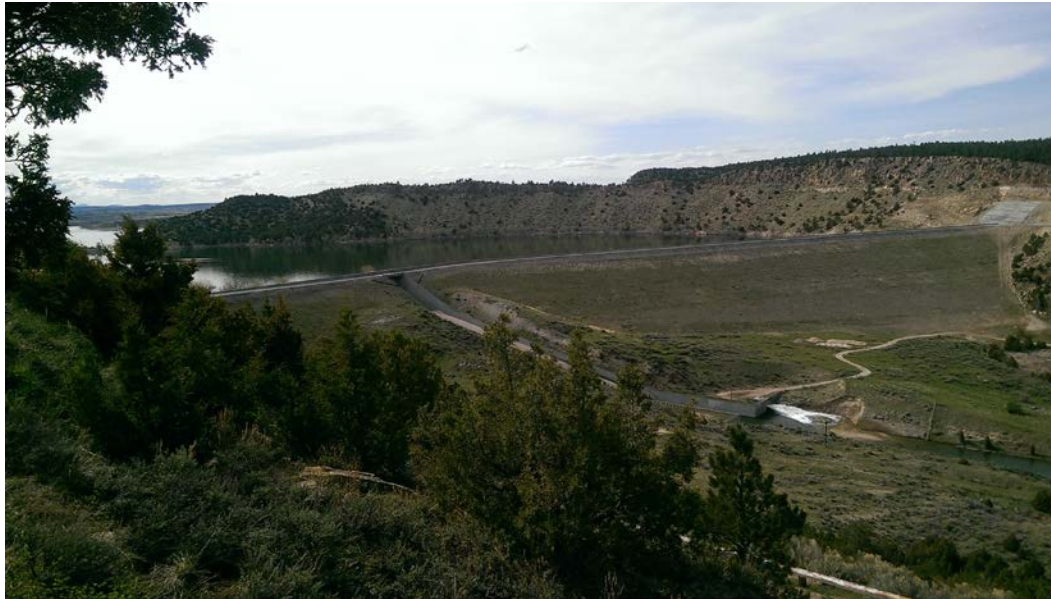
Figure 3.108. View of Glendo Dam and Reservoir (Looking Upstream).
