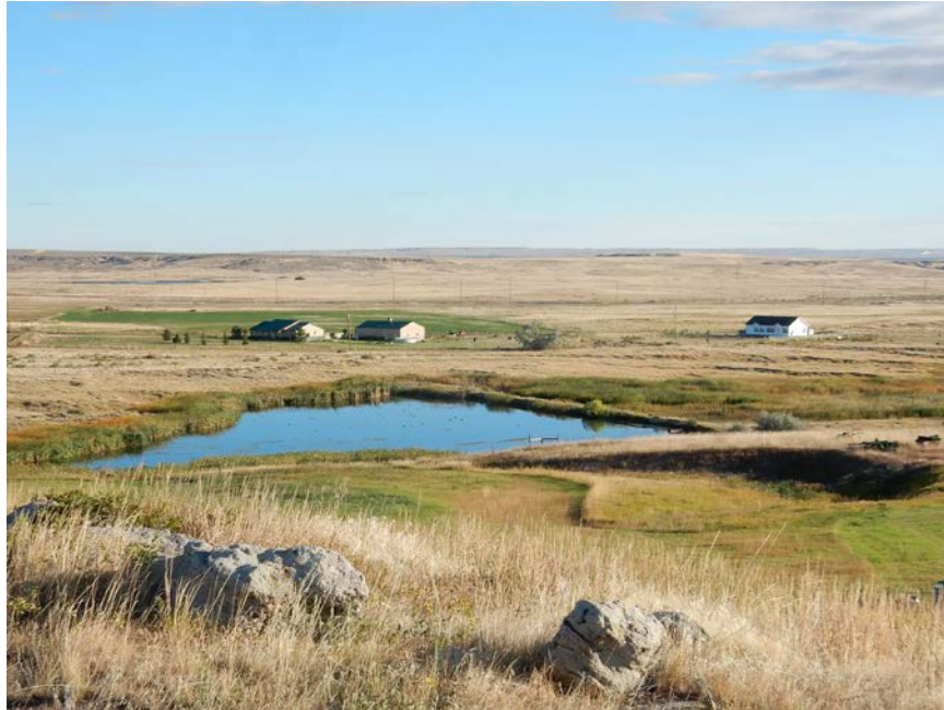
Figure 3.122. Downstream View of the Larime No. 1 Reservoir.
