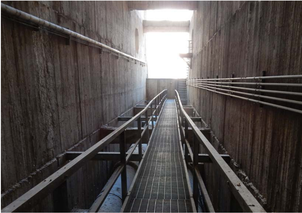
Figure 3.116. View From Inside the Hollow Reinforced Concrete Dam of LaPrele Reservoir.
