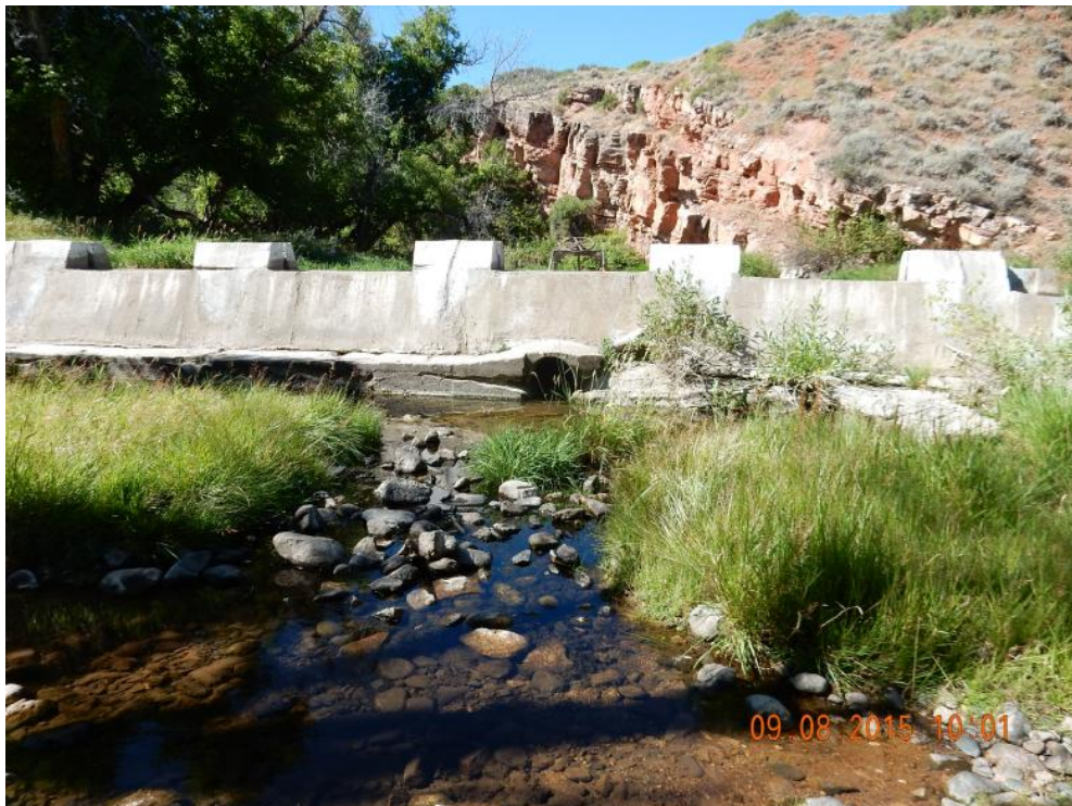
Figure 3.42. LaPrele Westside Canal Diversion Weir and Bypass Pipe (Middle).
