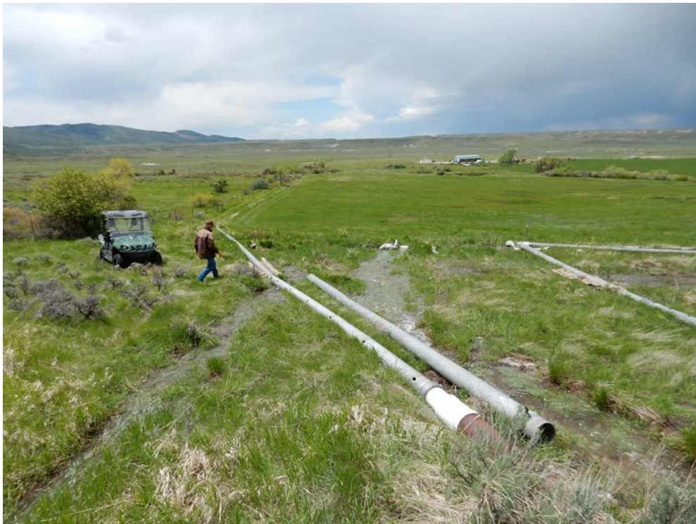
Figure 3.60. Seepage Saddle Ditch and Delivery System.
