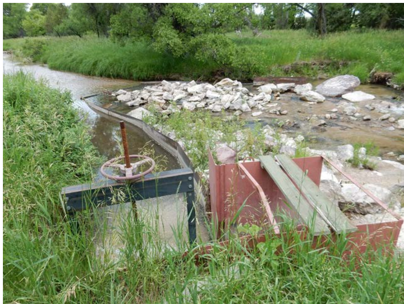
Figure 3.57. Wright No. 2 Ditch Enlargement Cross-Vane Weir (Middle) and Bank Scour (Upper Right).
