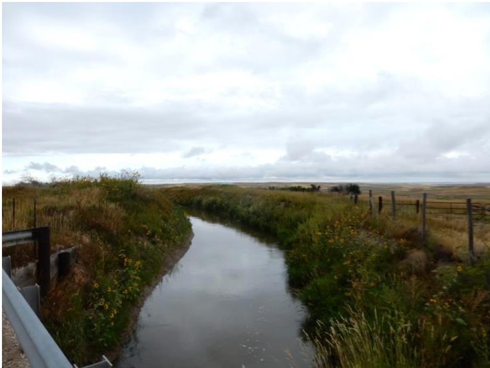
Figure 3.34. LaPrele Main Canal After Maintenance at Station 309+70 From Nelson [1983].
