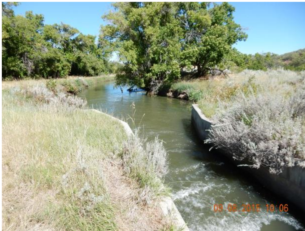
Figure 3.32. Downstream View of LaPrele Main Canal at SEO Hydrology Station 0120ETMD.
