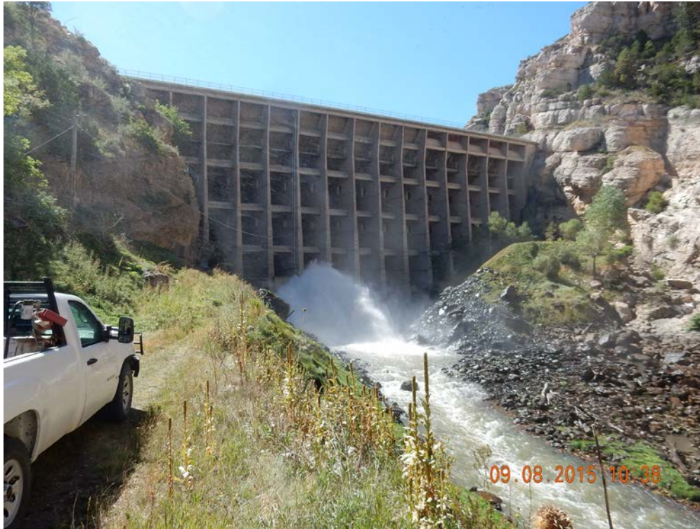
Figure 3.114. Existing Outlet Pipe for the LaPrele Reservoir.
