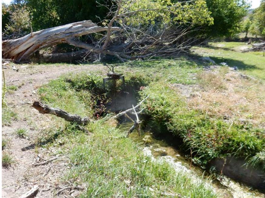
Figure 3.56. Wright No. 2 Ditch Diversion and Headgate Structure.
