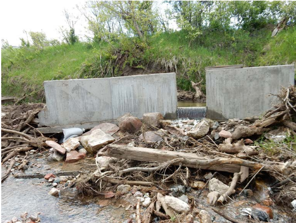
Figure 3.59. Seepage Saddle Ditch Concrete Diversion Structure on Hunton Creek.
