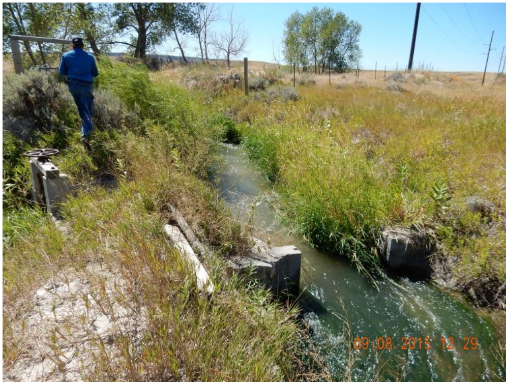
Figure 3.37. LaPrele Lateral No. 1 Near the Main Canal Headgate.
