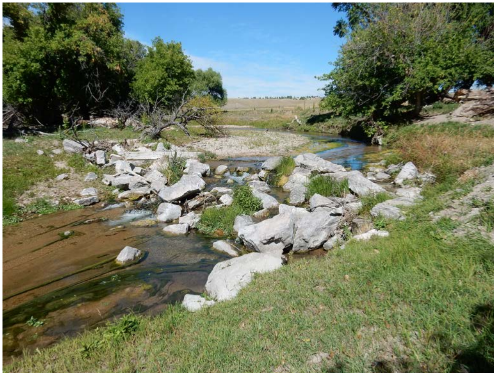
Figure 3.55. Wright No. 2 Ditch Rock Weir.
