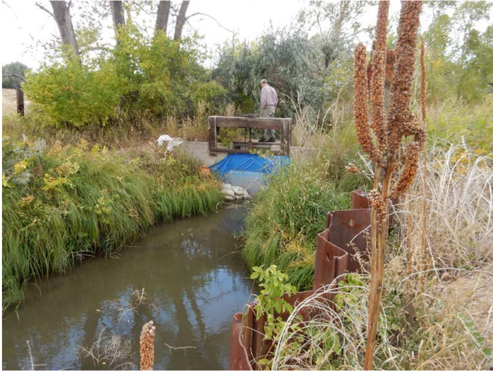
Figure 3.61. Carey Ditch No. 2 Diversion and Headgate Structure.
