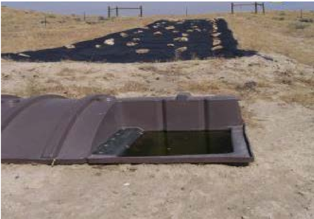
Figure 4.29. An Example of an Installed Wildlife Guzzler System.
