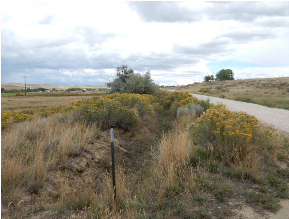
Figure 3.64. Earthen Section of Carey Ditch No. 2.
