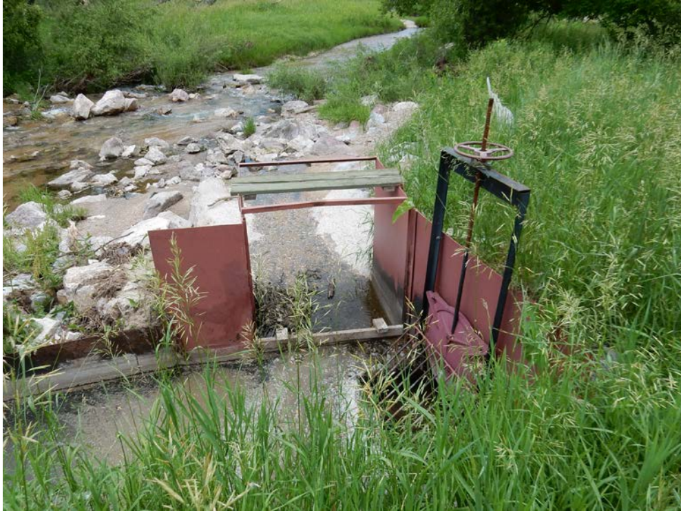
Figure 3.58. Wright No. 2 Ditch Enlargement Headgate and Bypass Structure.
