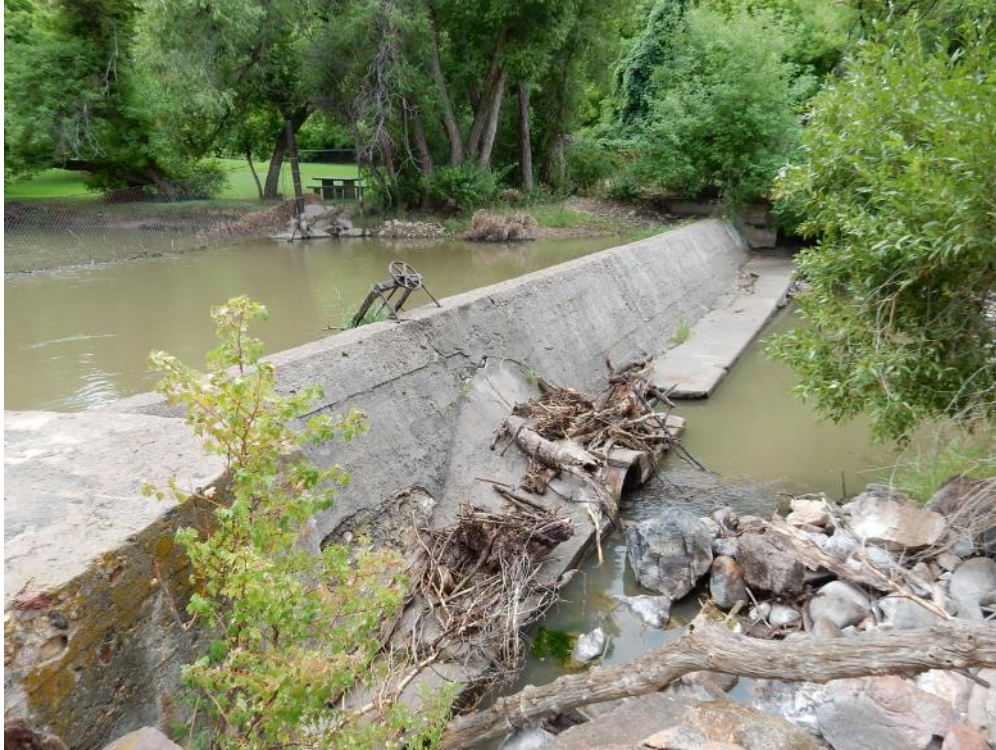
Figure 3.25. LaPrele Main Canal Diversion Weir and Bypass Pipe (Middle).
