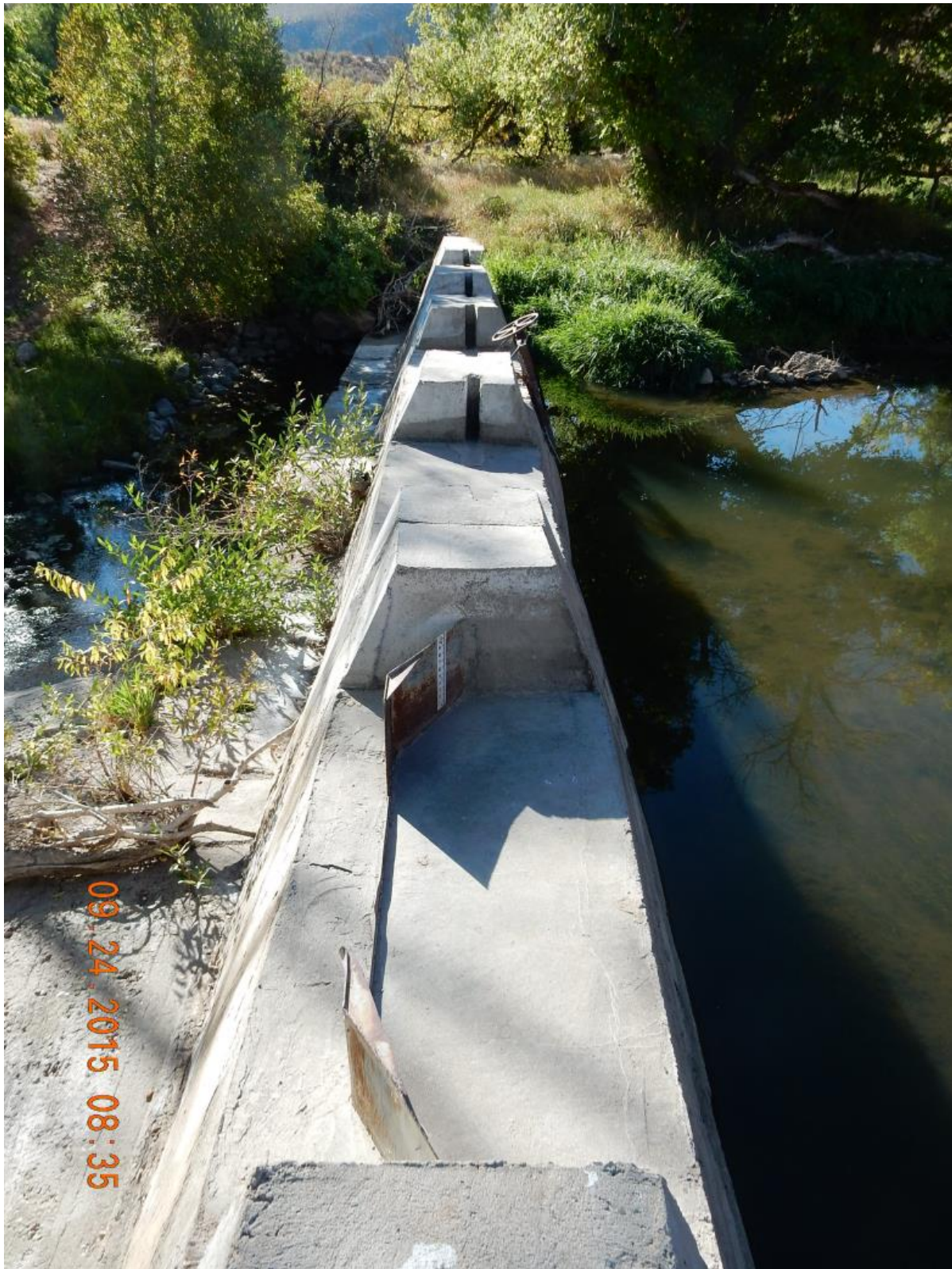
Figure 3.40. LaPrele Westside Canal Diversion Weir and Bypass Pipe (Middle).
