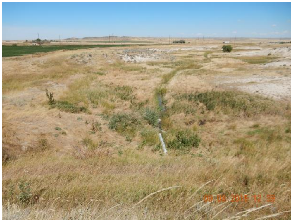
Figure 3.39. Outlet Pipe From East Side No. 3 Reservoir Into Lateral No. 2.
