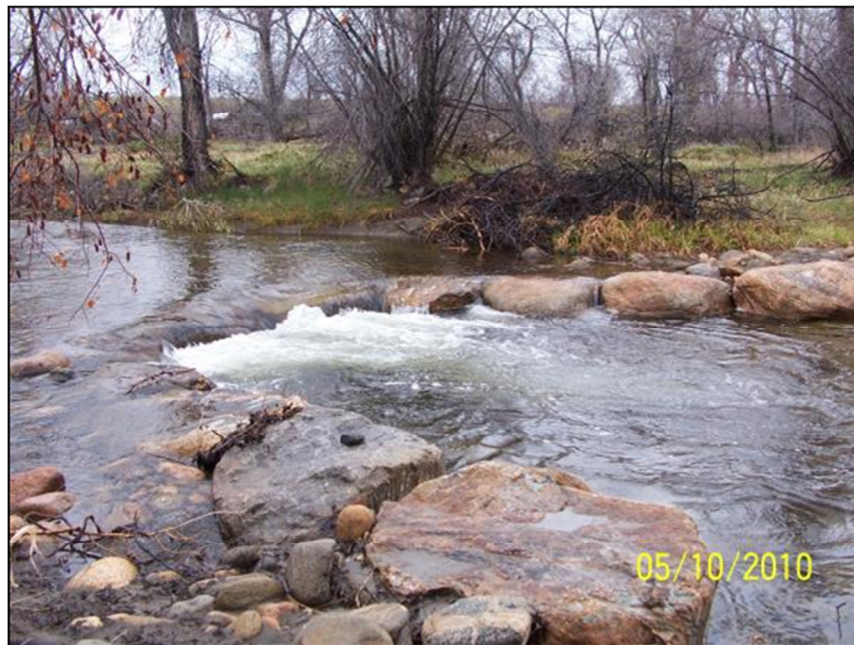
Figure 4.51. Stream Stabilization Structure: Rock Vortex Weir.
