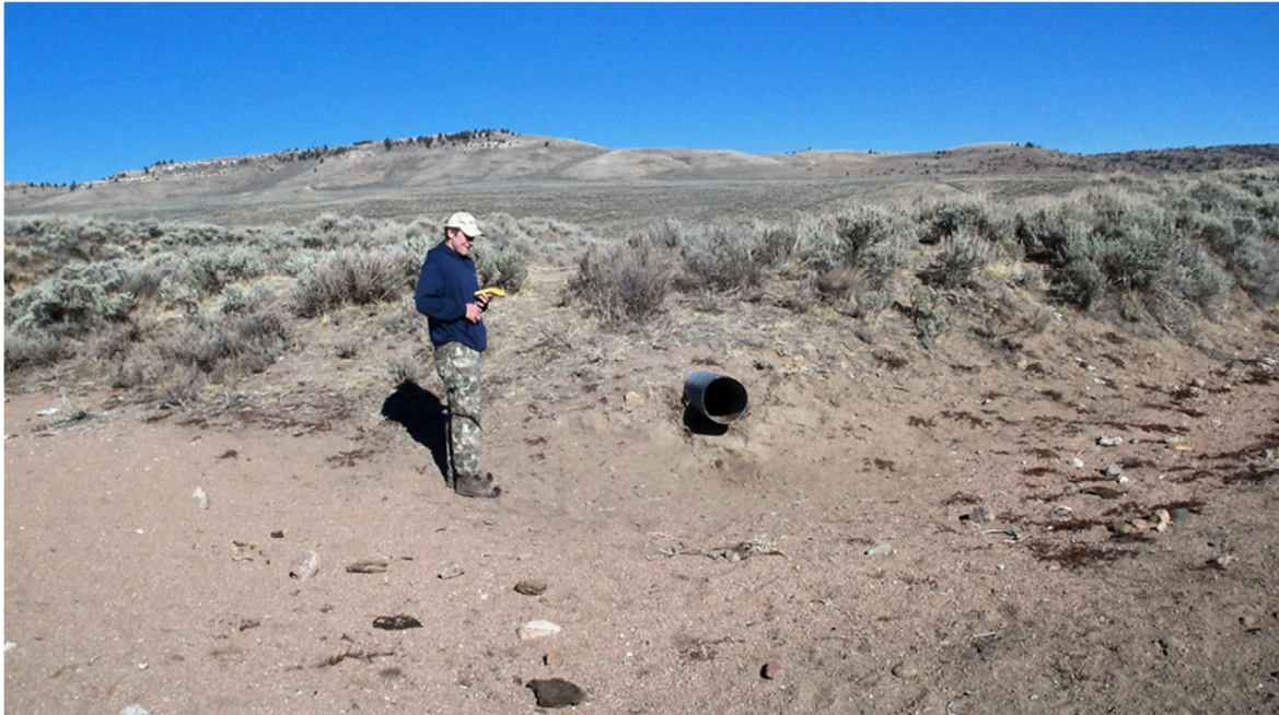
Figure 4.44. Typical Drain Pipe Installed Within the Diversion/Inlet Ditch.
