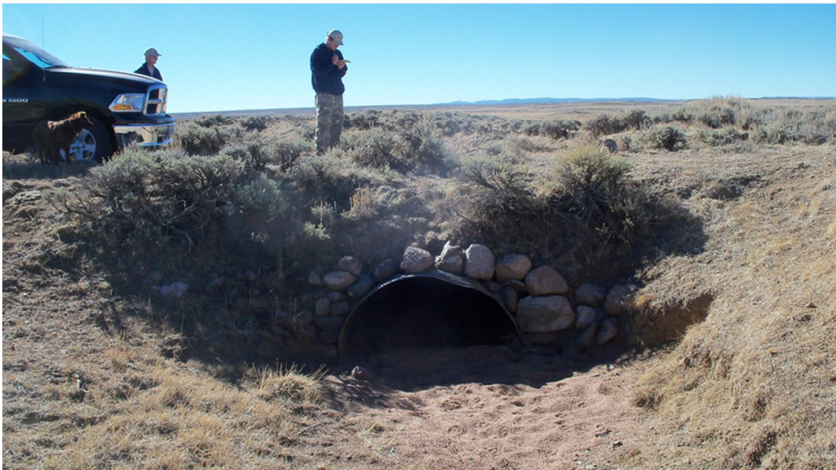
Figure 4.43. Corrugated Arch Pipe Crossing of the Diversion/Inlet Ditch.
