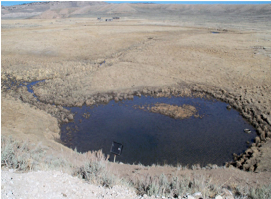
Figure 4.42. Seepage Below the Dam Embankment.
