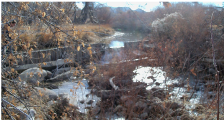
Figure 4.3. Diversion Dam/Check Structure on Bates Creek.
