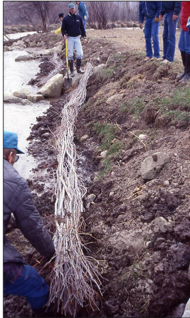
Figure 4.53. Willow Fascine Installation.
