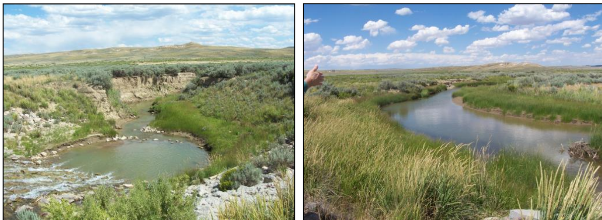
Figure 4.52. Channel Gradient Restoration Feature on Muddy Creek Near Baggs, Wyoming. Photograph on the left is viewed downstream from the dam at incised channel; photograph on the right is viewed upstream at restored gradient.
