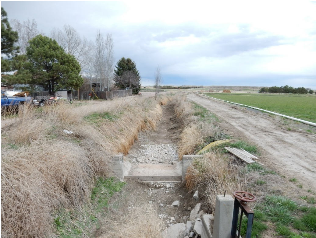
Figure 4.13. A View of Field Turnout Headgates Along the Lucerne Canal Located West of Lingle.
