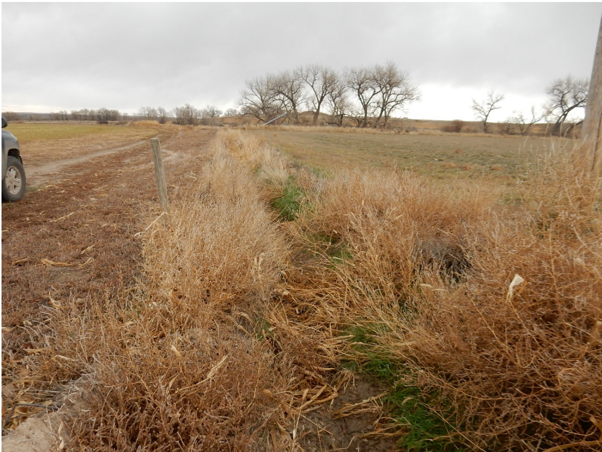
Figure 4.7. Earthen Ditch Located West of Peterson Draw.
