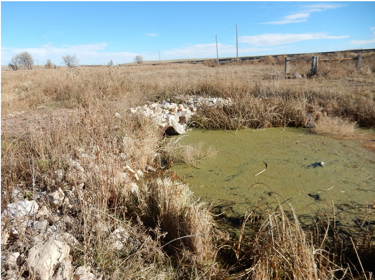
Figure 4.15. E B Wilson Ditch Diversion Structure on the Niobrara River.
