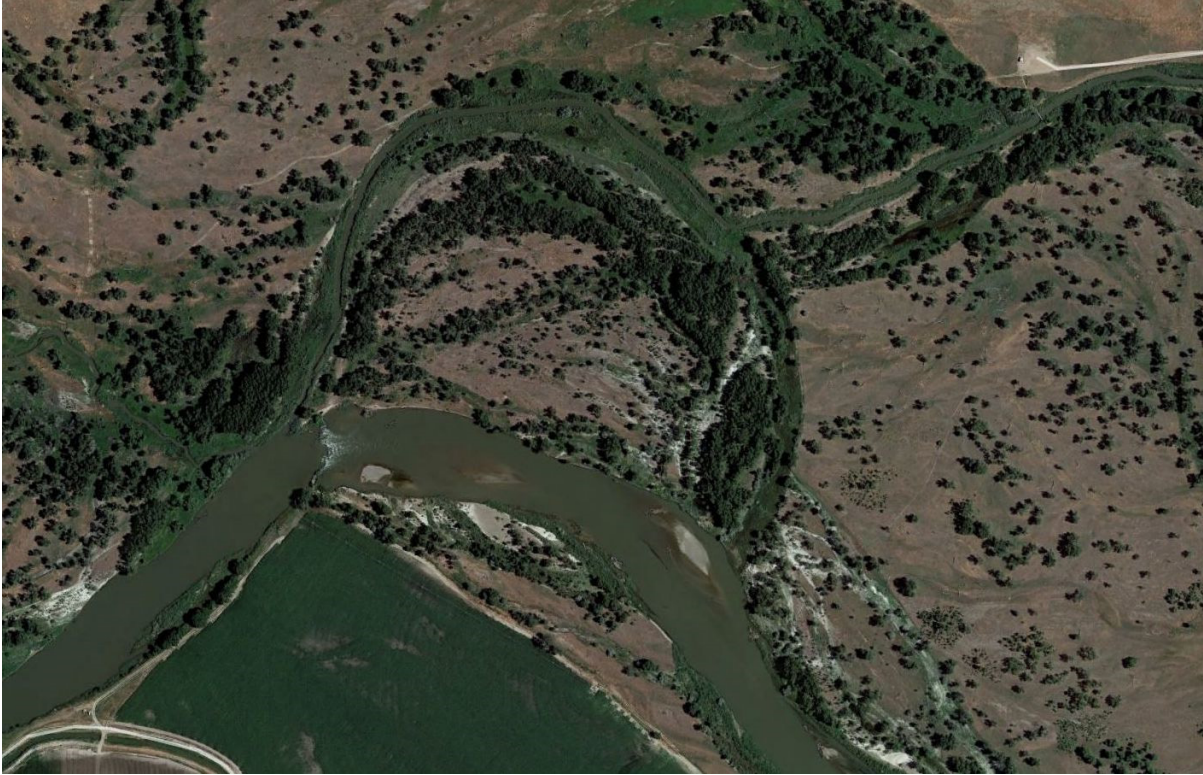
Figure 3.15. Rock Ranch Diversion Dam: North Platte River.
