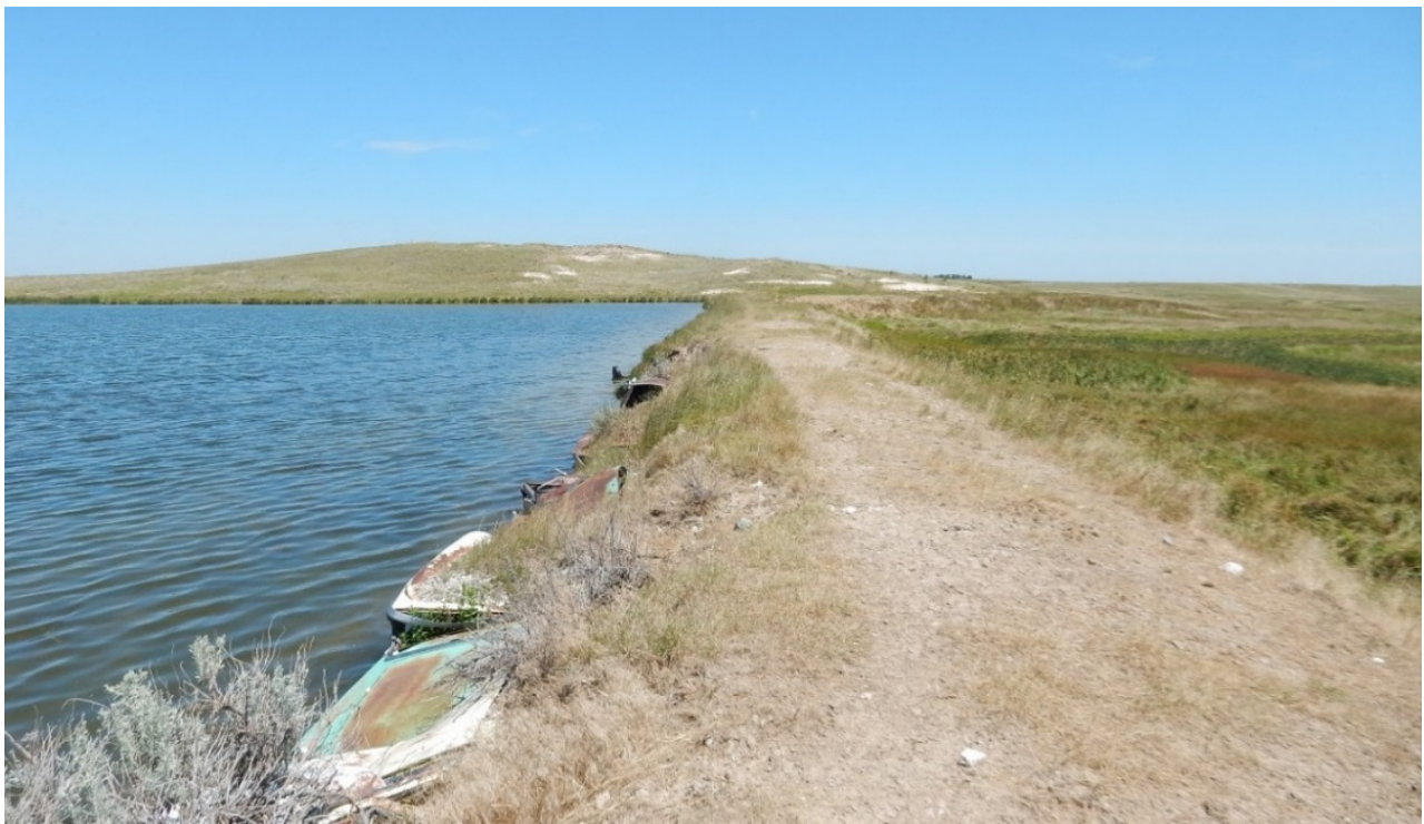
Figure 4.2. Top of Dam Embankment on Hoblit Reservoir.
