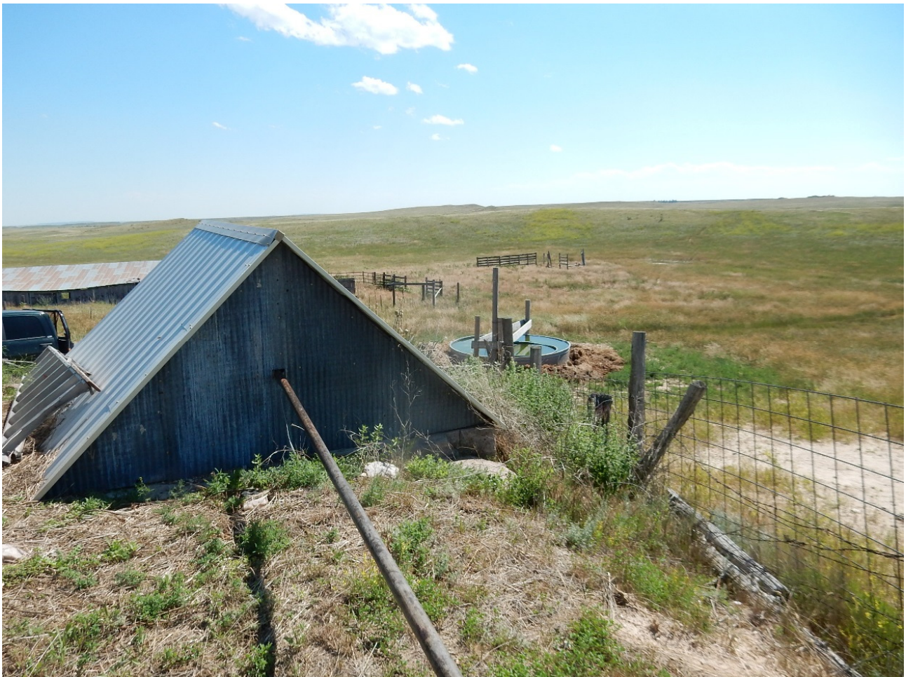
Figure 4.45. Existing Cistern Well and Stock Tank.
