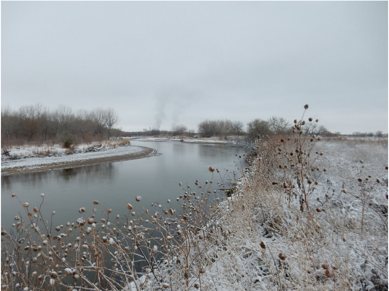
Figure 4.72. View of Channel Bank on the North Platte River at the C-03 Proposed Project Site.
