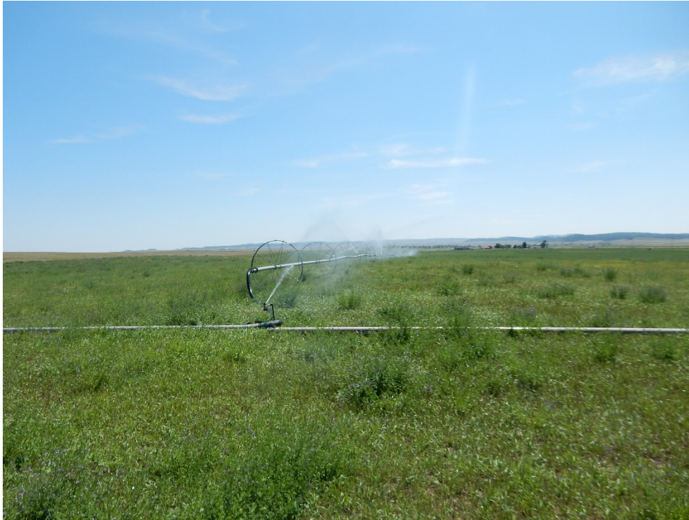
Figure 4.10. Existing Sideroll Sprinkler System Supplied by the Ladwig No. 2 Well.
