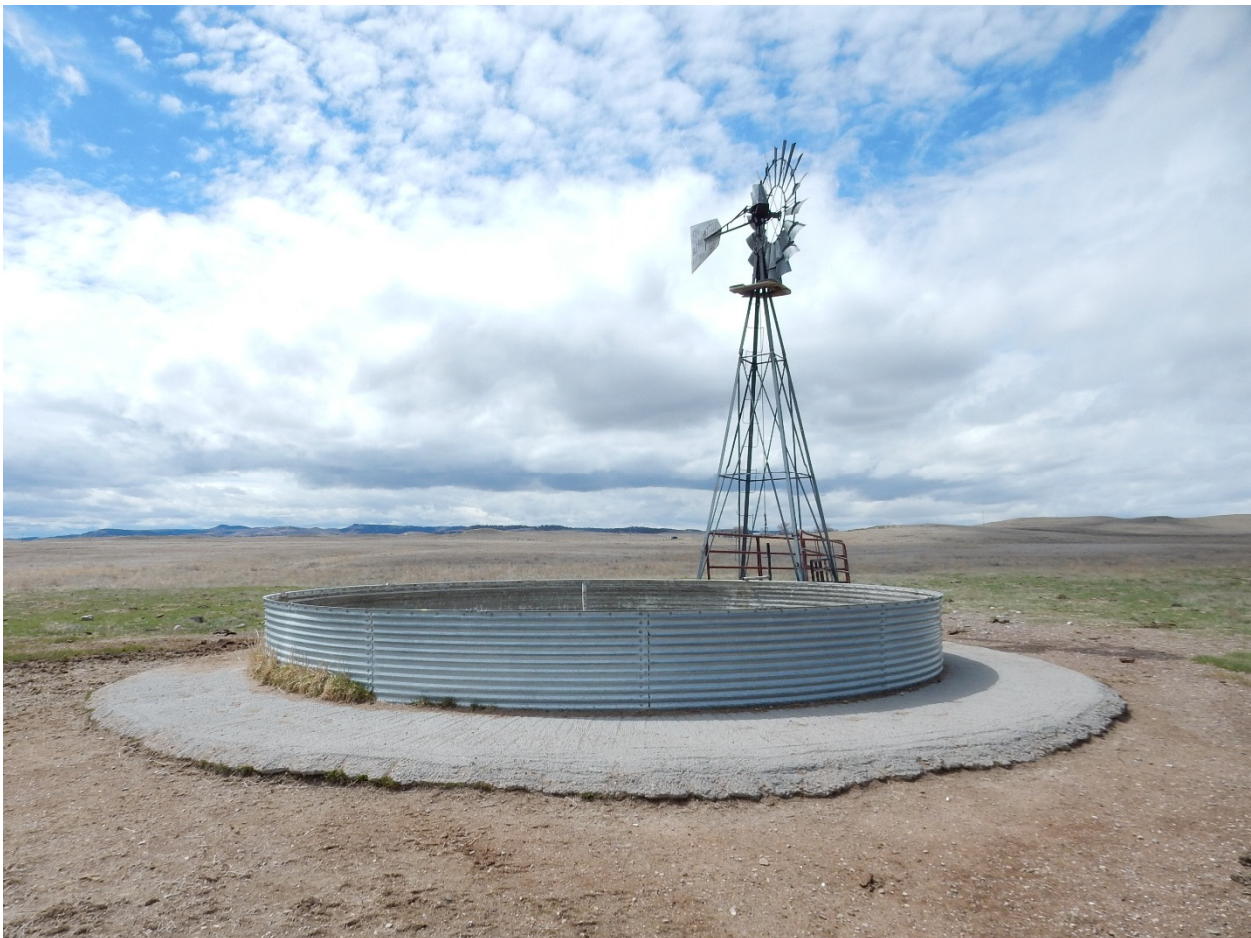
Figure 4.52. Existing Hoblit #3 Well and Stock Tank.
