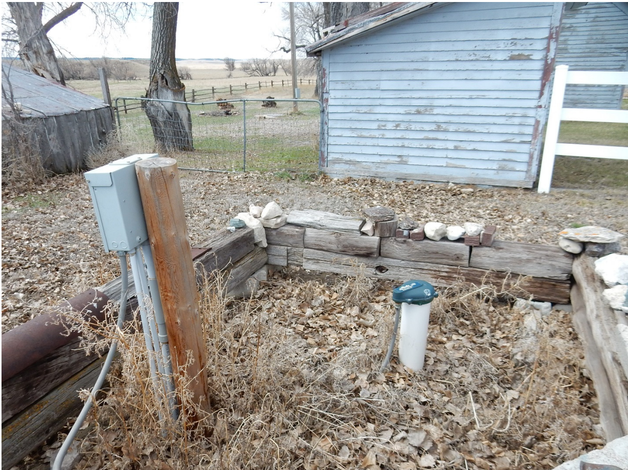
Figure 4.51. Existing Hoblit #5 Well and Stock Tank.
