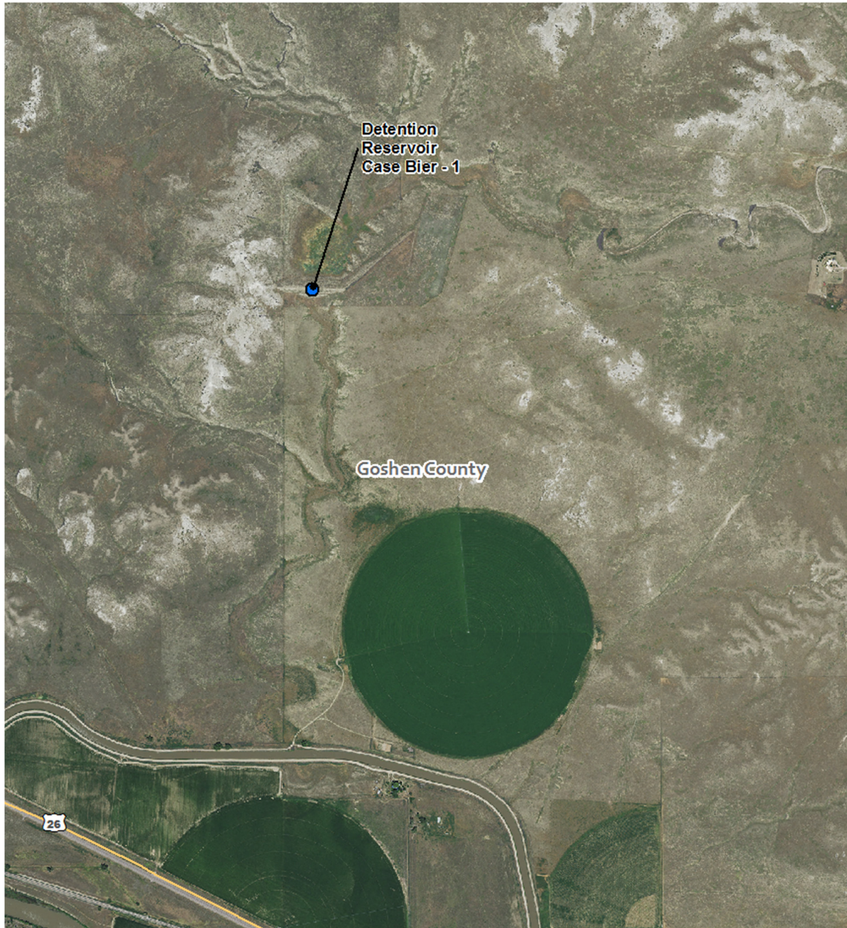
Figure 3.61. Detention Reservoir Case Bier – 1 Located North of Fort Laramie.
