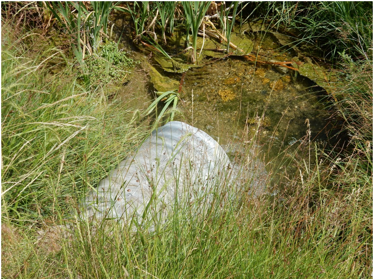
Figure 4.5. Headgate Structure on Hoblit Reservoir for the Emma Ditch.
