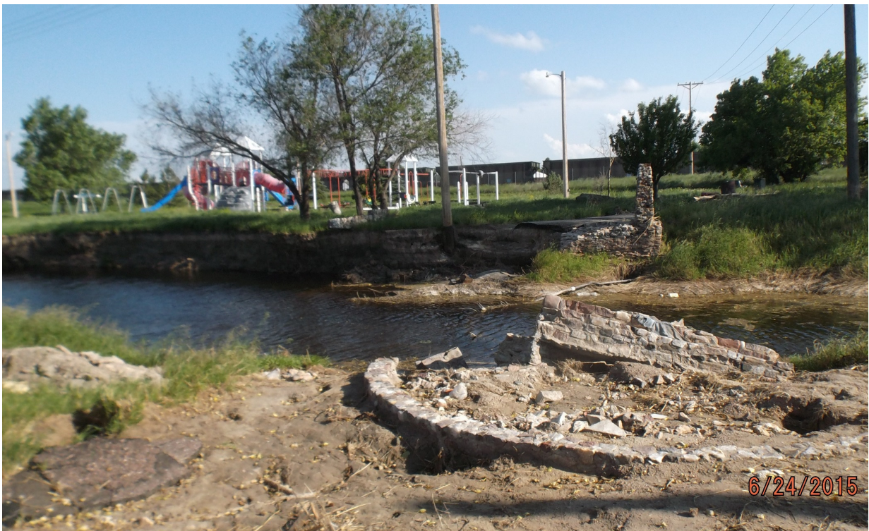
Figure 3.3. Niobrara River Flood at Lusk's Northside Park (Photograph by Niobrara Conservation District).
