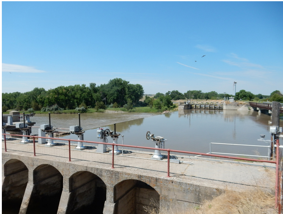
Figure 3.13. Whalen Diversion Dam: North Platte River.
