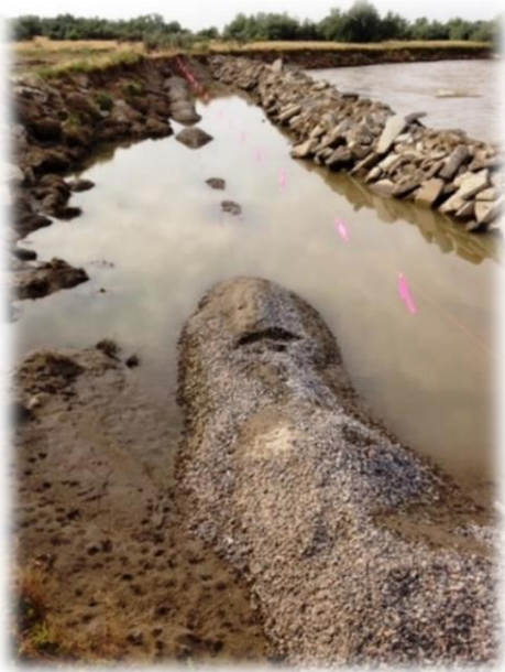
Figure 28: Exposed Worland sewer.
