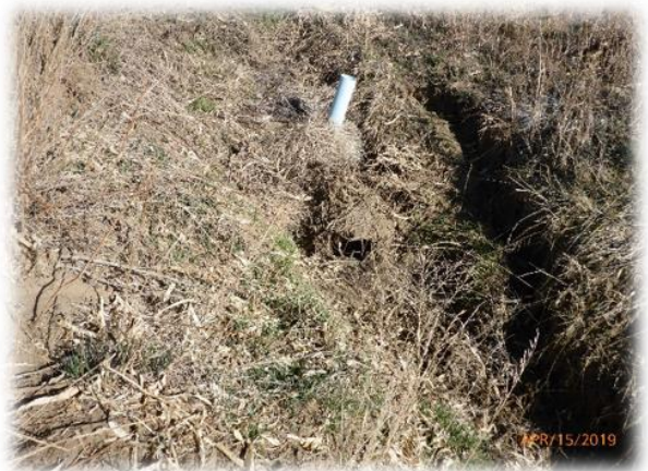
Figure 59: View of buried irrigation device.
