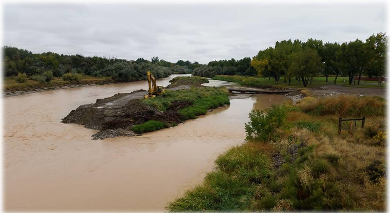
Figure 27: Removal of deposited silt island near Worland, WY. (Donnell & Allred, 2017)
