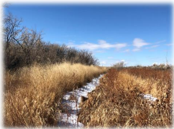
Figure 58: View of existing supply ditch off the Big Horn Canal near Manderson, WY.
