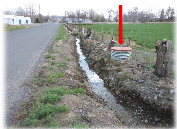
Figure 42: NADD ditch and access.
