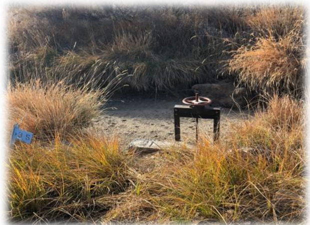
Figure 67: Representative view of headgate along the Big Horn Canal.
