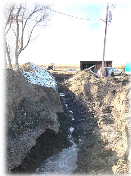
Figure 36: West River Road drainage project.
