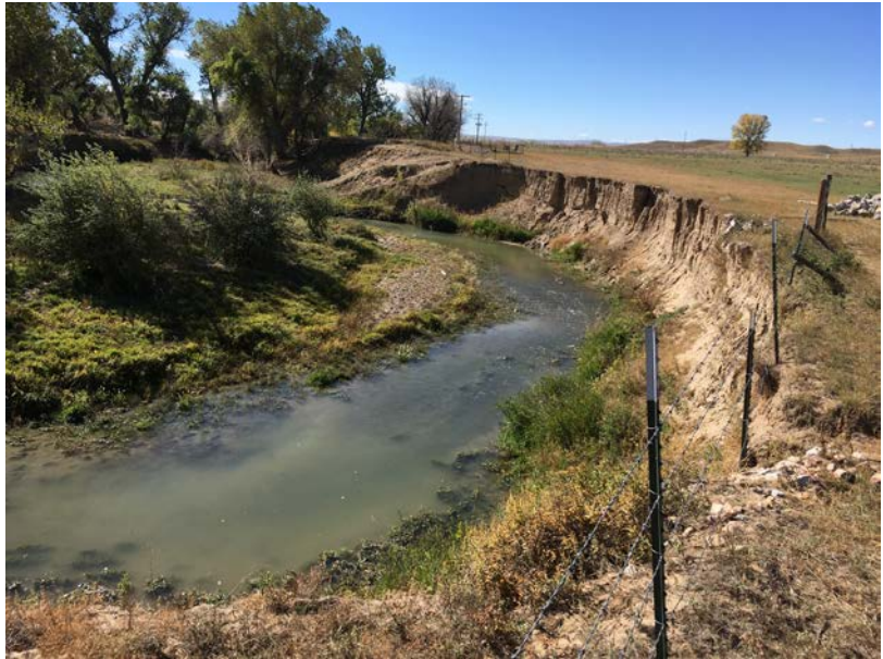
Figure 4.2-29. Bank Erosion on Lower Chugwater Creek.
