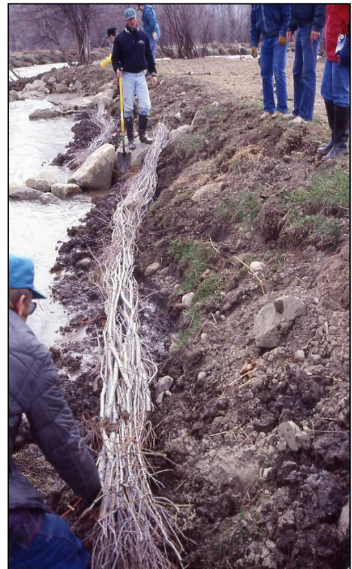
Figure 6.7-4 Stream Stabilization Measure: Willow Fascine Installation.
