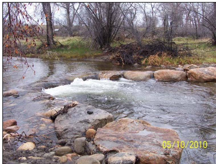
Figure 6.7-2 Stream Stabilization Structure: Rock Vortex Weir.
