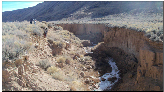
Figure 3.3-6 Inoperable Irrigation Headgate on Canyon Creek.
