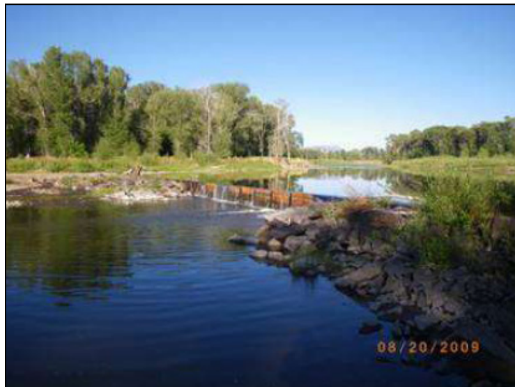
Figure 5.7-4 Sheet pile Diversion Structure: Little Snake River.
