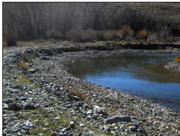
Figure 4.6-2 Example Channel Restricting Terrace Constructed at the Cobb Ranch Channel Restoration Project
