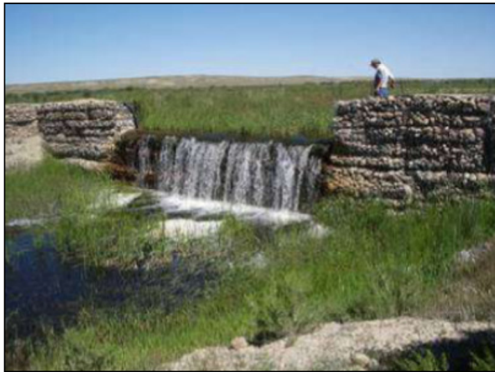
Figure 5.7-3 Gabion Gradient Control Structure: Muddy Creek.
