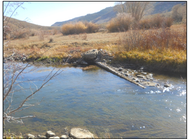
Figure 4.6-4 Flow Deflection Bank Stabilization on Cobb Ranch Section of Savery Creek
