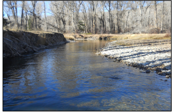
Figure 4.5-2 Savery Creek as Viewed Downstream from XS-03 Showing Evidence of Significant Bank Erosion of the Left Bank.
