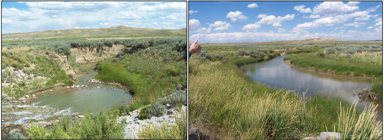
Figure 5.7-7 Channel Gradient Restoration Feature on Muddy Creek near Baggs, WY. Photo on left is viewed downstream from the dam at incised channel. Photo on the right is viewed upstream at restored gradient.
