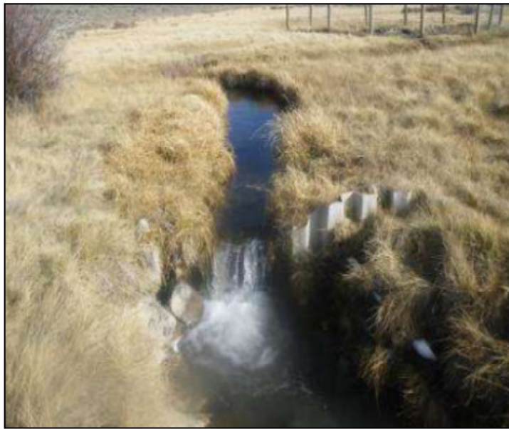
Figure 5.7-2 Typical Sheet pile Grade Control Structure on Upper Muddy Creek.
