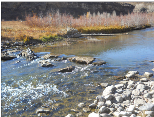
Figure 4.6-5 Typical Rock Vane Located on the Cobb Property
