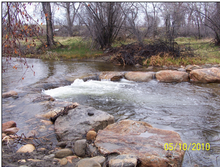
Figure 5.7-6 Stream Stabilization Structure: Rock Vortex Weir.
