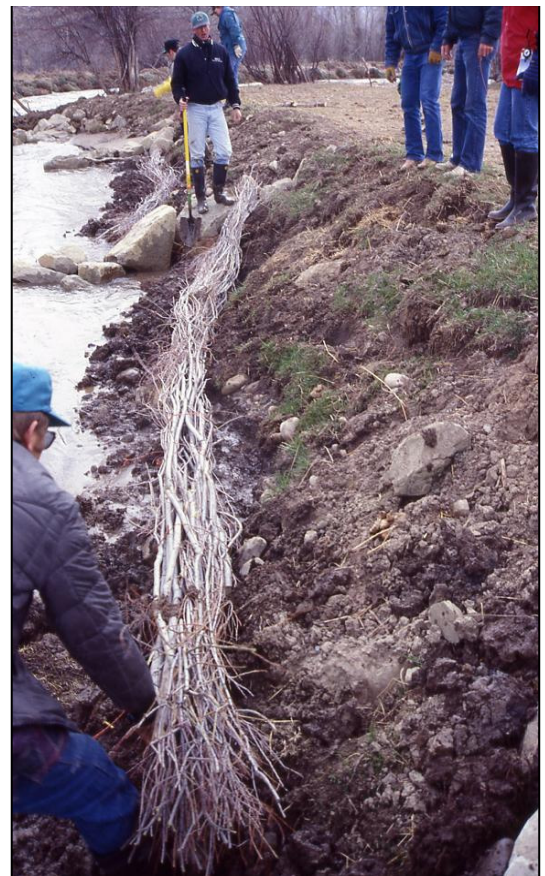
Figure 5.7-8 Stream Stabilization Measure: Willow Fascine Installation.
