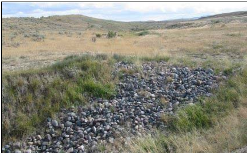
Photograph 15. Headcut with grading and rip-rap on a tributary to Kirby Creek.
