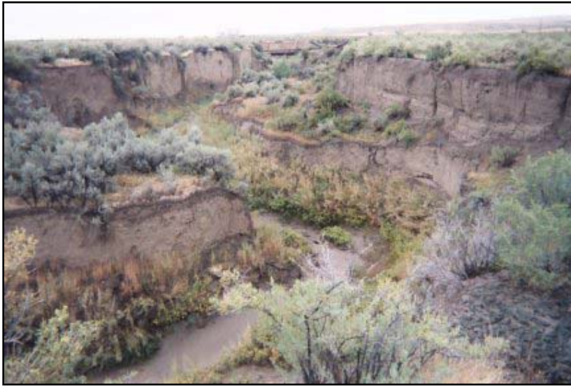
Photograph 7. View looking downstream at Kirby Creek incising itself upstream from the Red Hole Road. The bridge is visible as the dark object in the upper center of the photo. This stream is a Rosgen Type E.
