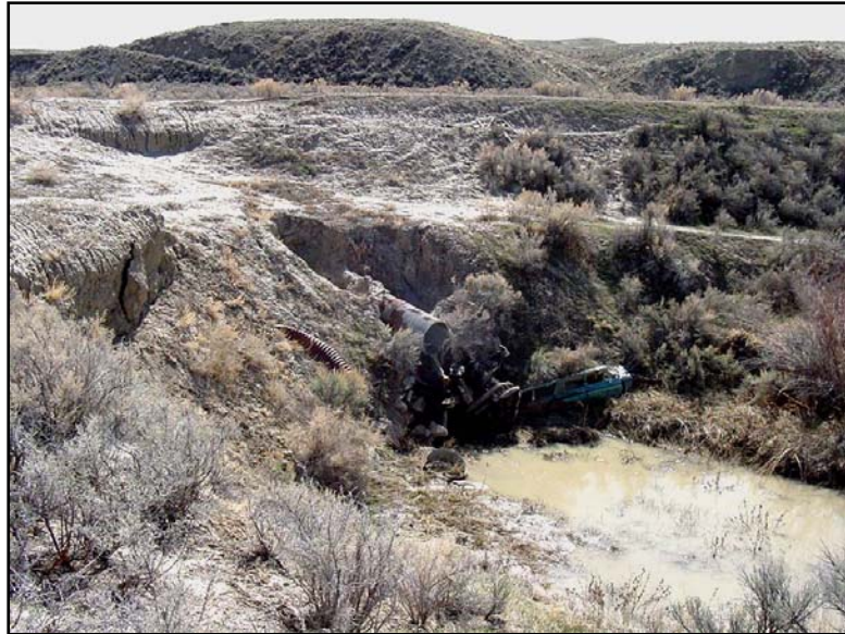
Photograph 18. Spillway of the Jones Dam
