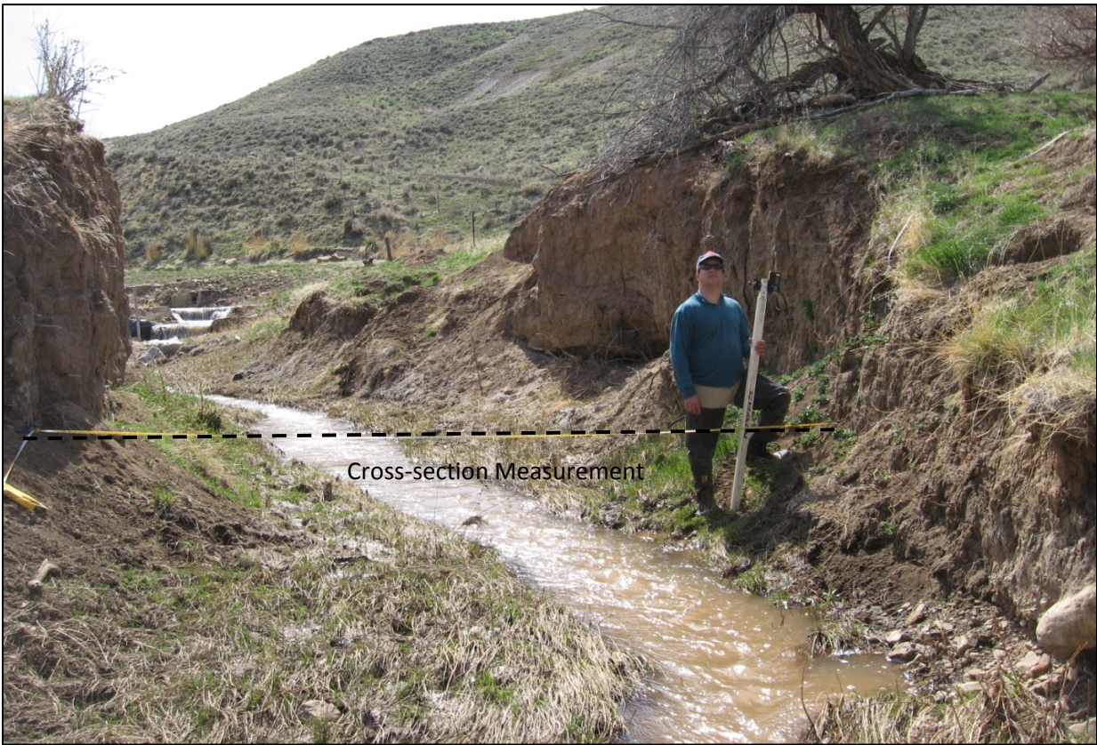
Figure 3.41. Overview of Terasen Stream Stabilization Cross-Section Downstream of Restoration Project.
