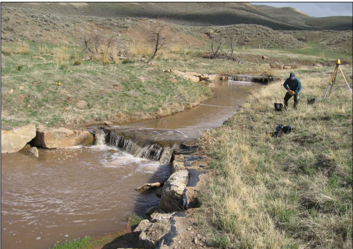
Figure 3.39. Terasen Stream Stabilization Project Overview.
