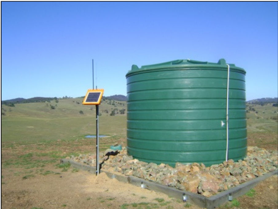
Figure G.5. Typical solar pump with storage tank configuration (Observant 2010).
