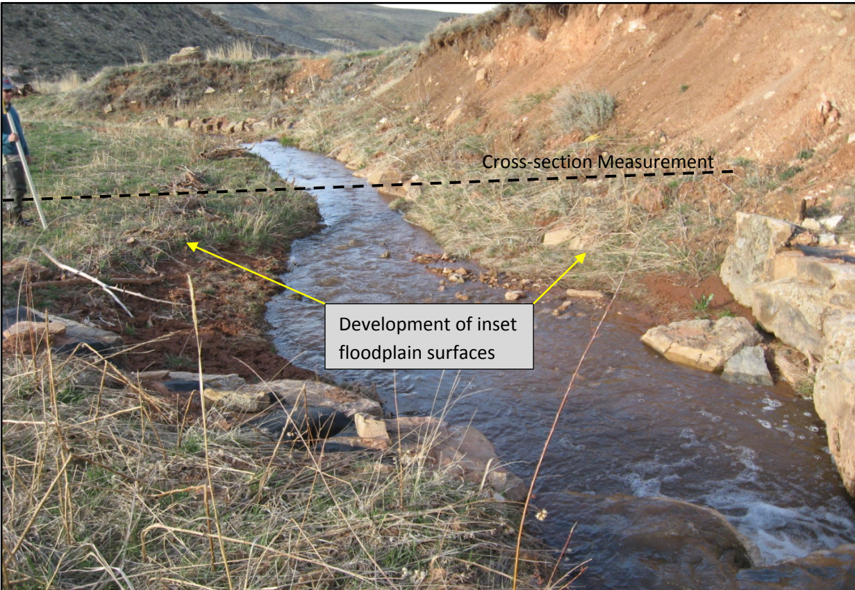
Figure 3.38. Overview of West Kirby Grade Stabilization Cross-Section within Restored Channel.
