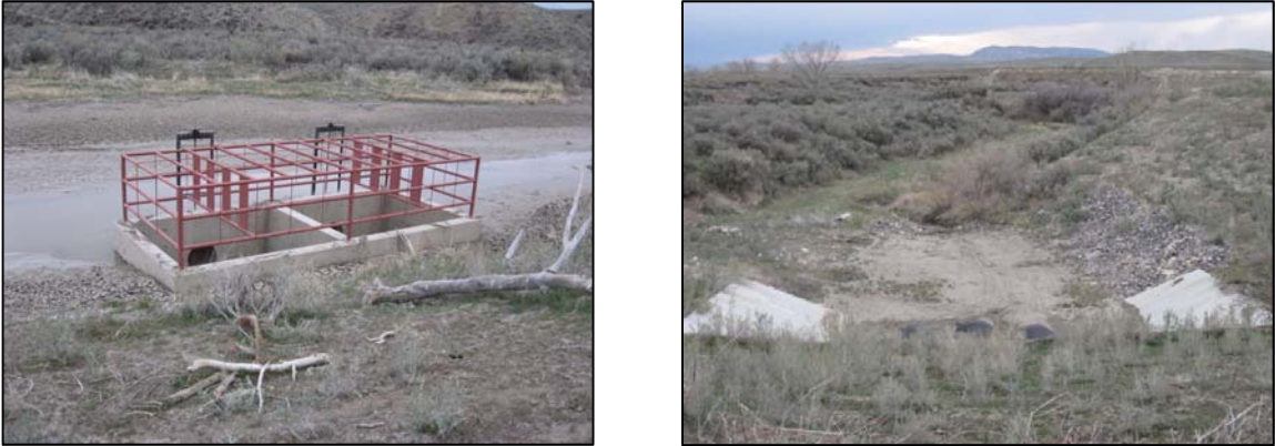
Figure 3.55. Jones Dam Outlet Structure (left), and emergency spillway (right).
