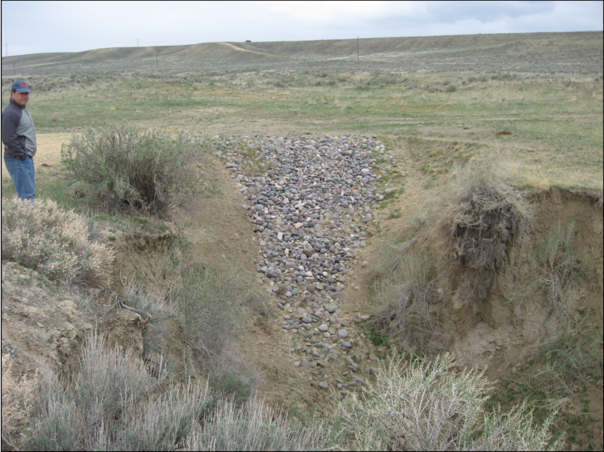
Figure 4.40. Headcut Stabilization with Large Cobbles in a Tributary to Kirby Creek.
