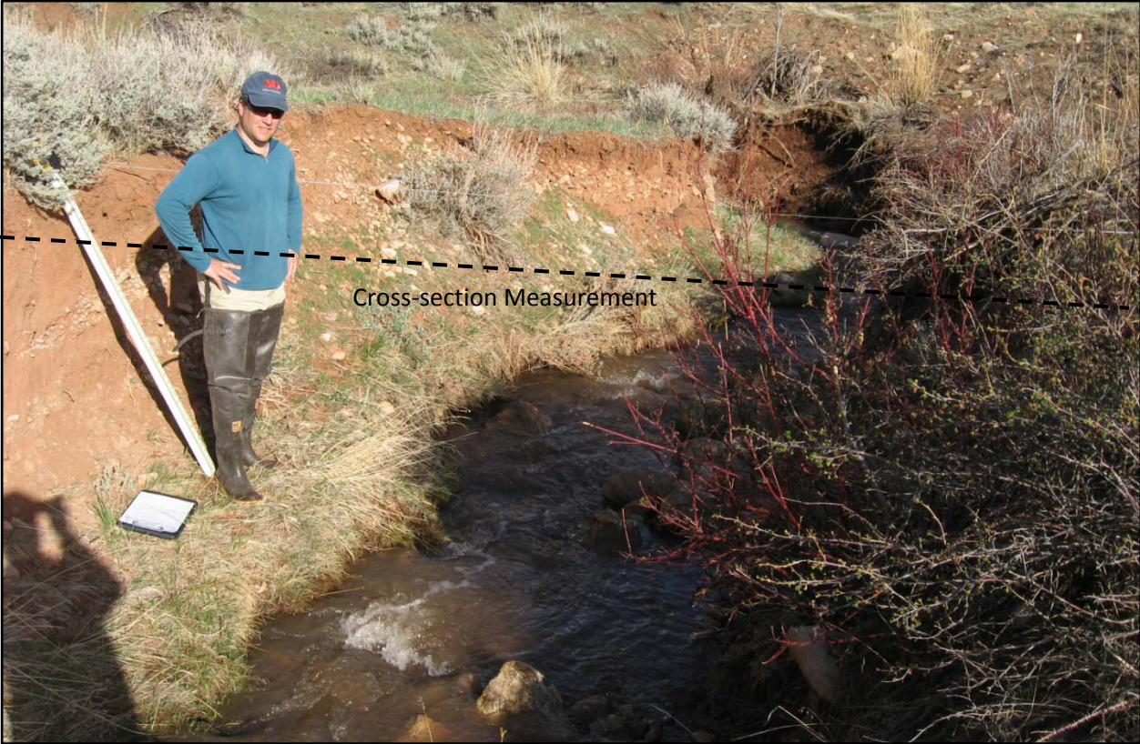
Figure 3.36. Overview of West Kirby Grade Stabilization Cross-Section Downstream of Restoration Project.
