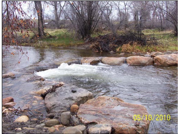
Figure 6.7-2 Stream Stabilization Structure: Rock Vortex Weir.
