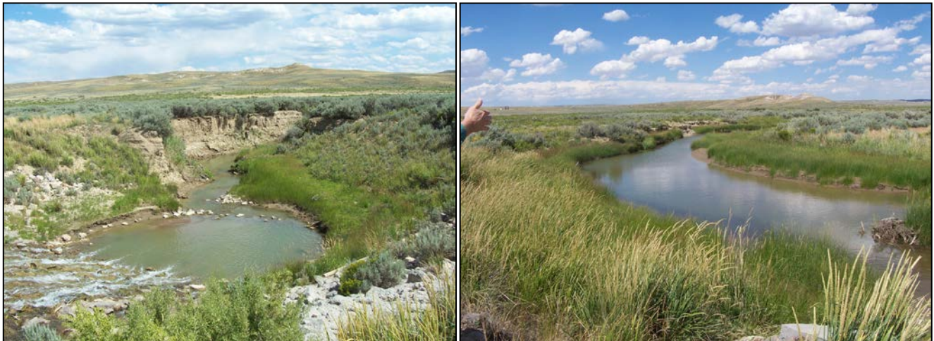
Figure 6.7-3 Channel Gradient Restoration Feature on Muddy Creek near Baggs, WY. Photo on left is viewed Downstream from the Dam at Incised Channel. Photo on the right is viewed Upstream at Restored Gradient.
