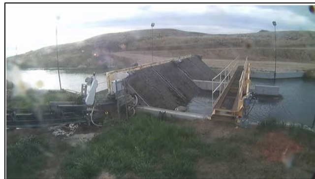
Figure 6.9-3. Self-cleaning weed screen device at Heart Mountain Irrigation District.
