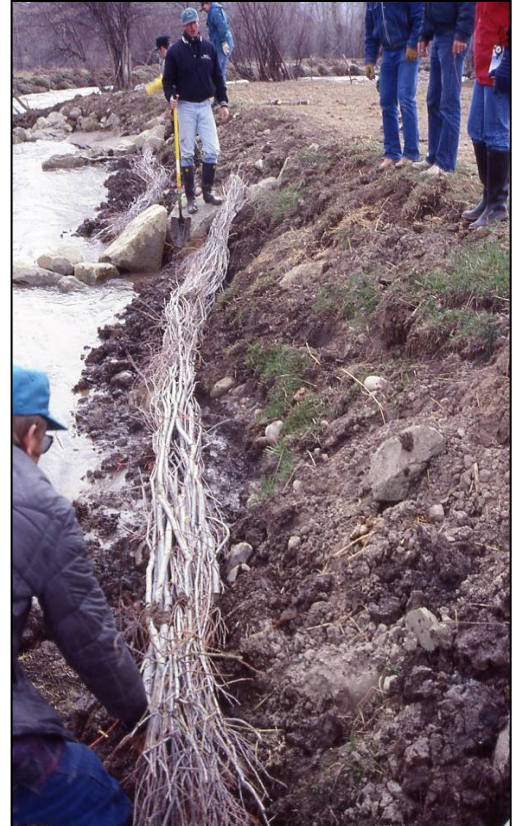
Figure 6.7-4 Stream Stabilization Measure: Willow Fascine Installation.
