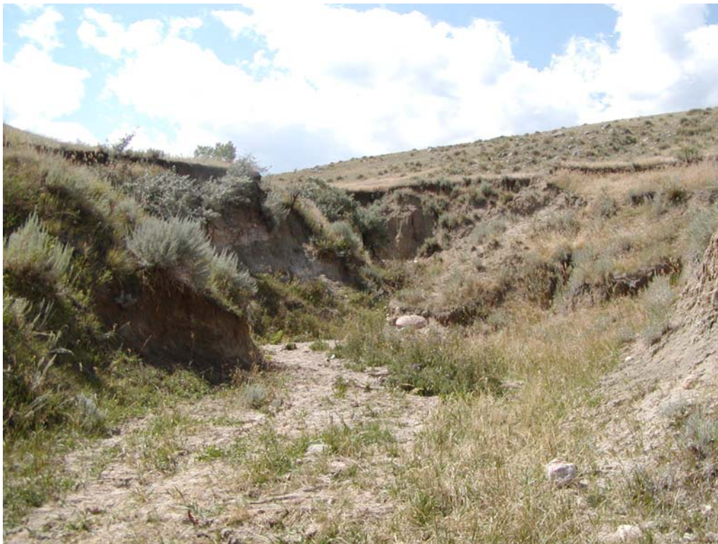
Site No. 1 – Moeller supply ditch upstream of reservoir – erosion
