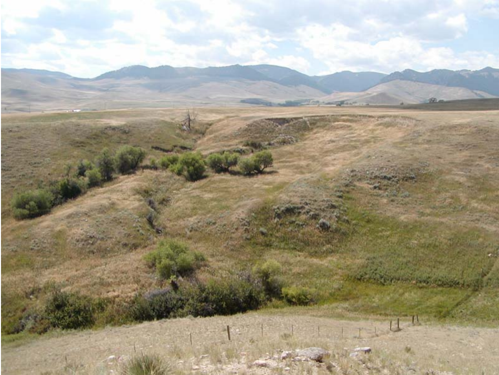
Site No. 1 – Slump upstream of right abutment
