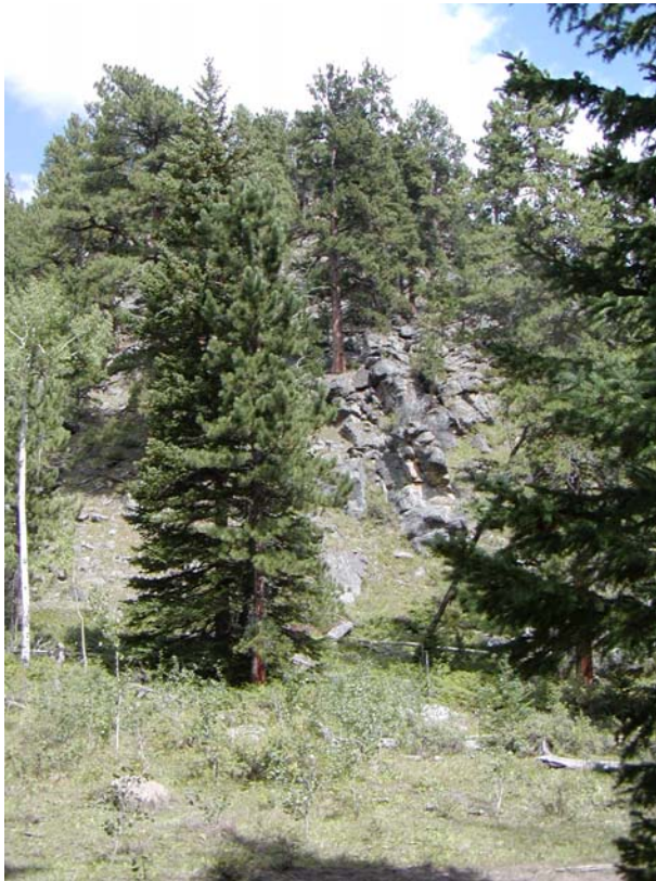
Site No. 4 – Left abutment
