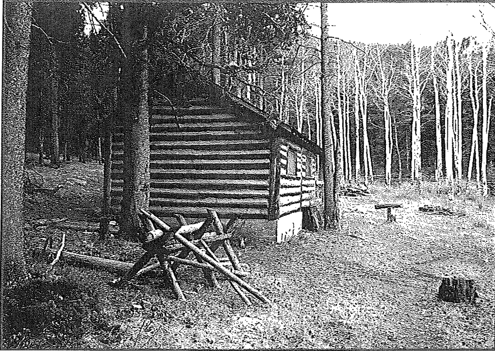
Rear of cabin viewed westward.
