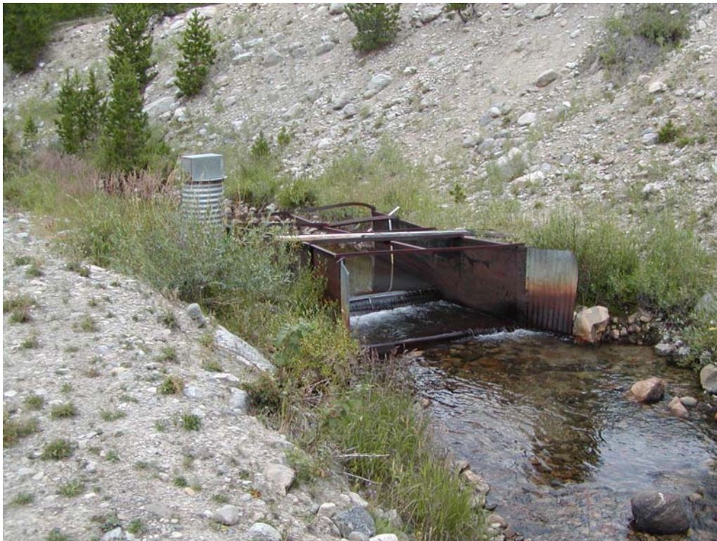
4 Lakes and French Creek Diversion – Flume
