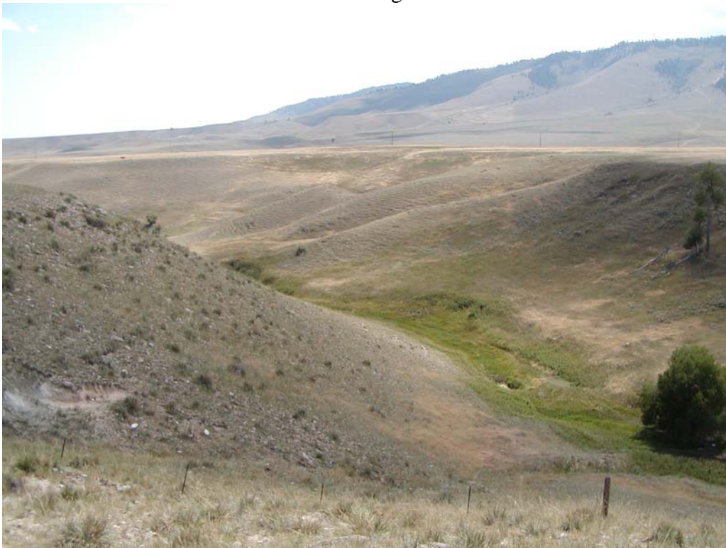
Site No. 1 – Left abutment (left foreground), right abutment (right side)
