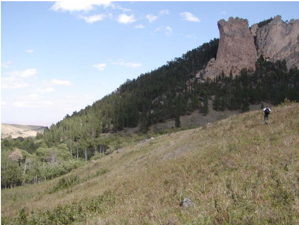
Site No. 3 – Right abutment (background)
