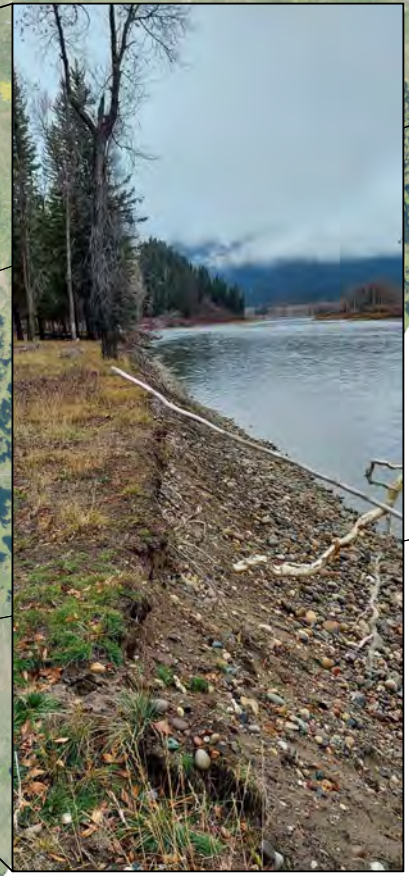
PIC 2: LOOKING UPSTREAM
