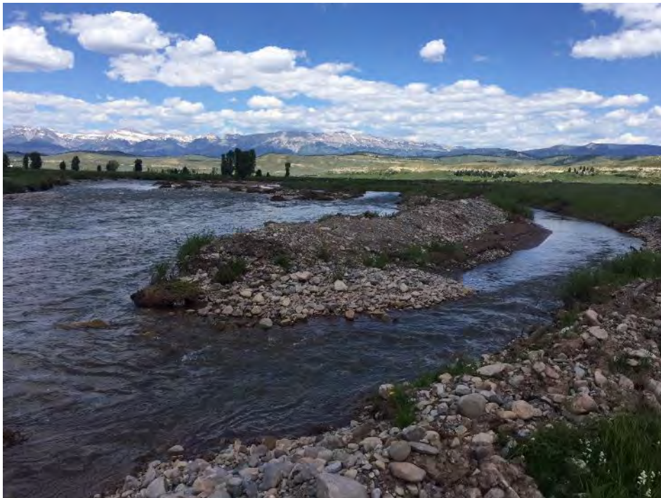
Photo 2: The lower gravel push-up dam location that is no longer in use as a result of Phase 1 project activities. Note the disturbance in the foreground and background resulting from heavy equipment instream.
