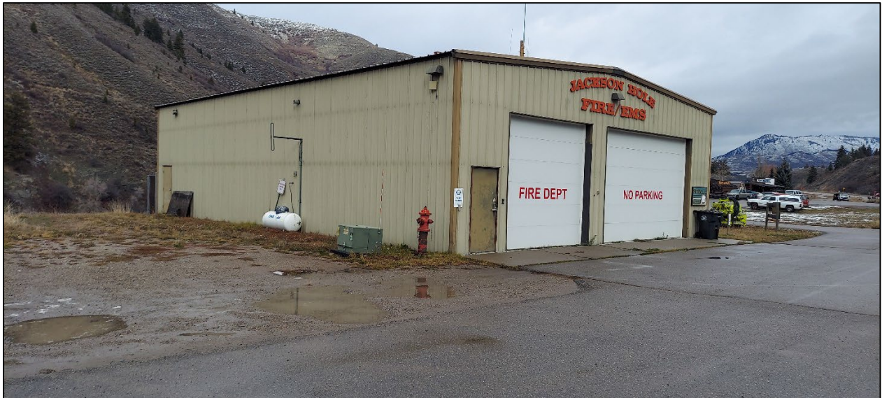
Figure 70: Hoback Fire Station – Fire Suppression Rehab (Project ID: 10.1)
