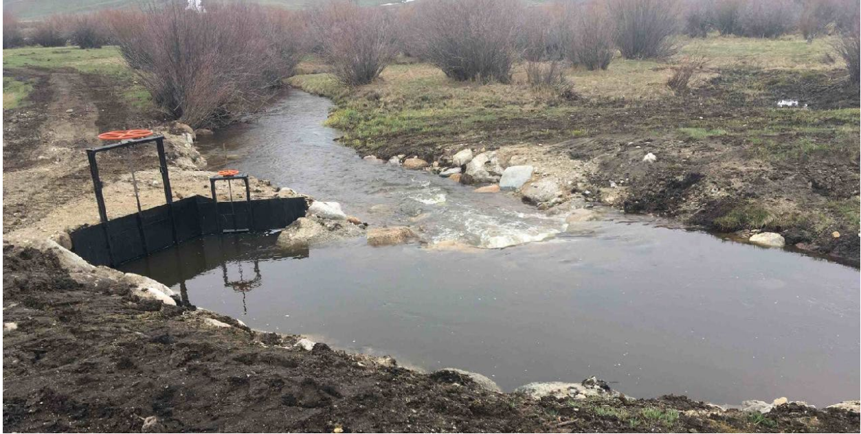
Example 5: Diversion structure and headgate rehabilitation project (New Fork River Watershed Study)
