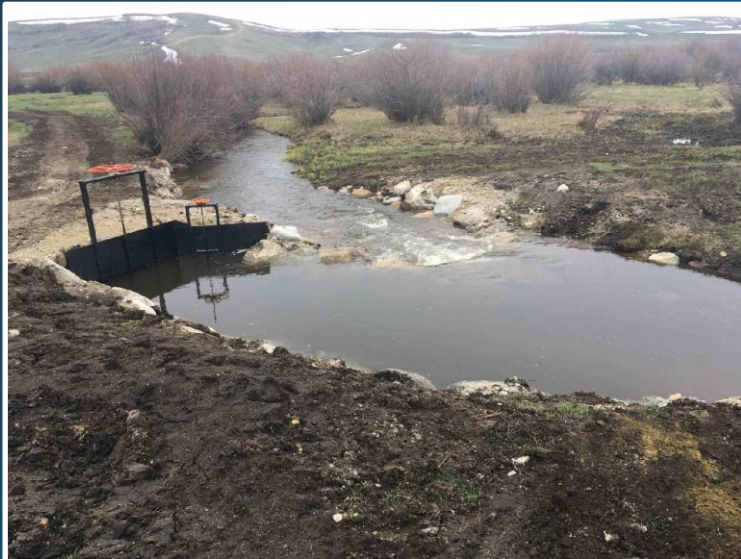
DIVERSION / IRRIGATION REHAB
