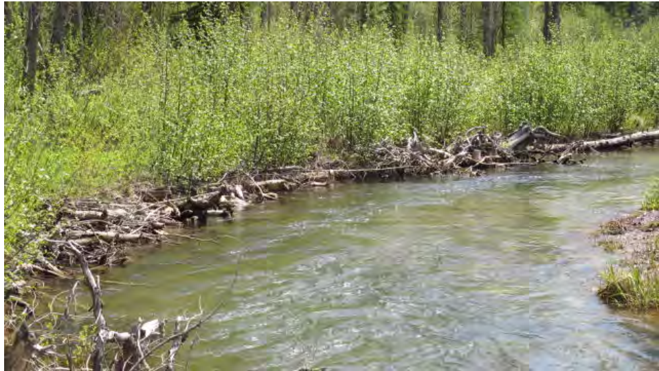
Photo 8: Brush bank structure 2 years post-treatment, Ninemile Creek, MT.
