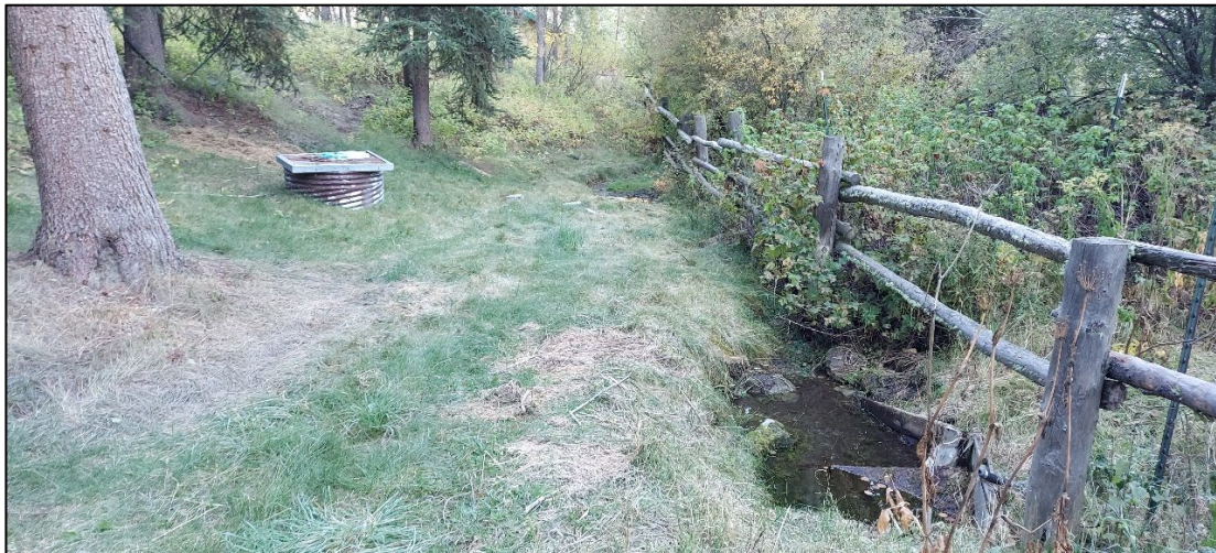
Figure 66: Rode No. 1 Well and Stock Tank Project (Project ID: 11.1)
