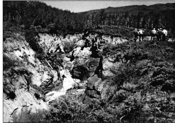
Figure 3.8 Wiant Ditch Washout (Reach 3).
