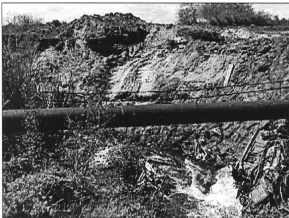
Figure 3.11 Ryan Foreman Pipe Crossing Over Wiant Ditch.
