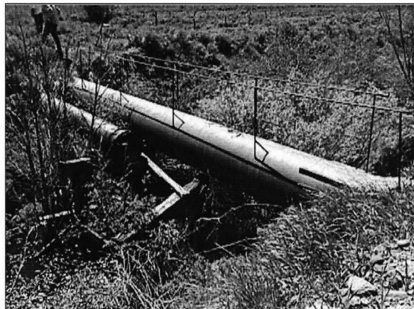
Figure 3.9 Gross Ditch Pipe Crossing Over Wiant Ditch.
