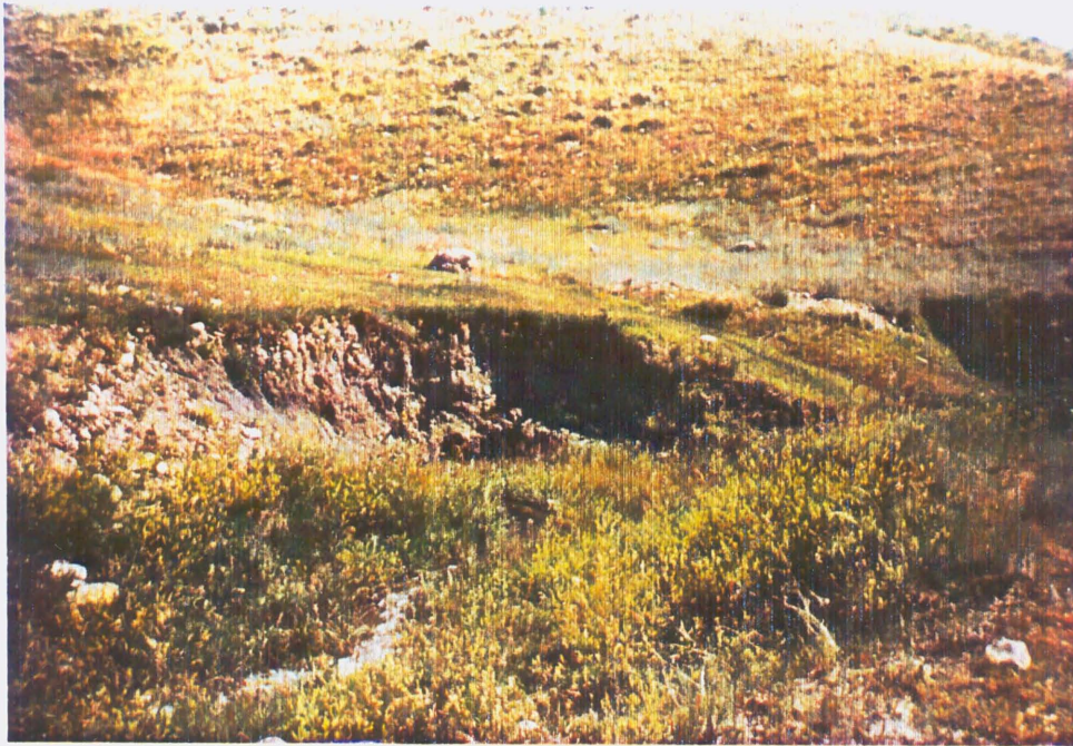
EROSION: 41 RANCH BAUER DITCH PROJECT NO. 6 - STA 61+46 THRU 64+05
