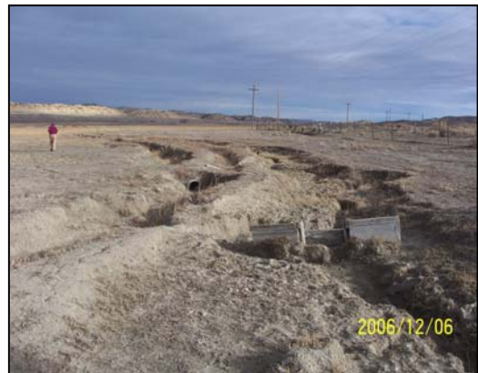
Figure 2.5-7 Parallel Ditches on Little John Ditch
