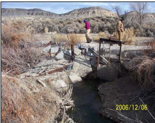
Figure 2.5-6 Little John Ditch Diversion
