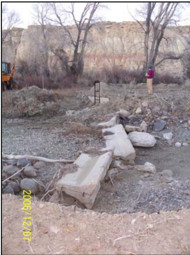
Figure 2.5-10 Wilson Ditch Diversion
