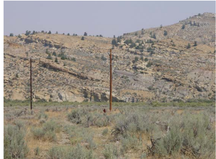
Close-up of left abutment; note bedded sedimentary sequence; note power line and oil pipeline markers in middle ground
