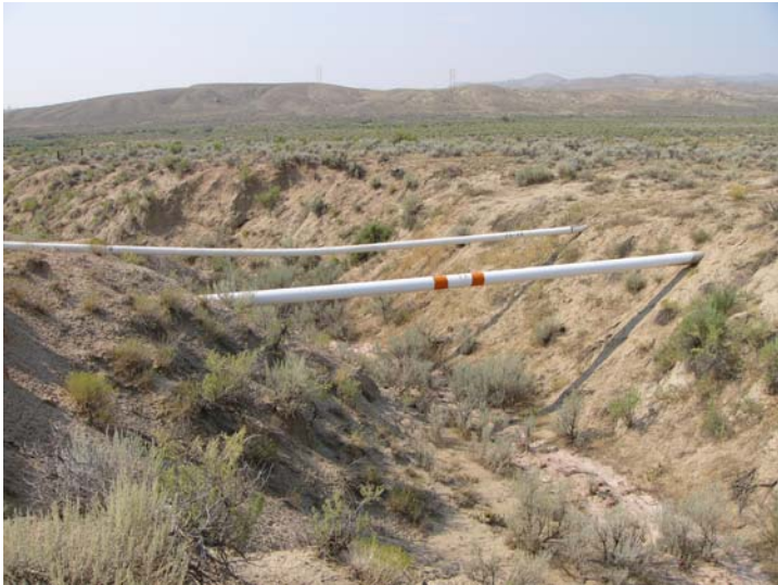
Oil pipelines in corridor passing through reservoir area; photo taken northwest of reservoir site
