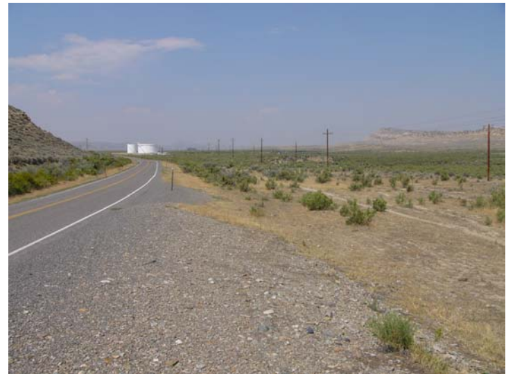
View of upper reservoir area; note oil storage tanks (and buried pipeline), highway, power line and telephone line are within inundated area
