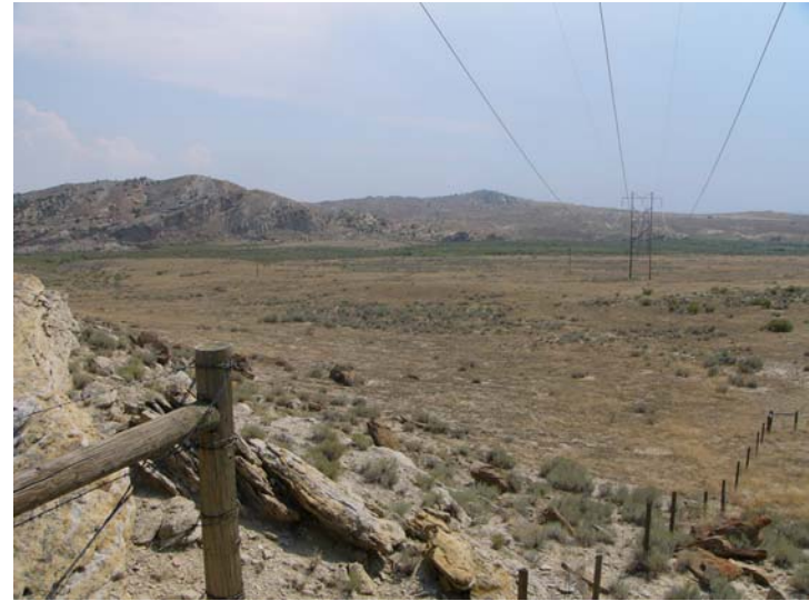
Right abutment and valley section; note transmission line; view looking upstream
