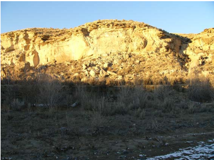
View of left abutment
