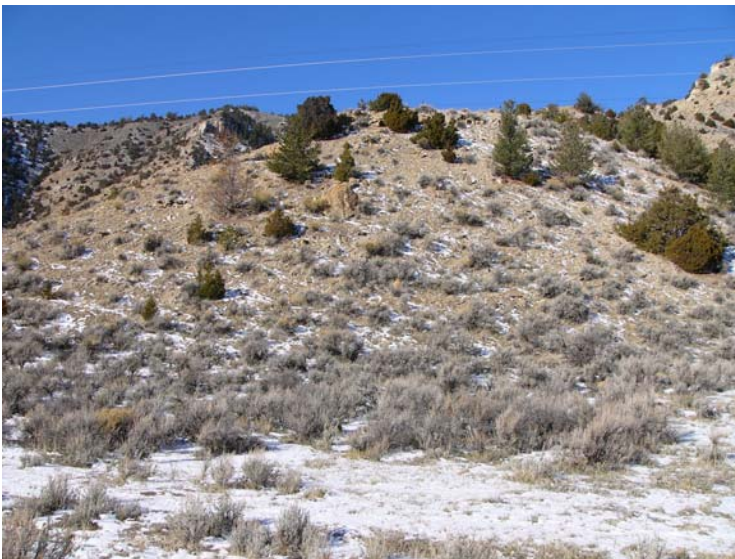
Close-up of left abutment
