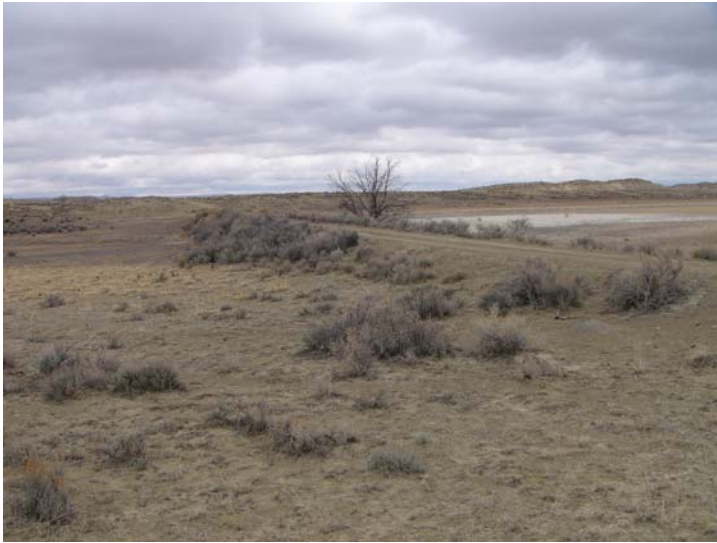
Existing Wales Reservoir Dam
