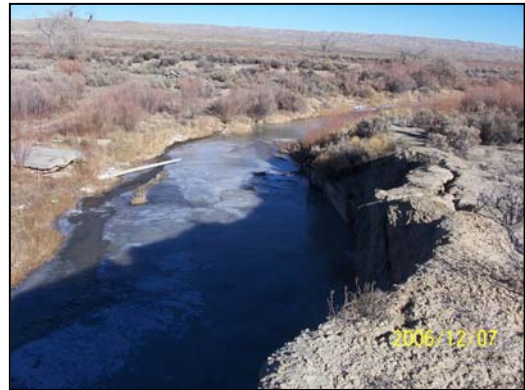
Figure 2.5-5 Kirby Ditch Diversion
