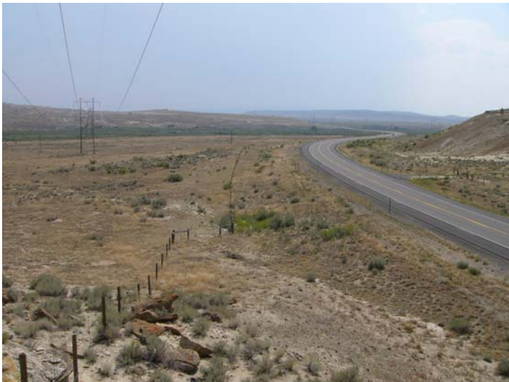
Left abutment; note Highway 120; view looking upstream
