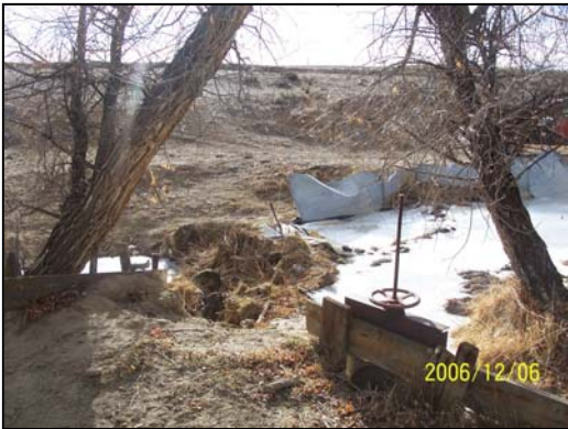
Figure 2.5-4 Hillberry North Headgate
