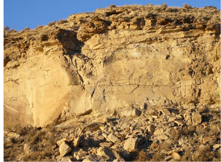
Close-up of thick-bedded sandstone in right abutment
