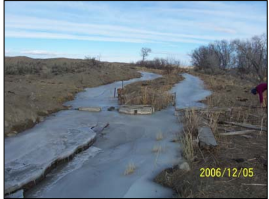
Figure 2.5-3 Splitter Structure in Caledonia Ditch
