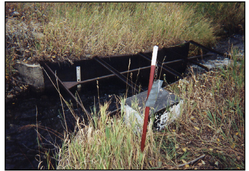
Six Mile flume
