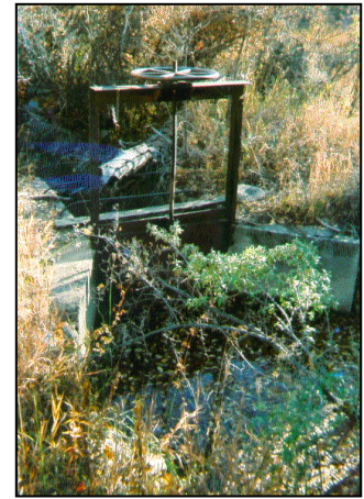
Hallie Ditch headgate
