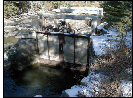
Rock Creek & South Piney headgate
