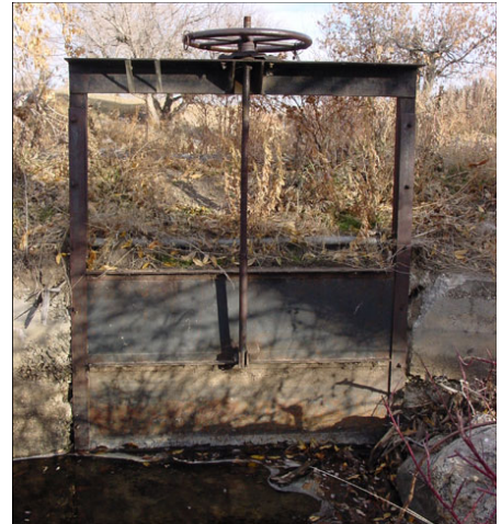
Hopkins Ditch headgate
