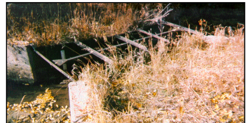
Penrose Ditch at Johnson Creek flume
