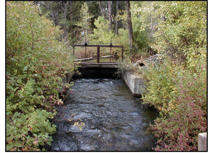
Prairie Dog , Primary Diversion headgate
