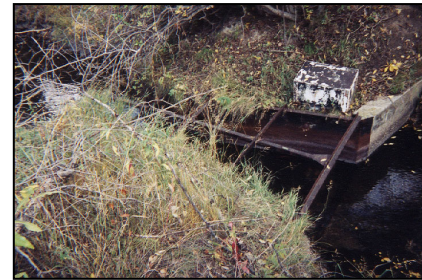
Clear Creek Land & Ditch Co. flume
