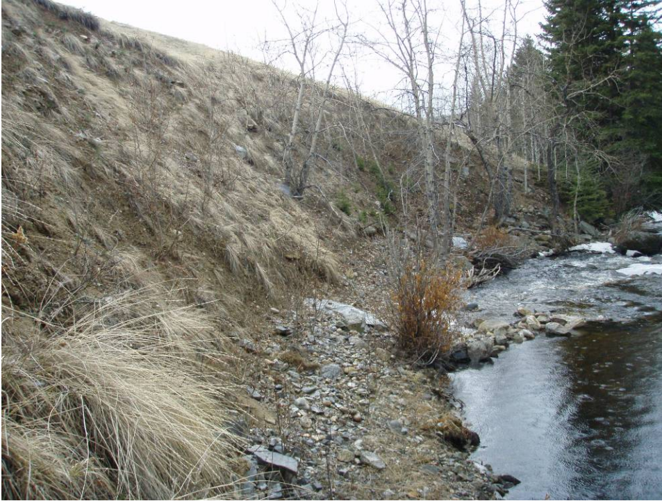
Photograph 10: Dam centerline at valley bottom looking downstream at thick alluvium.
