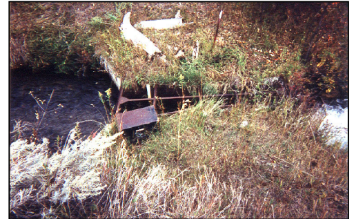
Crown Ditch Flume
