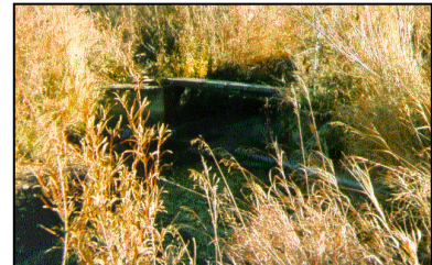
Mowry Basin flume
