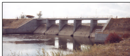
Healy Reservoir diversion dam
