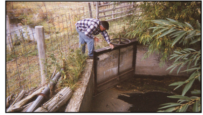
Dunlap Ditch Headgate
