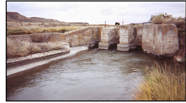
Pratt & Ferris No. 2 diversion structure
