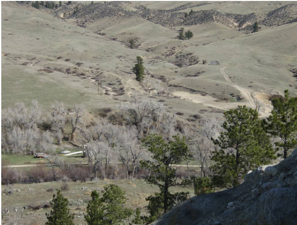
Photograph 4: Right abutment looking at the left abutment.
