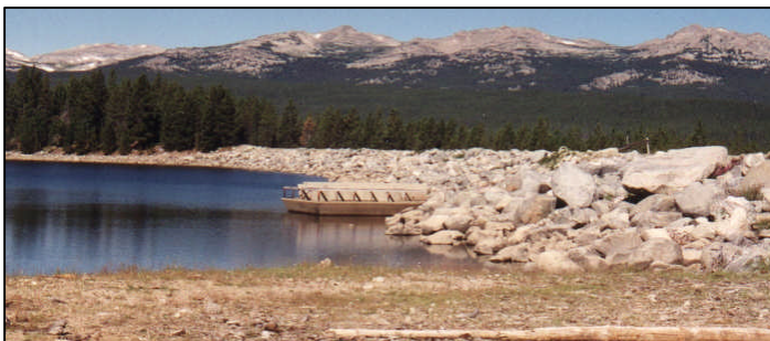
Willow Park Reservoir's upstream dam face and outlet structure
