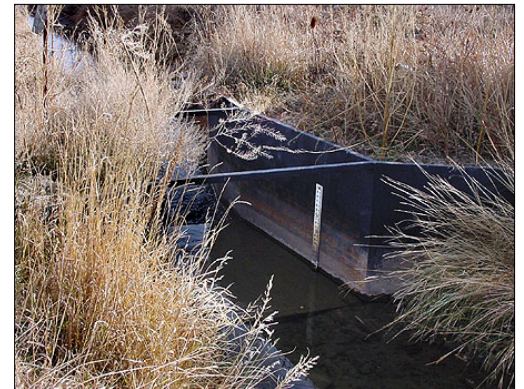
Prince Albert Ditch flume
