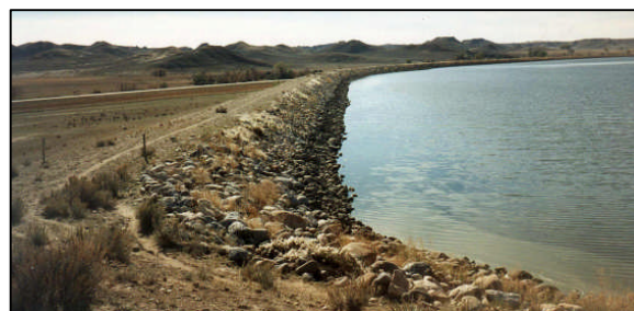
Healy Reservoir dam
