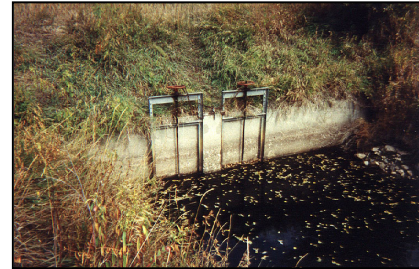
Clear Creek Land & Ditch Co. headgate
