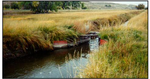
Roberts Ditch flume
