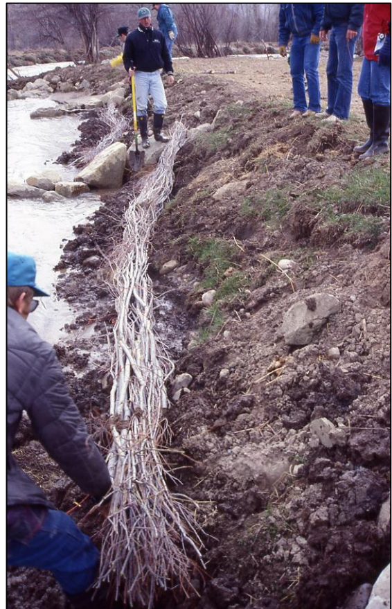
Figure 4.35 Stream Stabilization Measure: Willow Fascine Installation.
