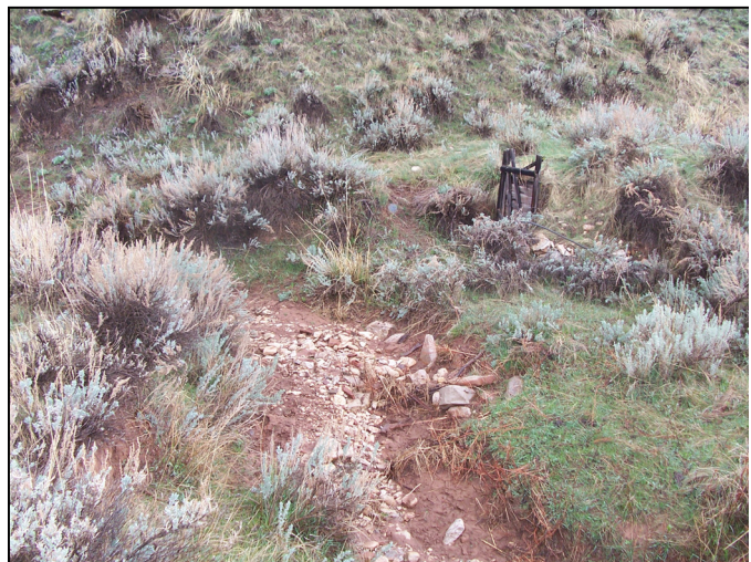
Figure 3.7 Inoperable Irrigation Headgate on Buffalo Creek.
