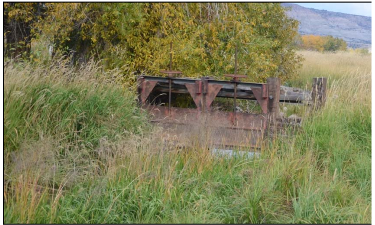
Figure 3.2-10 Nelson Ditch Headgate.
