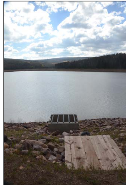
Figure 3.5-3. Beaver Meadows Reservoir Outlet Structure.
