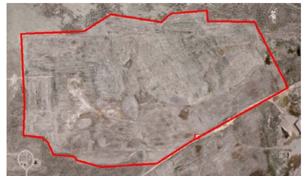
Figure 2.2-9 WDEQ Abandoned Sand/Gravel mine near Granger WY (Phase III Study Area).
