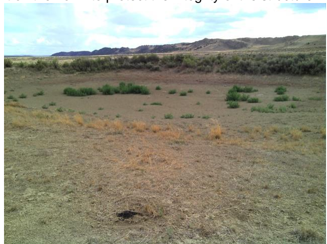
View of pond looking downstream at embankment
