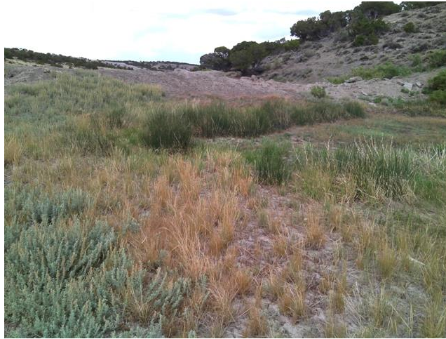
Uppermost pond with un-compacted embankment
