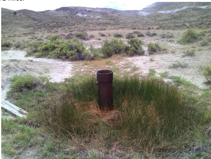
Well with overflow to pond (non-functioning)
