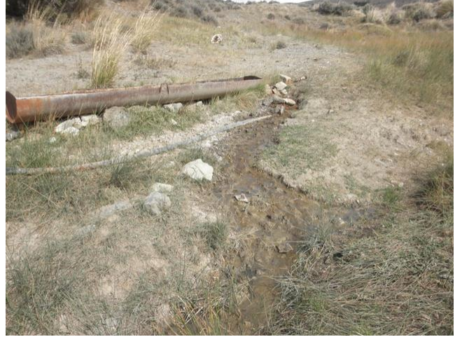
Outlet of spring development looking up toward collection box
