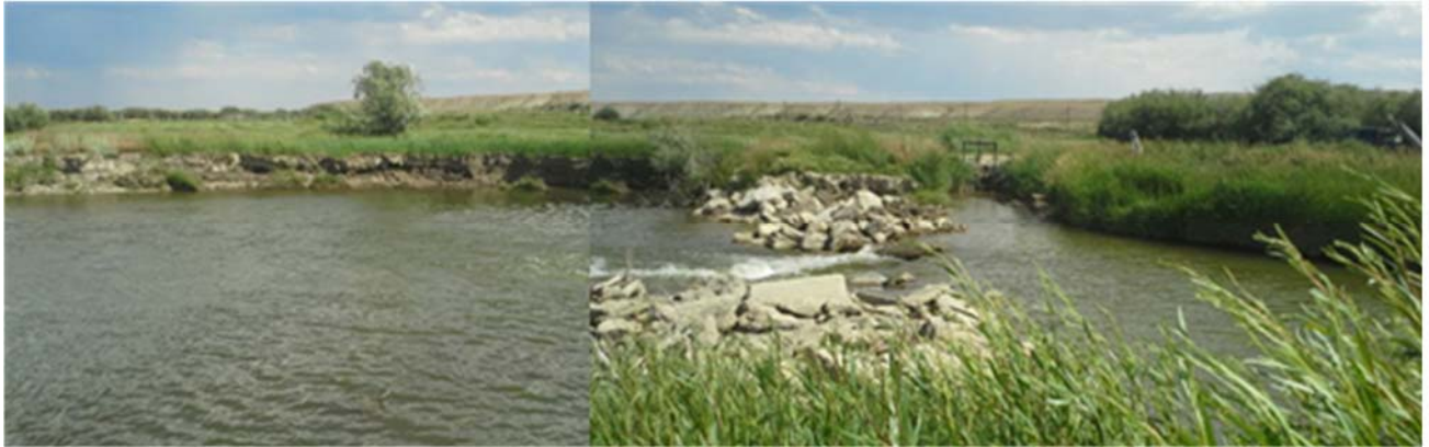
Figure 3.2-2 Christman #1 and Christman #2 diversion facility, Hams Fork River.
