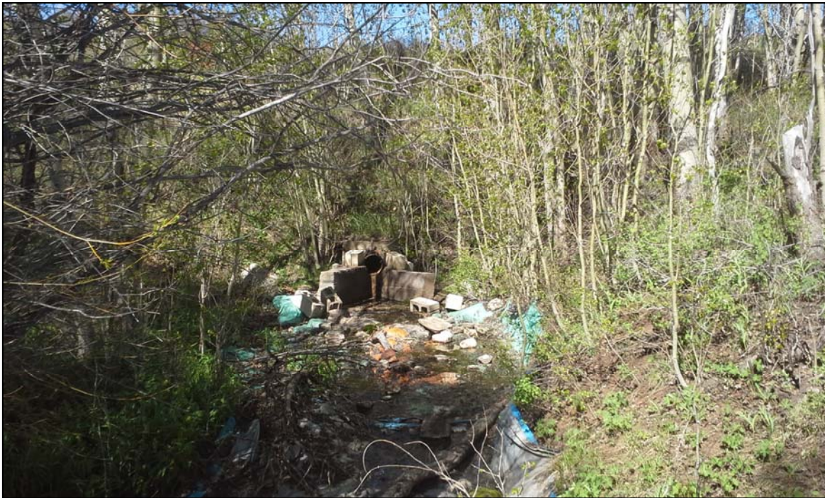
Figure 3.5-6 Davis No. 2 Reservoir outlet.
