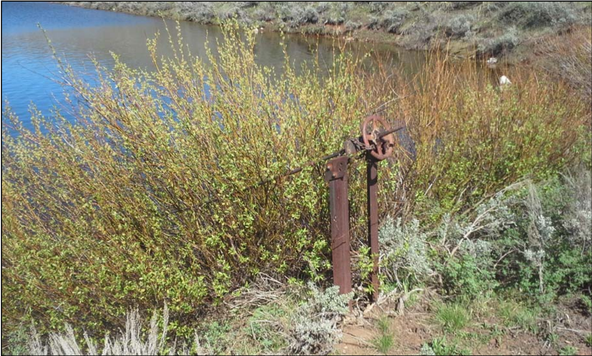
Figure 3.5-5 Davis No. 2 Reservoir outlet control.
