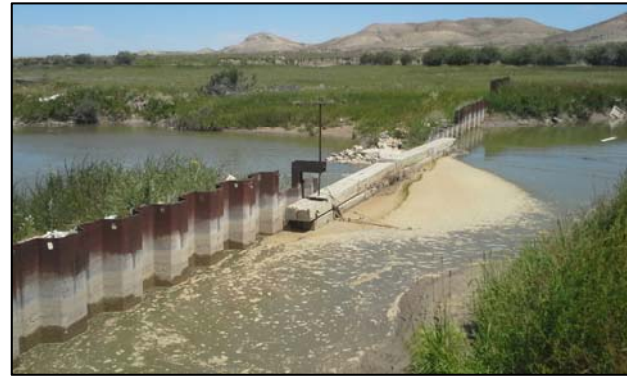
Figure 3.2-8 Existing Philbrick and Johnson Ditch Diversion.
