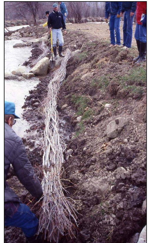
Figure 4.7-4 Stream Stabilization Measure: Willow Fascine Installation.
