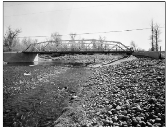
Figure 3.3-25 Bridge over Blacks Fork near Fort Bridger, WY (Source: SHPO, 2014).
