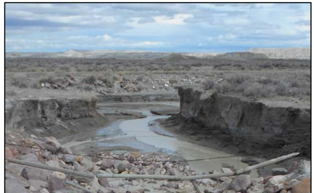
Figure 3.6-9 Severe channel degradation on Sage Creek.
