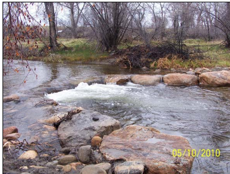
Figure 4.7-2 Stream Stabilization Structure: Rock Vortex Weir.
