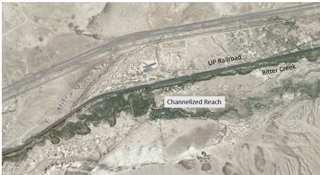
Figure 4.2-31 Stream Channelization: Bitter Creek at UP Railroad.
