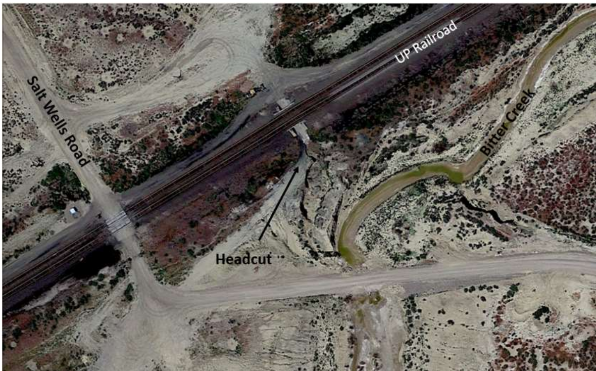
Figure 4.2-33 Headcut Location: Tributary to Bitter Creek.
