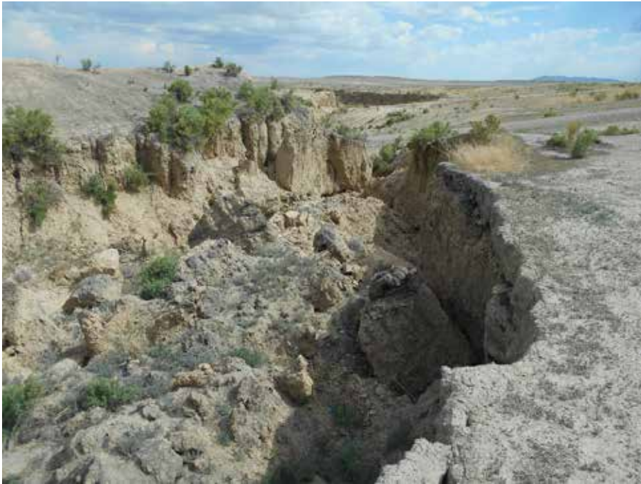
Active Headcut at UPRR
