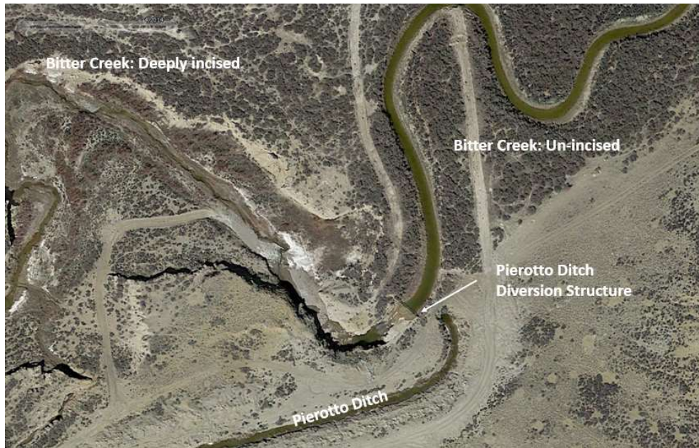
Figure 4.2-35 Pierotto Ditch Diversion Structure.
