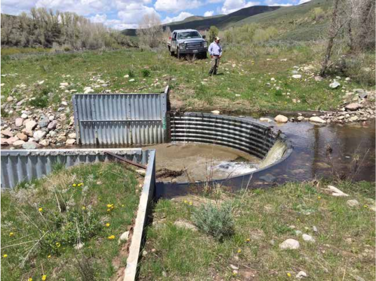
Typical Fish Barrier
