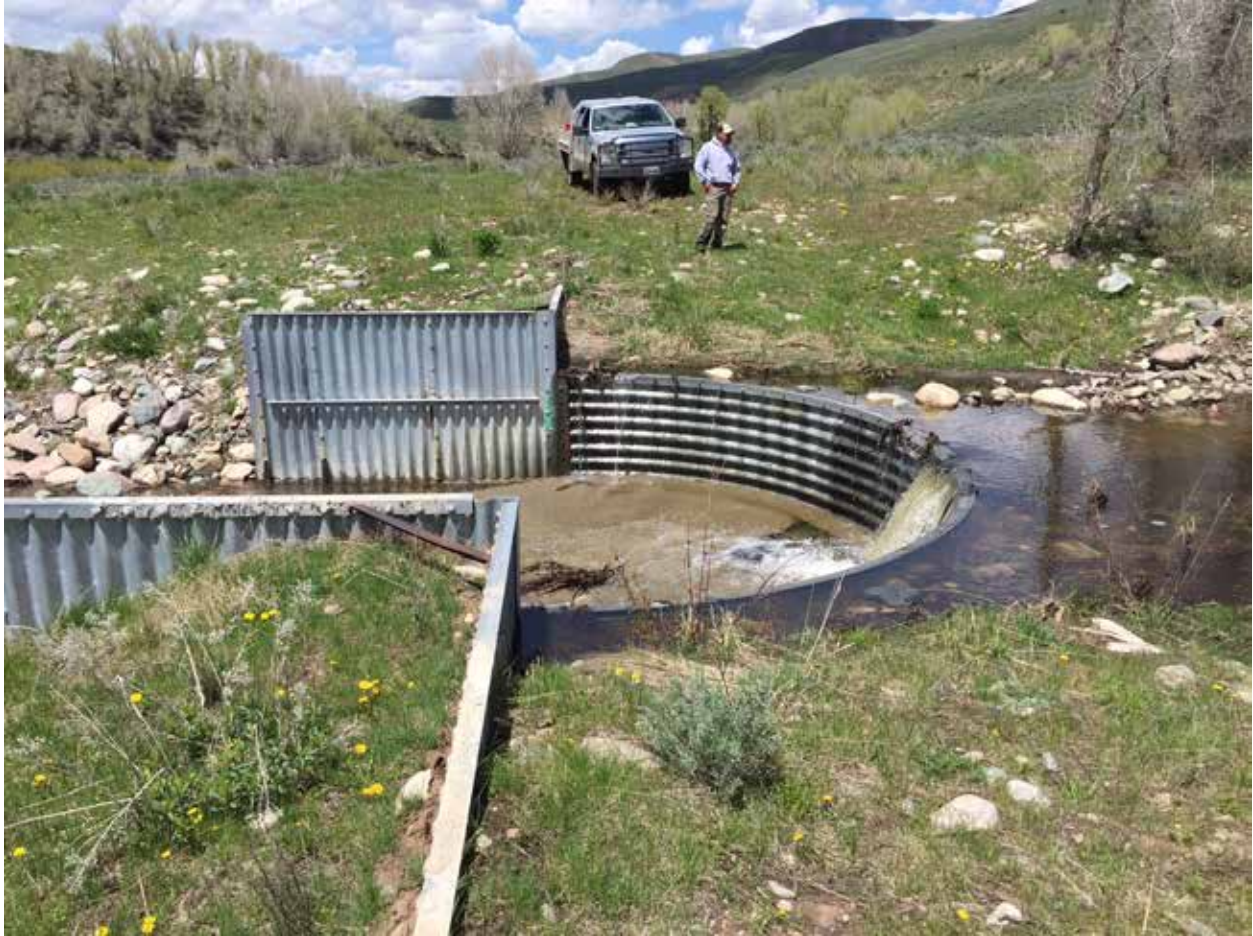
Typical Fish Barrier
