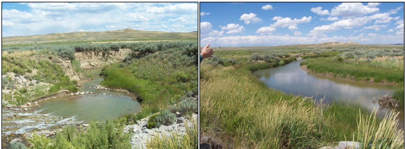
Figure 6.5-3 Channel Gradient Restoration Feature on Muddy Creek near Baggs, WY. Photo on left is viewed Downstream from the Dam at Incised Channel. Photo on the right is viewed Upstream at Restored Gradient.
