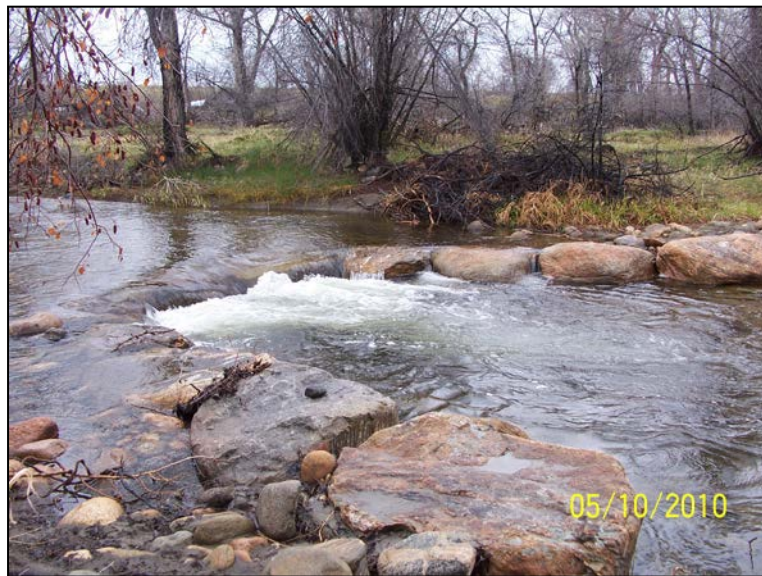
Figure 6.5-2 Stream Stabilization Structure: Rock Vortex Weir.
