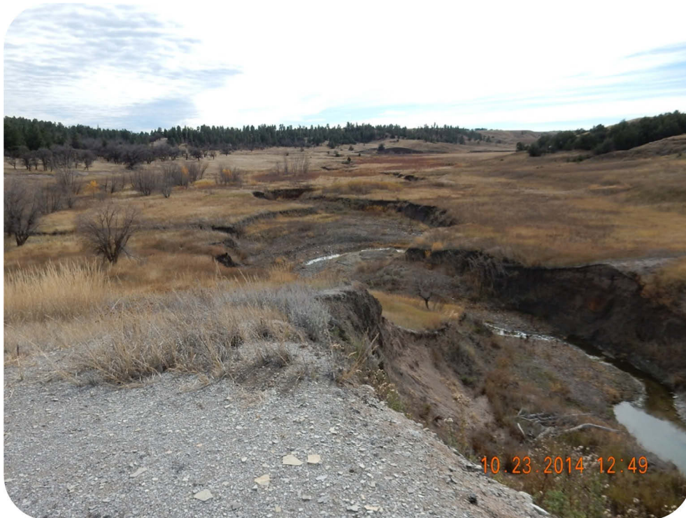
Figure 4.8. A View Looking Upstream From Pine (Deep) Creek Reservoir’s Breached Dam.
