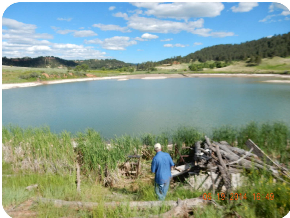
Figure 4.5. A View of Driskill #1 Reservoir's Inlet Structure.
