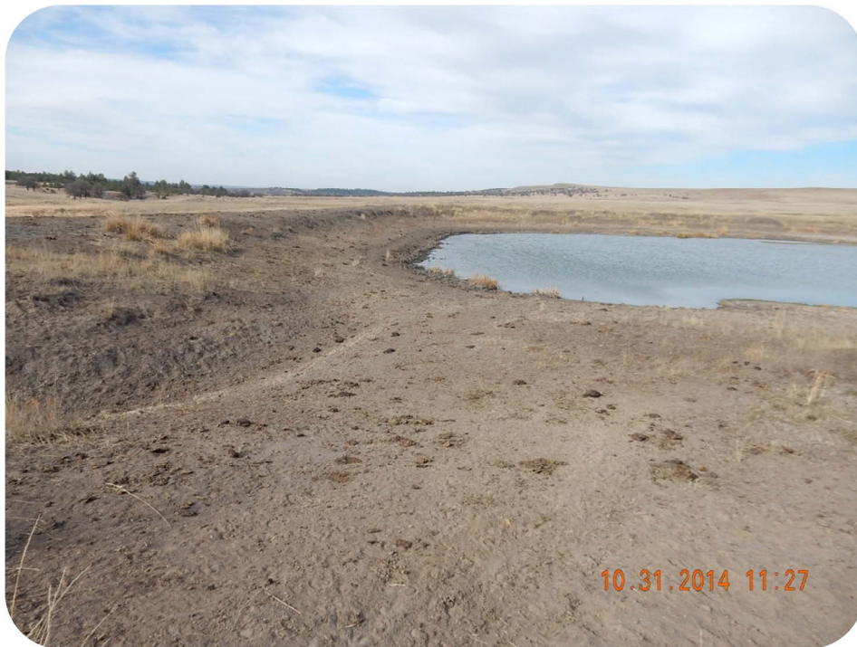
Figure 4.16. A View of Newland #4 Reservoir Dam.
