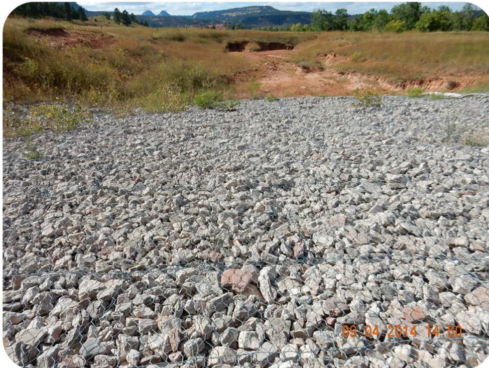
Figure 4.6. A View of Driskill #1 Reservoir's Emergency Spillway.
