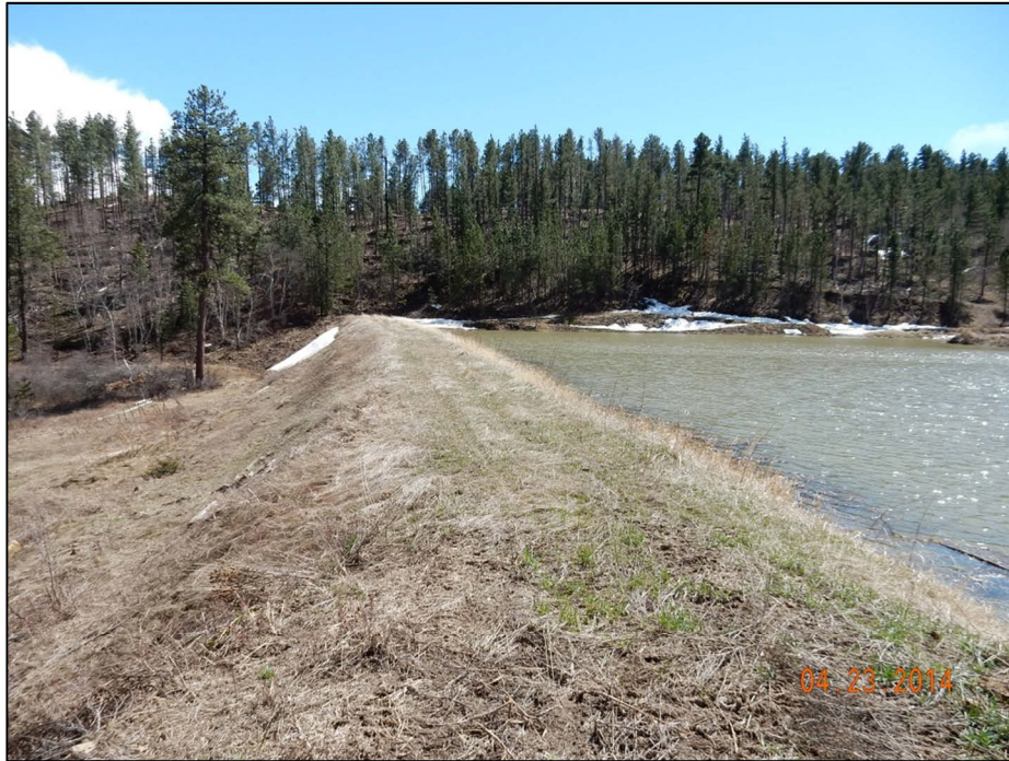
Figure 4.14. A view of Hemler Dam on Sunset Reservoir on April 23, 2014.
