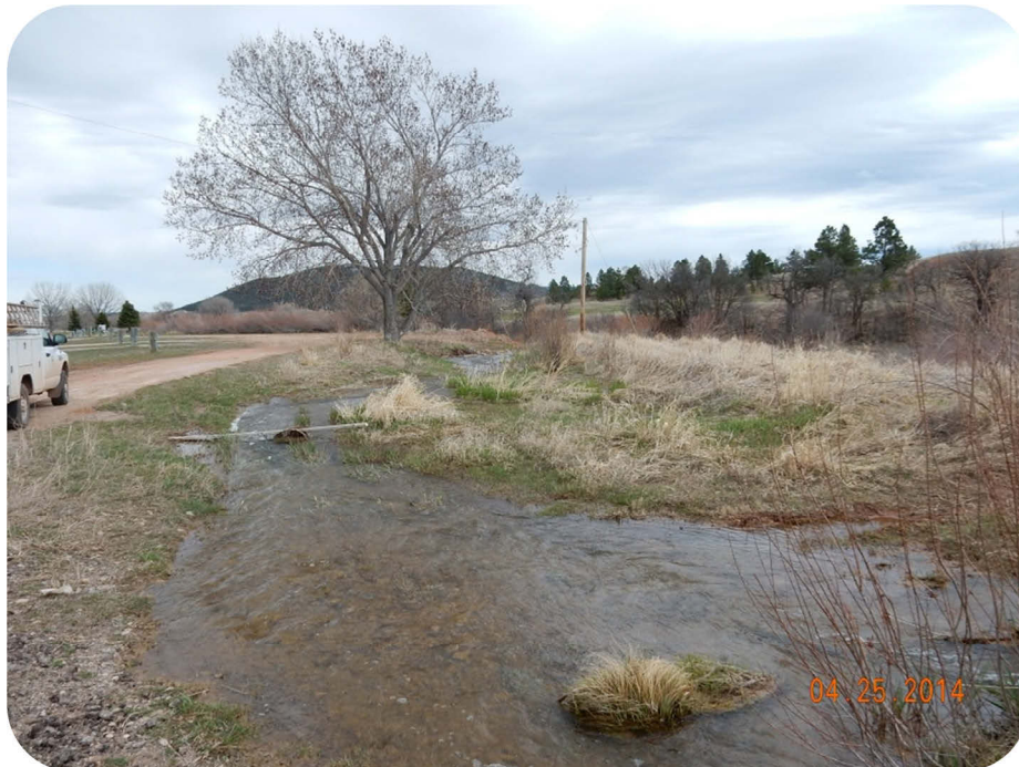
Figure 4.12. A view of Washington Memorial Reservoir's Emergency Spillway.
