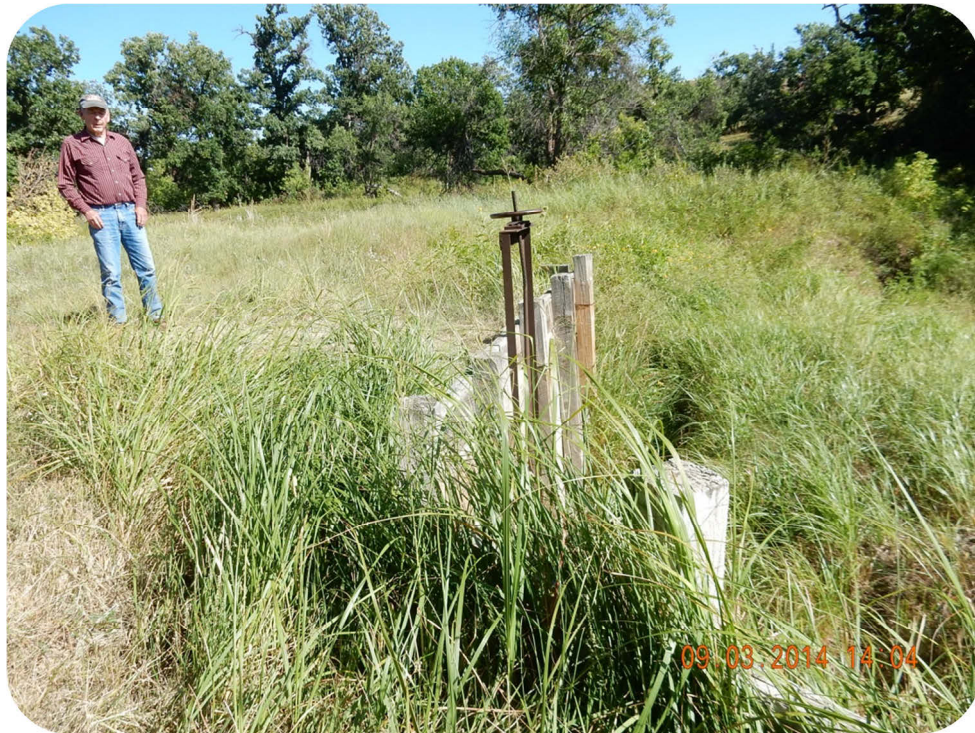
Figure 4.1. Diversion/Headgate Structure on North Redwater Creek.
