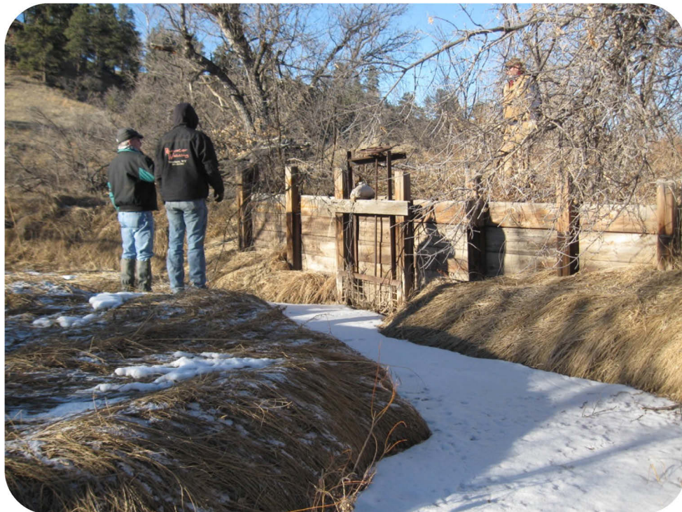
Figure 4.2. Diversion/Headgate Structure on South Redwater Creek.
