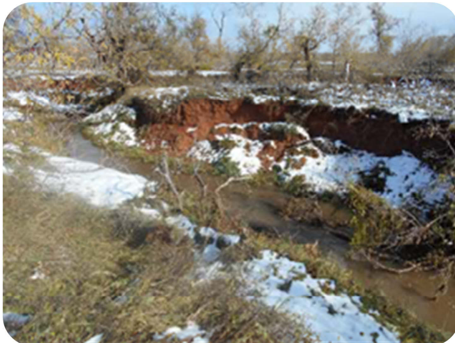
Figure 3.27. Evidence of Channel Widening of Redwater Creek.
