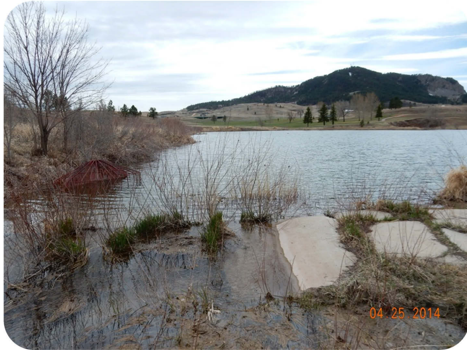
Figure 4.11. A View of Washington Memorial Reservoir's Inlet Structure and Emergency Spillway.
