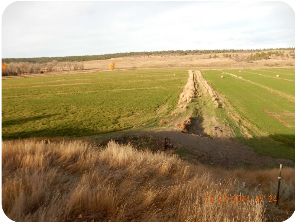
Figure 4-3. Headgate Structure on Lateral Ditch on Oak Creek.
