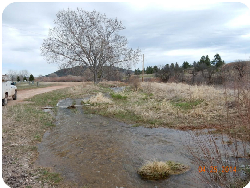
Figure 4-83. A View of Washington Memorial Reservoir's Emergency Spillway.
