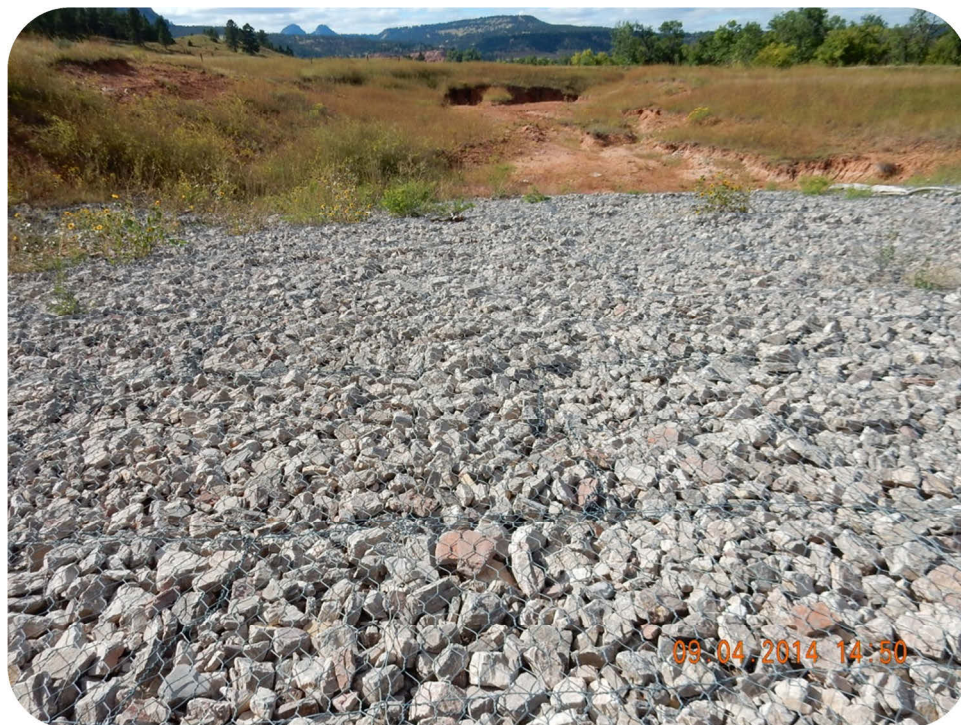
Figure 4-80. A View of Driskill #1 Reservoir's Emergency Spillway.
