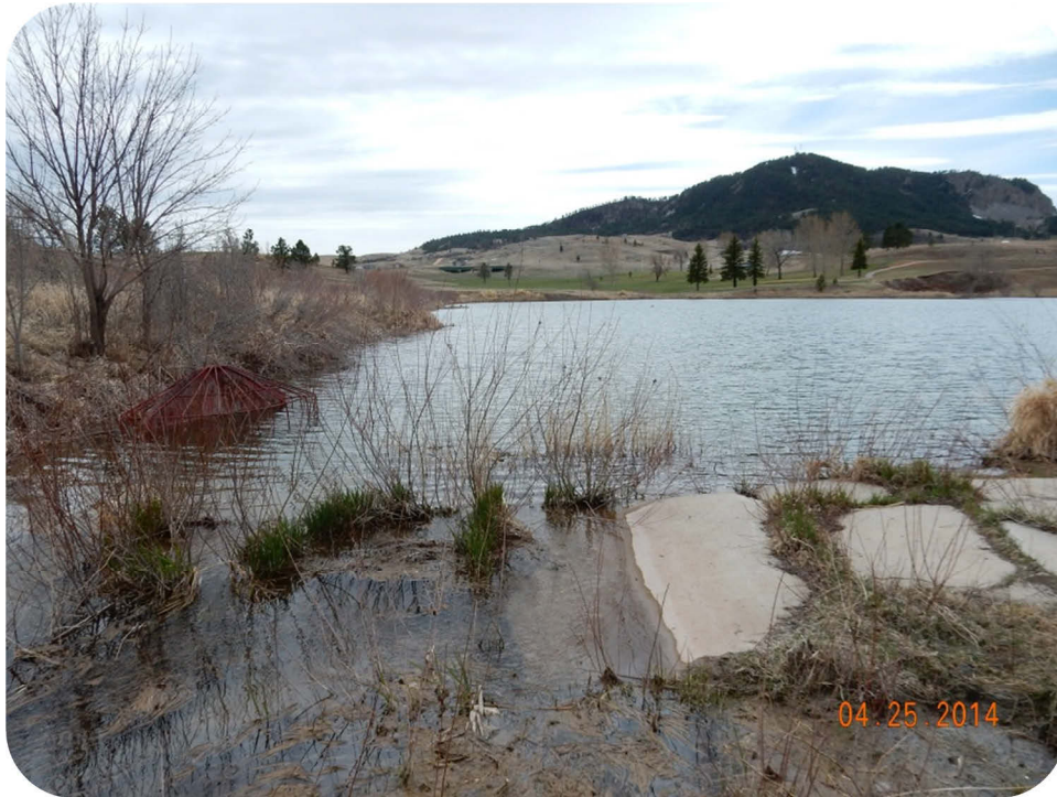
Figure 4-82. A View of Washington Memorial Reservoir's Inlet Structure and Emergency Spillway.
