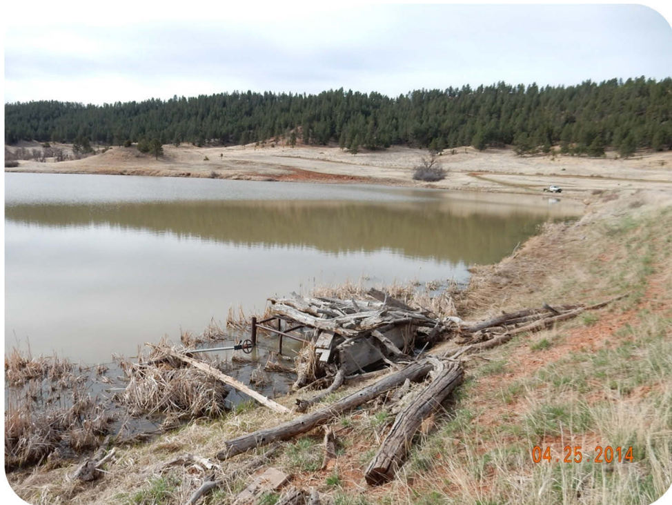
Figure 4-2. Outlet and Diversion Structure at Driskill #1 Reservoir on Lytle Creek.
