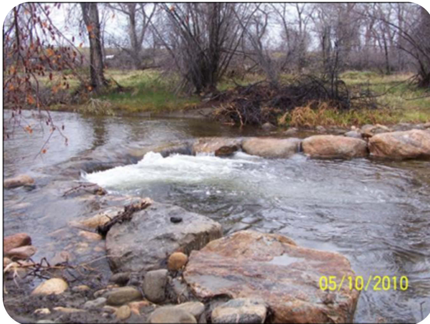
Figure 4-102. Stream Stabilization Structure: Rock Vortex Weir.
