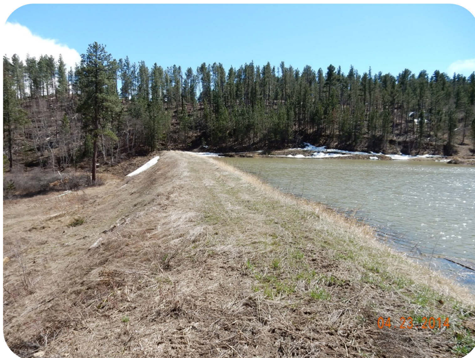
Figure 4-99. A View of Hemler Dam on Sunset Reservoir on April 23, 2014.
