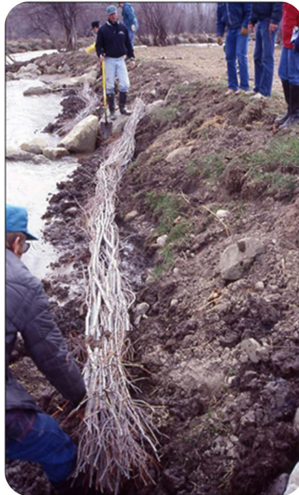
Figure 4-104. Willow Fascine Installation.
