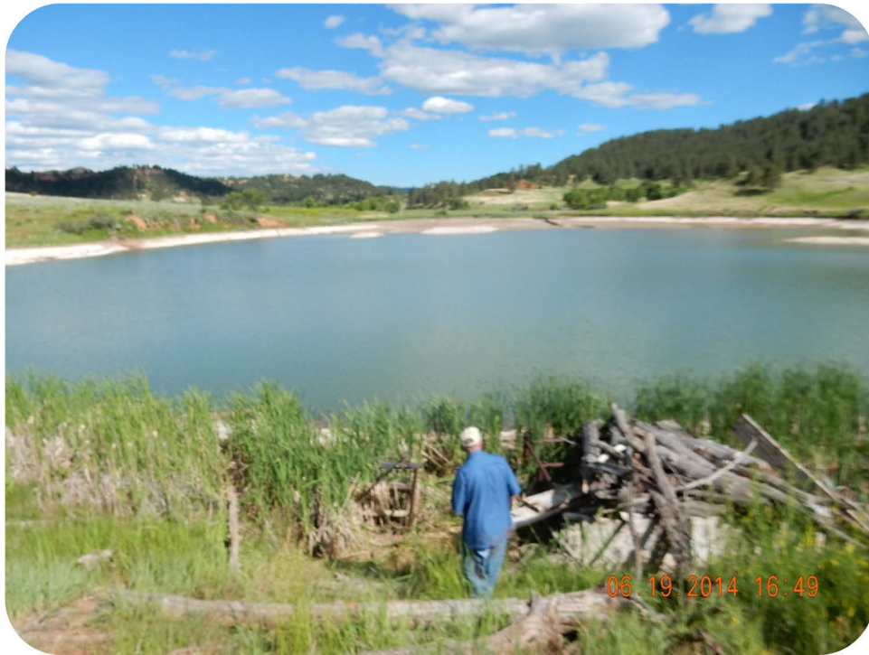
Figure 4-79. A View of Driskill #1 Reservoir's Inlet Structure.
