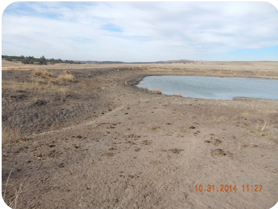
Figure 4-93. A View of Newland #4 Reservoir Dam.
