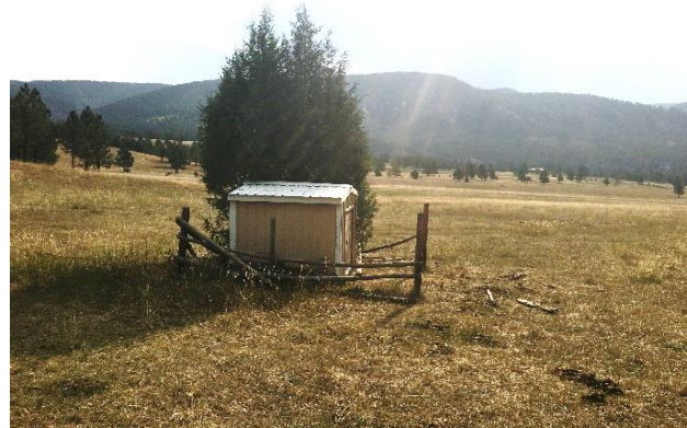
Photo 27 Existing wellhouse (LWW-21.2).
