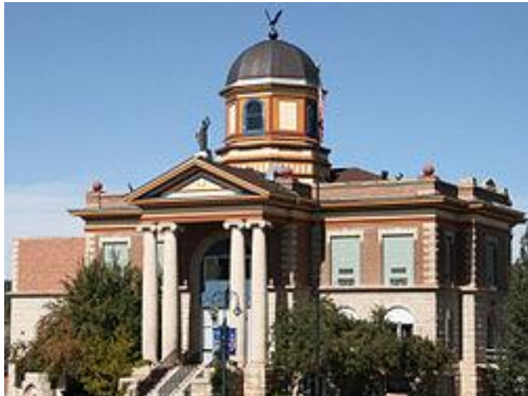
Photo 20 Weston County Courthouse.
