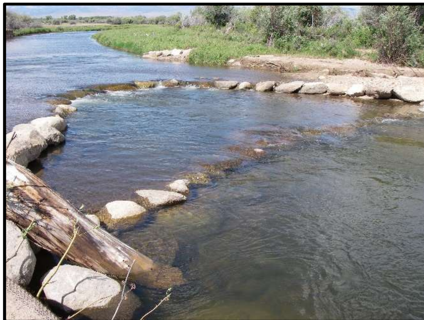
Photo 4.3.2.2 Instream treatment example: rock cross vanes.
