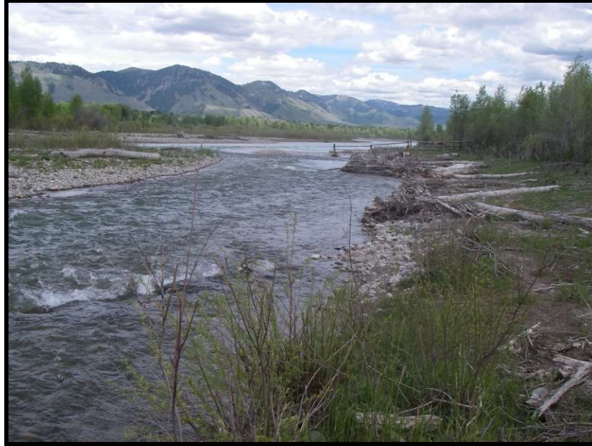
Photo 4.3.2.5 Instream treatment example: root wad revetment and rock barb.
