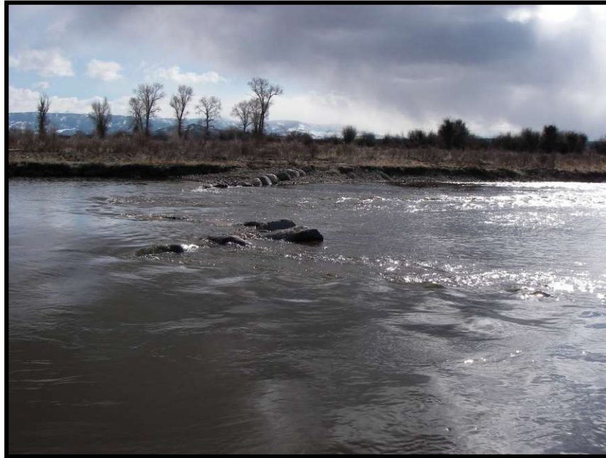
Photo 4.3.2.1 Instream treatment example: W-weir.
