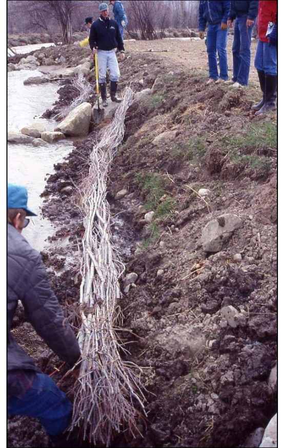
Figure 4.7-4 Stream Stabilization Measure: Willow Fascine Installation.
