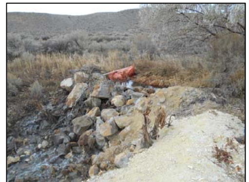
Figure 3.8-1 Dry Creek No. 2 Ditch Diversion.
