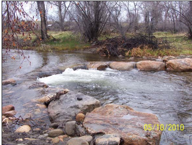
Figure 4.7-2 Stream Stabilization Structure: Rock Vortex Weir.
