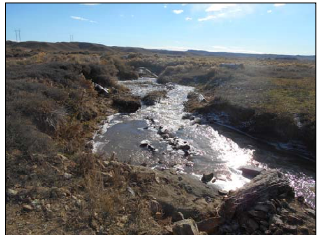
Figure 3.8-3 Channel Degradation in vicinity of Moore Ditch Diversion.
