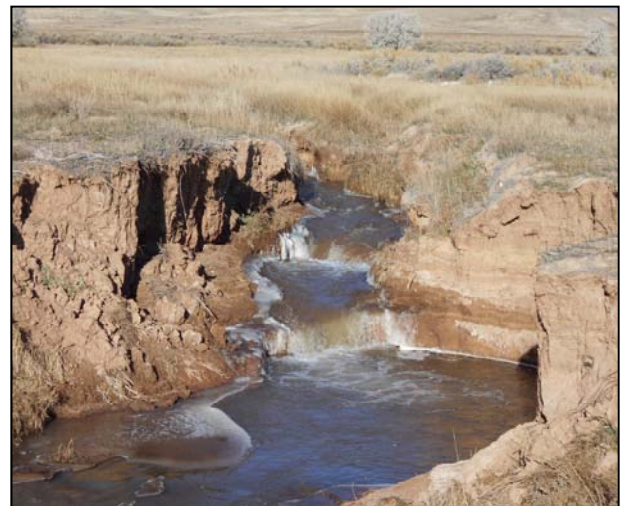
Figure 3.6-10 Active headcut located on Bridger Creek.
