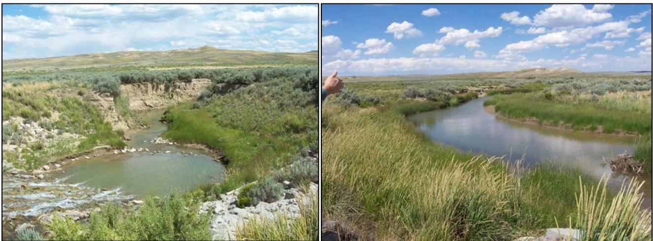
Figure 4.7-3 Channel Gradient Restoration Feature on Muddy Creek near Baggs, WY. Photo on left is viewed downstream from the dam at incised channel. Photo on the right is viewed upstream at restored gradient.
