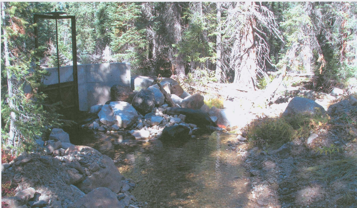
Figure 3. Point of diversion for the Carlson Auxiliary Ditch on Carlson Creek
