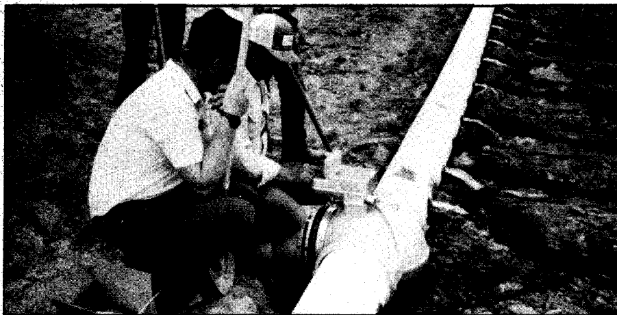
John Brenner (left), USDA SCS Area One project engineer in Riverton, watches Hurley Dockham, an area farmer, program the surge valve's solar-powered computer. Dockham is programming the timing of the irrigation surges.
